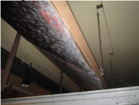
Damaged Baffles
