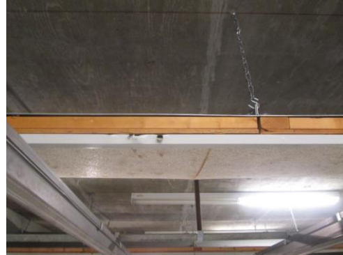
Steel baffles with plywood
