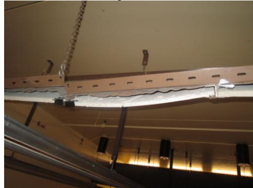
Back side of damaged baffles
