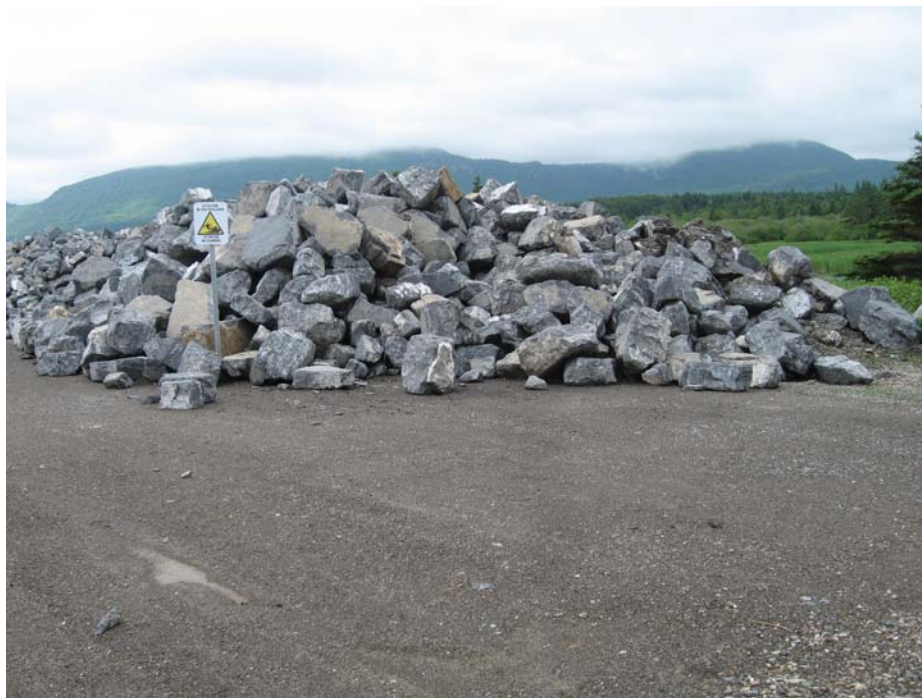
Photo 9 - Stone size 300 to 450 mm (quantity 3420 mt) provided by PWGSC. It is situated along the coast road.
