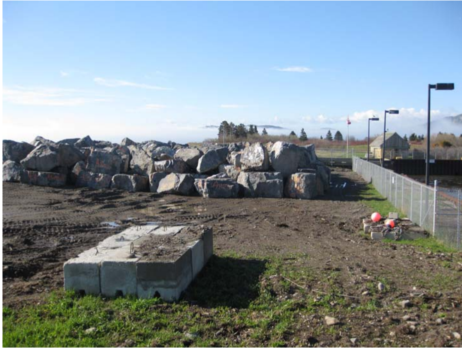
Photo 7 - Stone size 8-12 mt (quantity 3200 mt) provided by PWGSC. It is located near the harbor.
