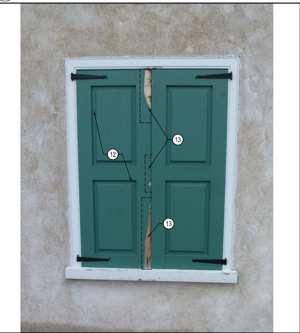
7 PHOTO - WINDOW 110 - SHUTTERS TO REPAIR N.T.S.
