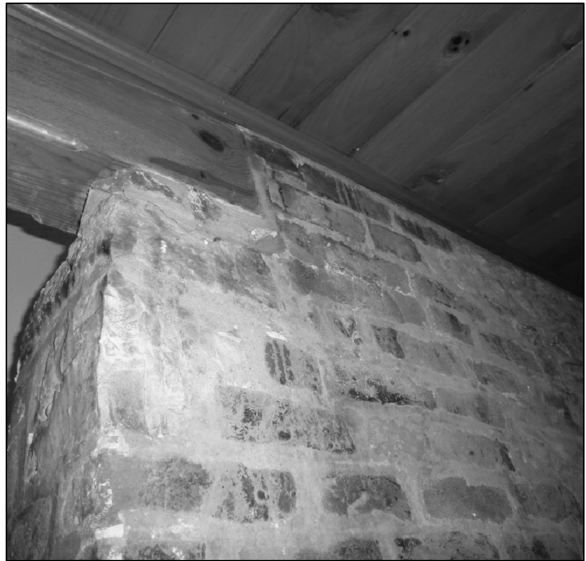
7 PHOTO - BRICK AND WOOD LINTEL A500 N.T.S.
