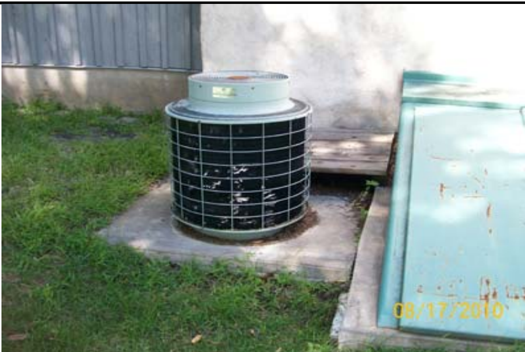
Photo No. 18: Heat pump, south side of building, potentially contains ODS.
