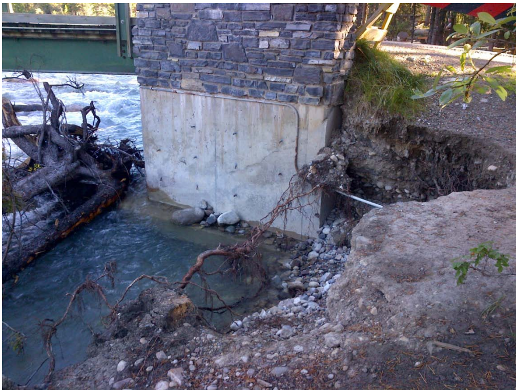
Figure 2. Scouring of bridge abutment
