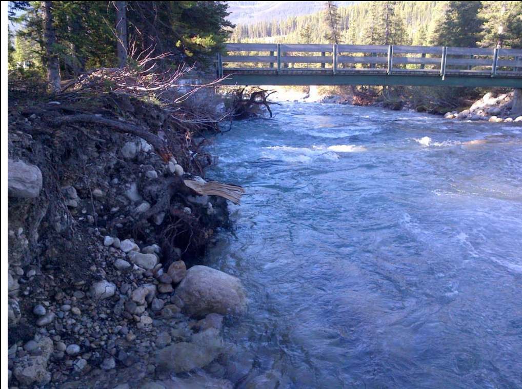
Figure 1. Bank erosion upstream of footbridge
