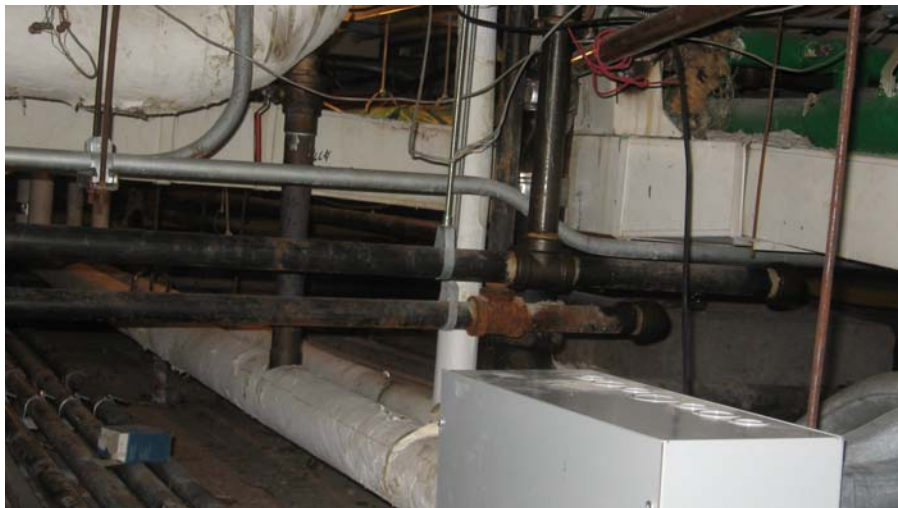
Photo 4: MHK Crawspace White Canvas Jacketed Supply Air Ducting.
