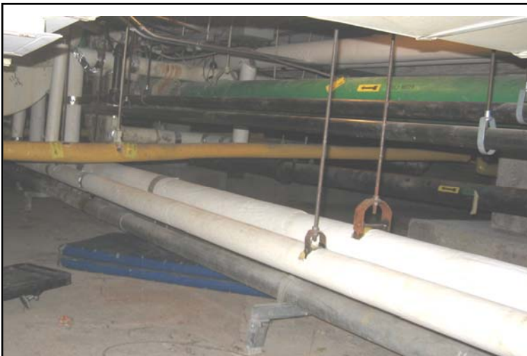
Photo 5 & 6: MHL Crawlspace Yellow and Green Canvas Jacketed Piping. Note joist hangers are free of plaster.
