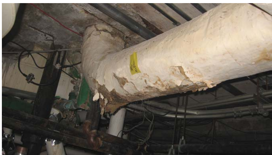
Photo 8: MHL Crawlspace White Canvas Jacketed Supply Air Ducting.
