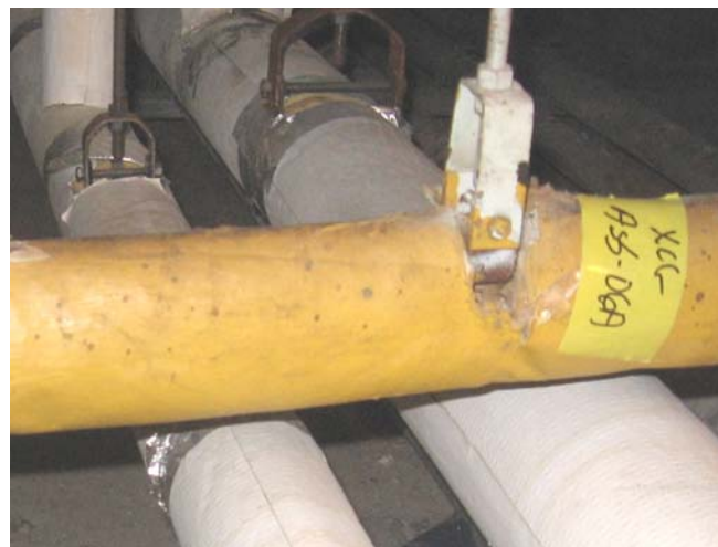
Photo 5 & 6: MHL Crawlspace Yellow and Green Canvas Jacketed Piping. Note joist hangers are free of plaster.
