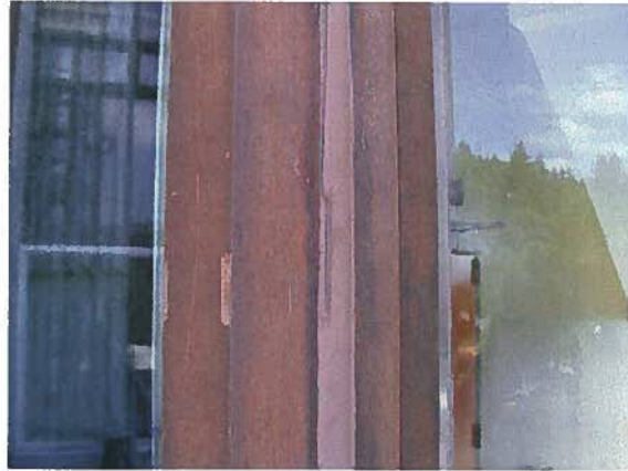
Photo 2: Red Exterior Window Mastic (none detected)
