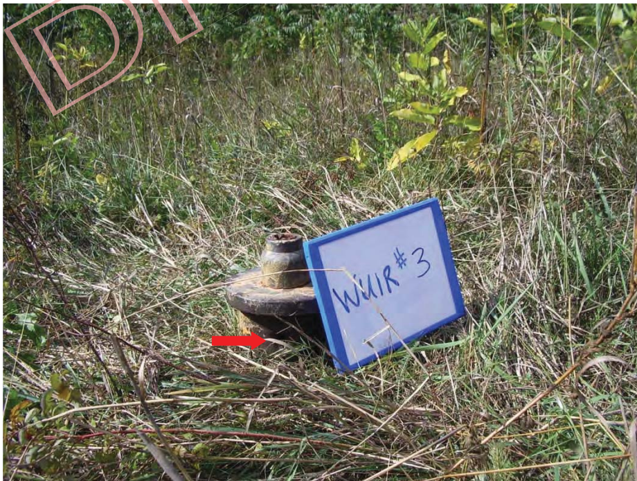
Photograph 8: Well 3 – Looking north. Well is sealed with a metal plate and casing is perforated (red arrow). Photograph taken September 13, 2012. See accompanying text for description of the well and site conditions.
