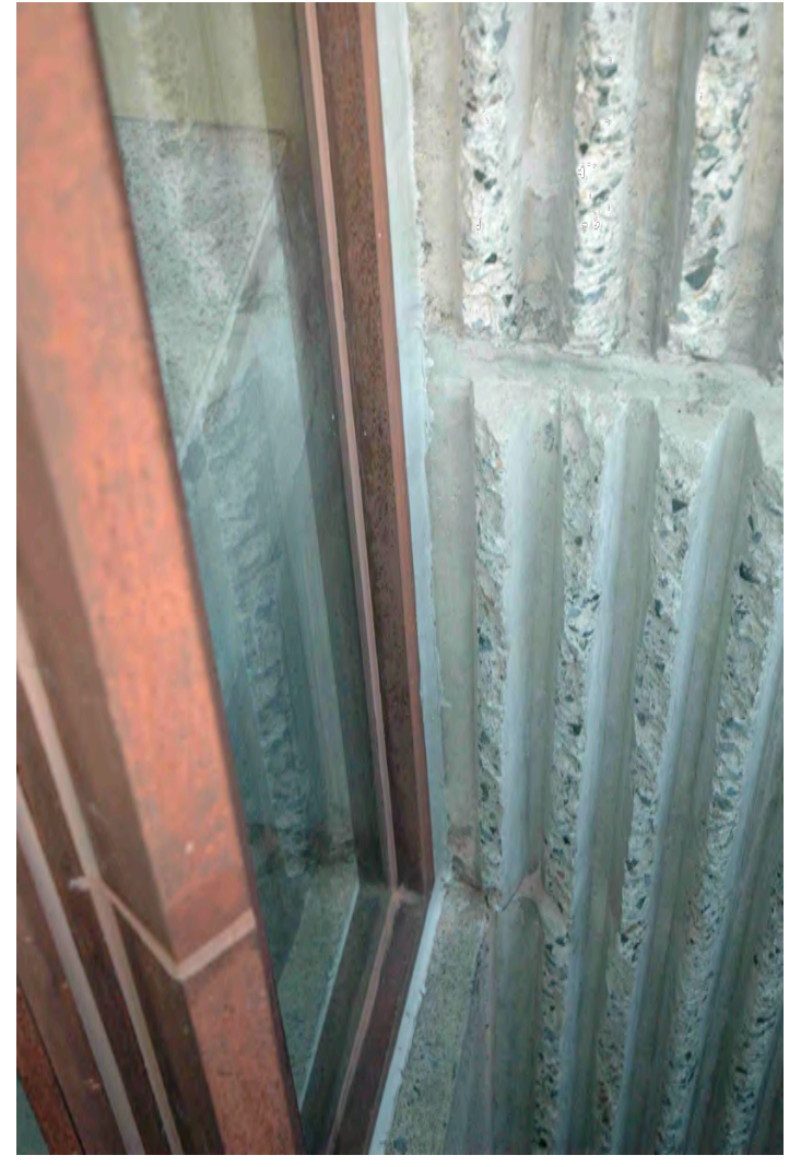
(E) STEEL FRAME ON CURB @ WALL
