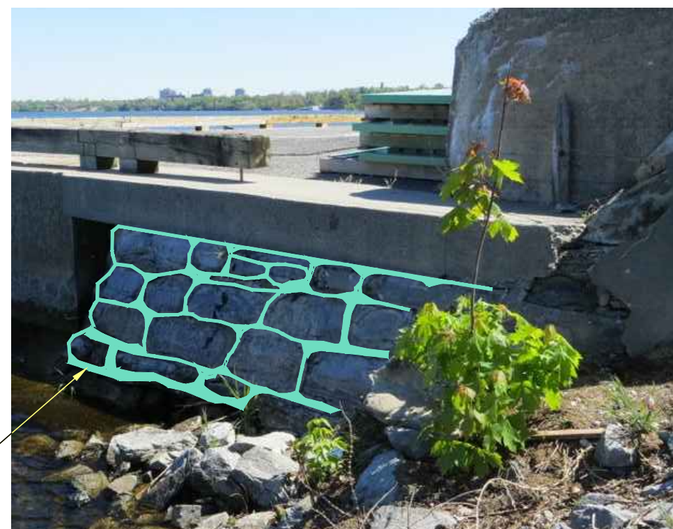
WEST END OF WHARF - PHOTO #3 STONE MASONRY REPOINTING N.T.S.
