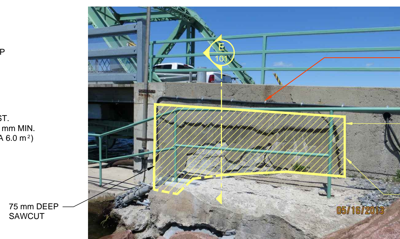
SOUTHEAST WING WALL - CONCRETE REPAIRS - PHOTO#7 N.T.S.
