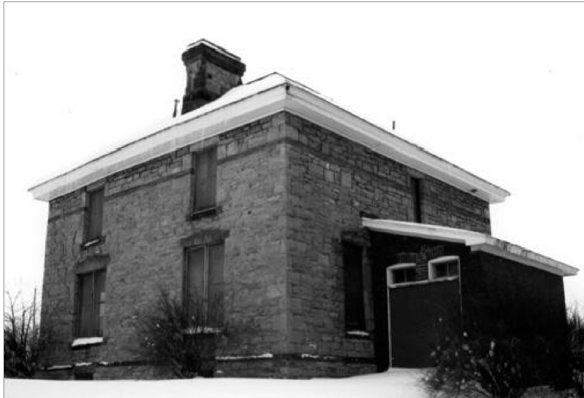
VUE DU NORD-EST / NORTH-EAST VIEW
