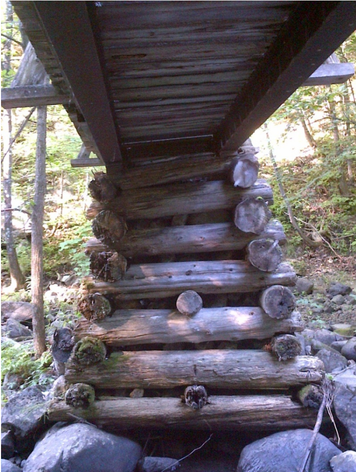
Figs 3 and 4 (facing W. then N.) show failure of centre pier
