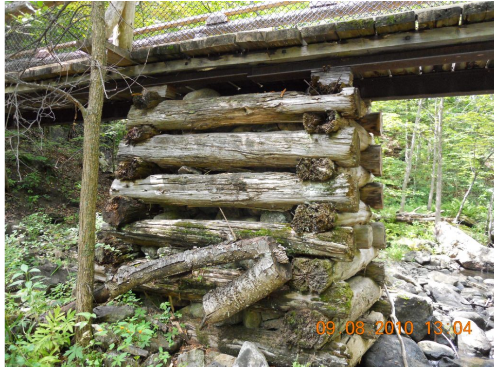
Figs 3 and 4 (facing W. then N.) show failure of centre pier
