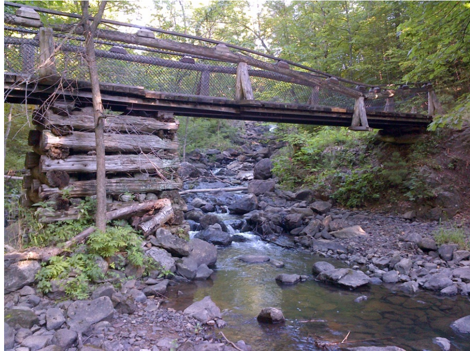
Figs 1 and 2 (facing W. then N.) shows handrail failure and deck warping
