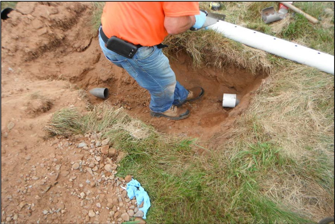
Photo 4 – Septic line replacement at TH209
