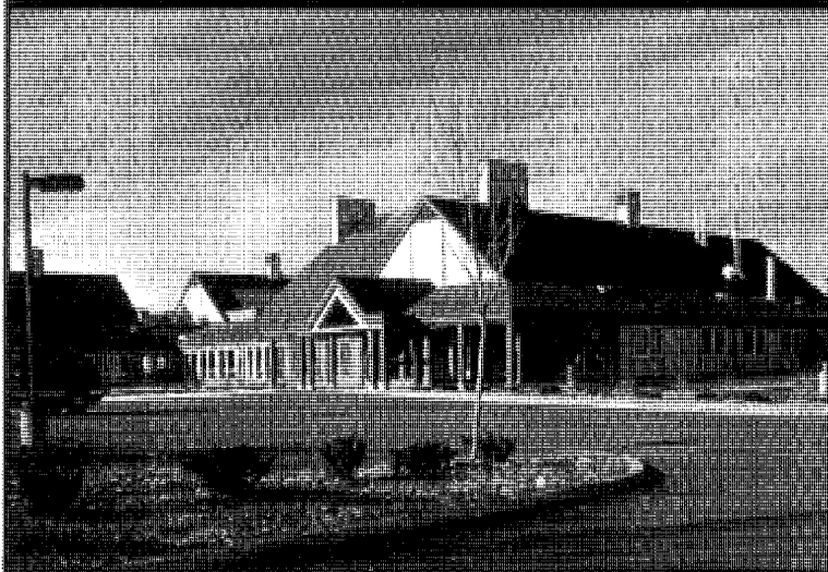
Photo 119: Each of the three houses in this complex is joined by a large common area
