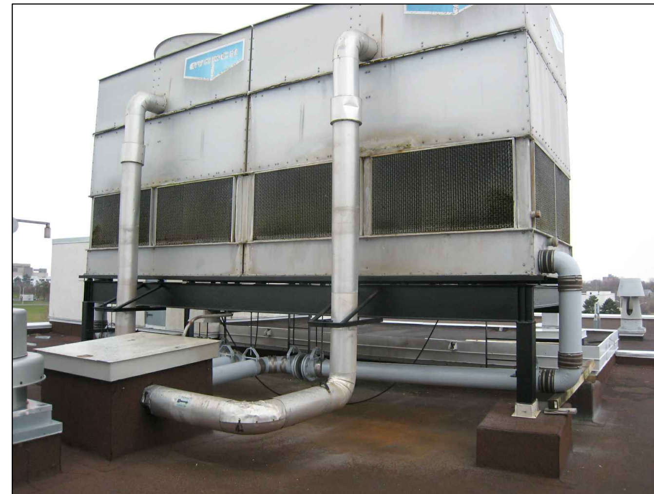
1 BACK VIEW OF EXISTING COOLING TOWER M02 SCALE = NA
