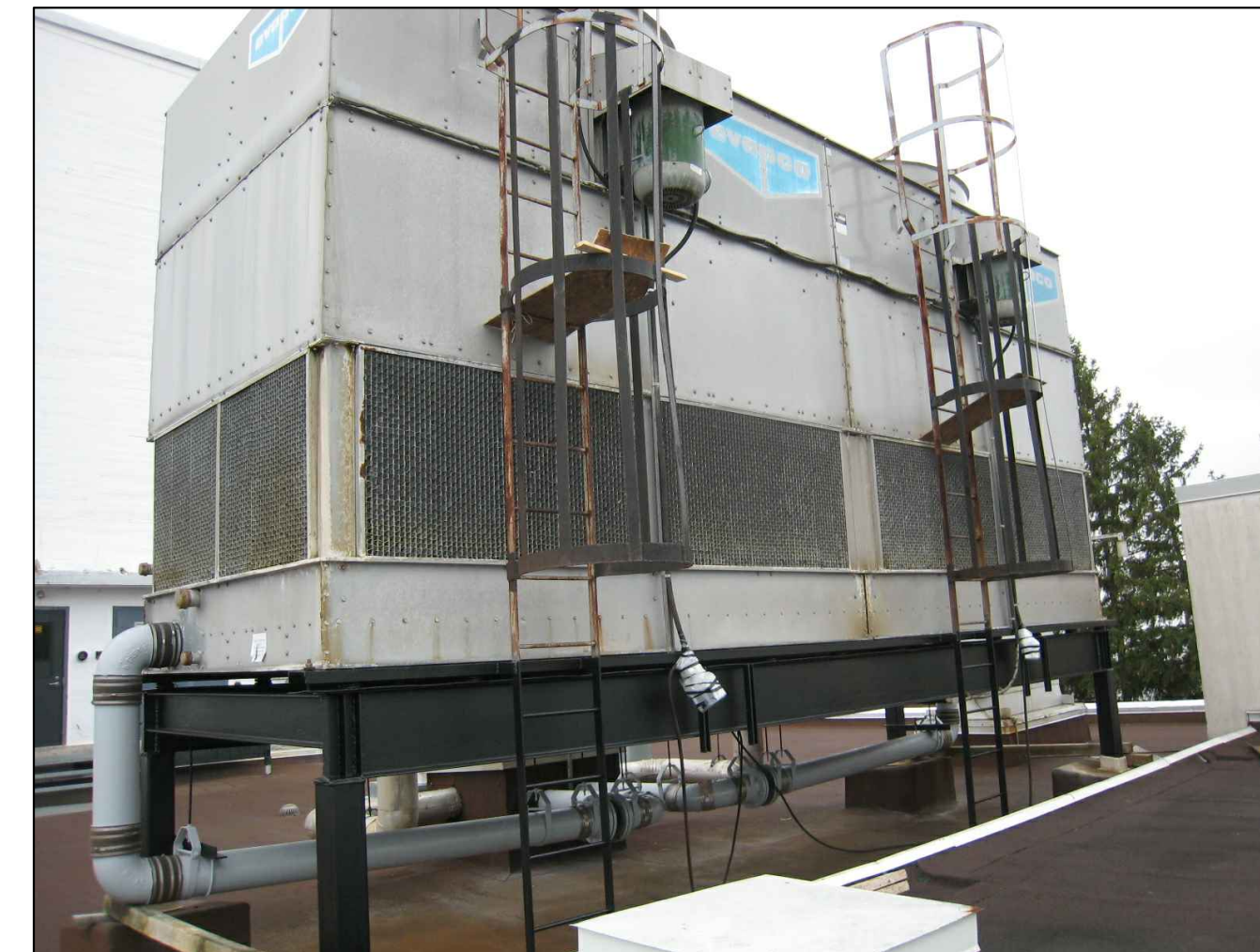
2 FRONT VIEW OF EXISTING COOLING TOWER M02 SCALE = NA
