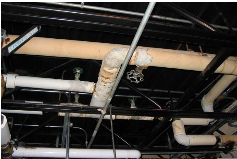
PHOTO 1: WW16 – Room 201 – Pipe elbows in the room noted to be in good condition. The elbows contained more than 75% chrysotile asbestos
