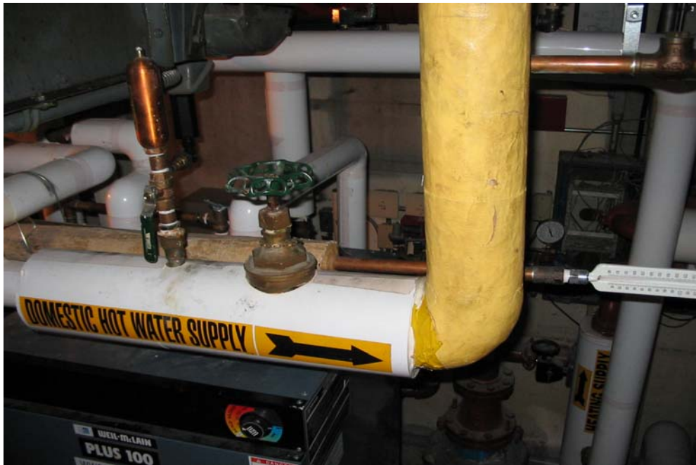
PHOTO 1: WW05 – Room 109 – An example of a pipe elbow that, along with other elbows and T-joints, contained between 50 and 75% chrysotile asbestos.
