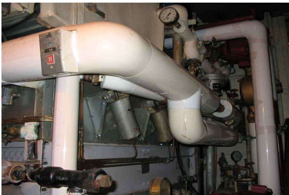
PHOTO 1: WW06 – Room 114 – A view of the pipe elbows and T-joints that contained between 25 and 50% chrysotile asbestos.
