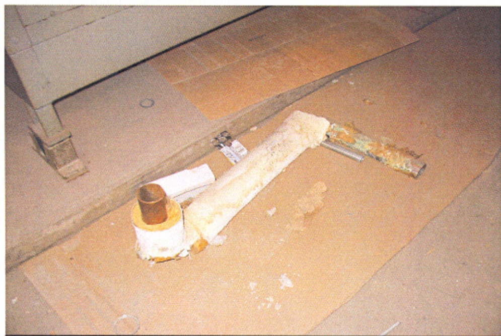
PHOTO 2: WW18 – Room 201 – A disassembled pipe elbow that contained greater than 75% chrysotile asbestos. There were other elbows and joints that were noted to be in fair or poor condition.
