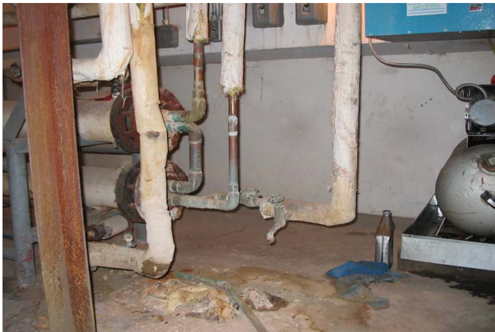
PHOTO 2: WW12 – Room 209 – Another example of the pipe elbows and joints in poor condition. They were found to contain between 50 and 75 % chrysotile.
