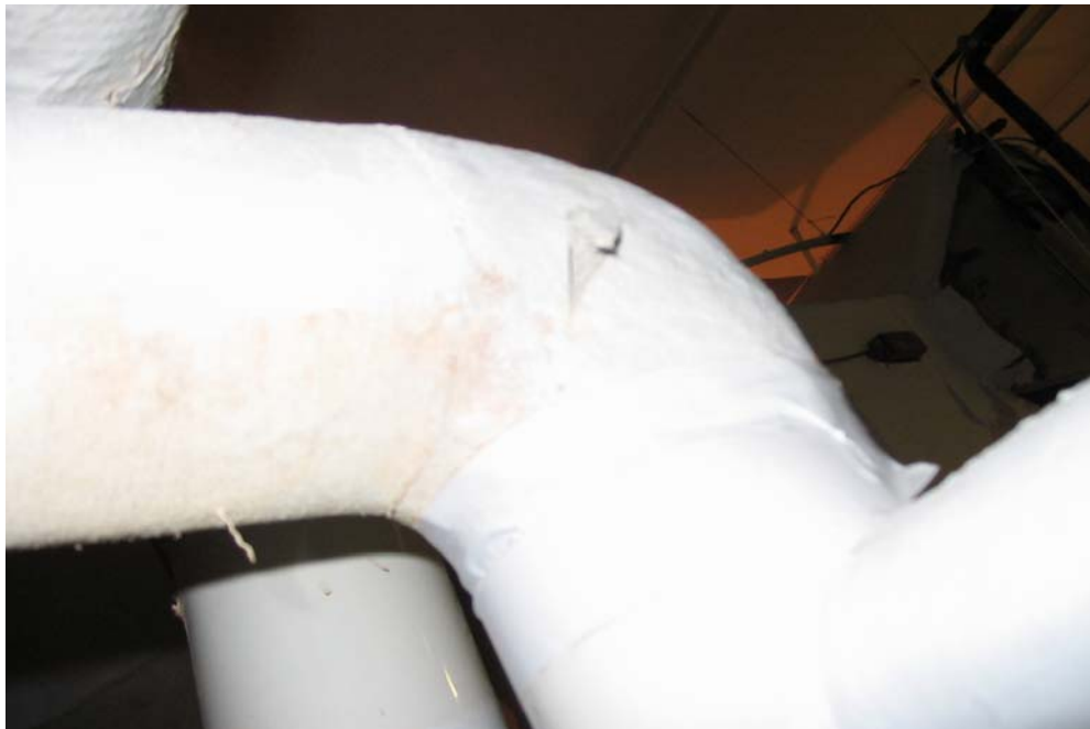
PHOTO 1: WW03 – Room 130 – This pipe elbow was sampled and found to contain between 50 and 75% chrysotile asbestos.
