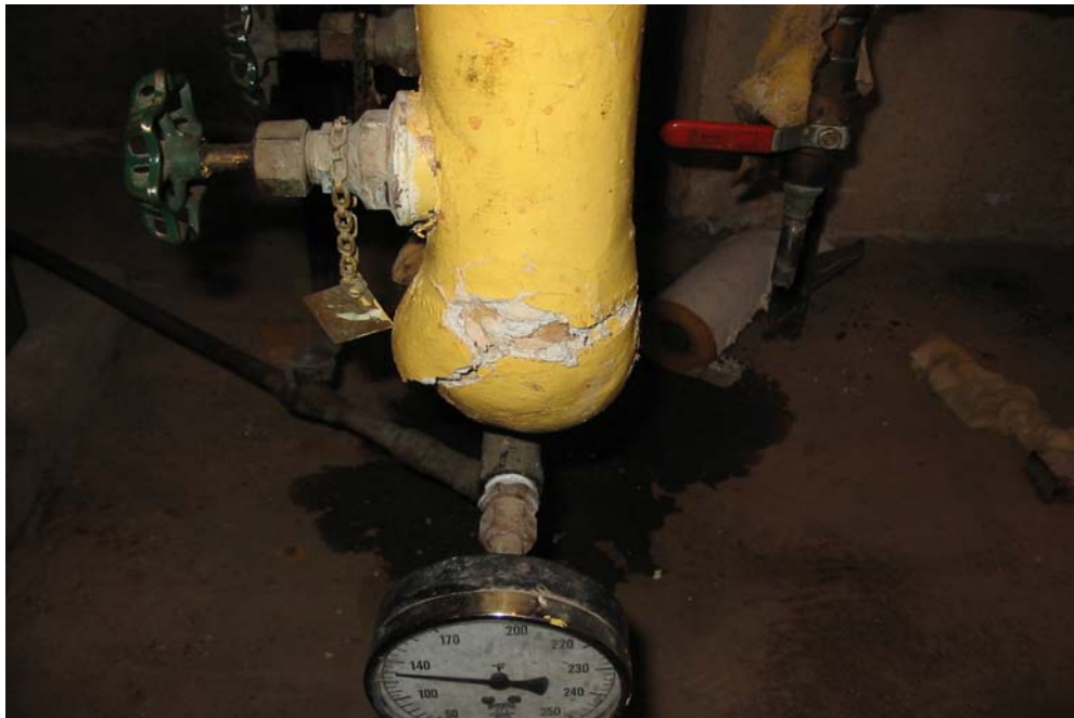
PHOTO 1: WW07 – Room 139 – An example of the many pipe elbows that were found in the room. This one was found to contain between 50 and 75% chrysotile asbestos and is in poor condition.
