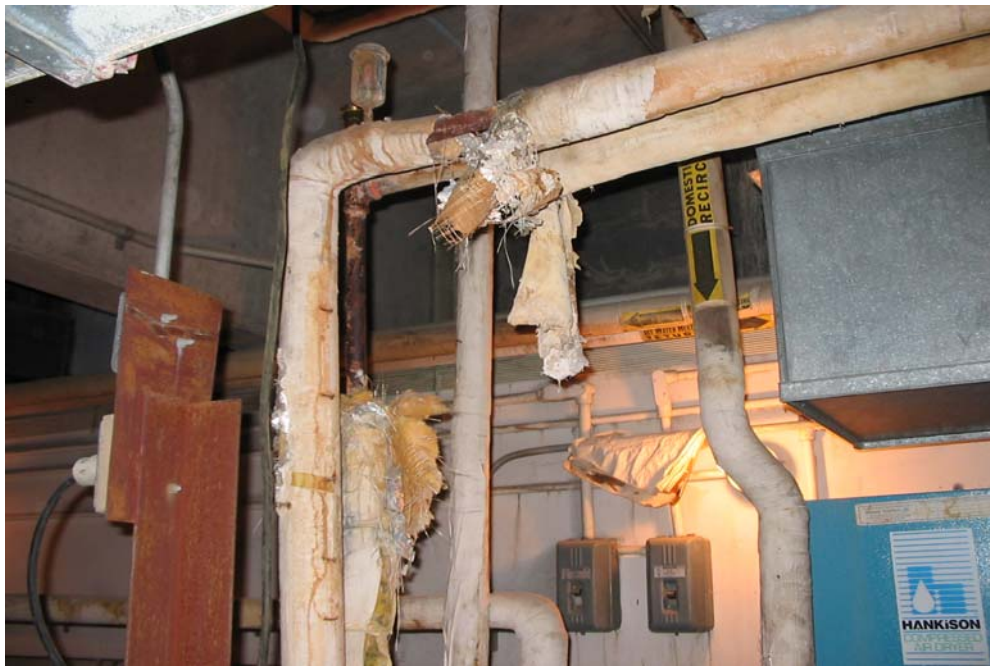
PHOTO 1: WW12 – Room 209 – An example of the pipe elbows and joints in poor condition. They were found to contain between 50 and 75 % chrysotile.
