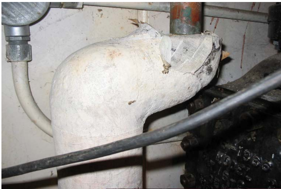
PHOTO 1: WW15 – Room 102 – A pipe elbow which, along with others, contained between 50 and 75% chrysotile asbestos. The elbow was noted to be in fair condition.
