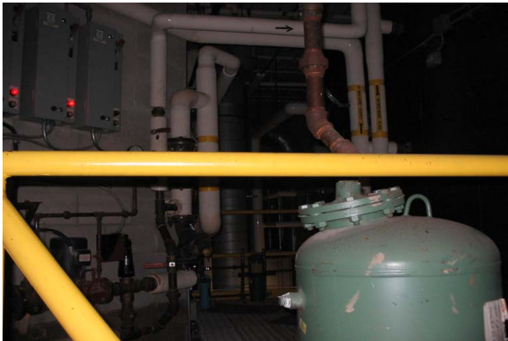
PHOTO 1: WW31 – Room M02 – Yellow railing paint that was found to contain a lead concentration of 10,052 ppm. The paint was noted to be in poor condition.
