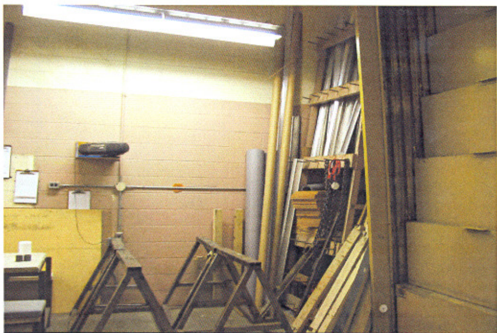
PHOTO 1: WW18 – Room 142 – Light brown paint on lower half of the wall was found to contain a lead concentration of 11,399 ppm. The paint was in fair condition.
