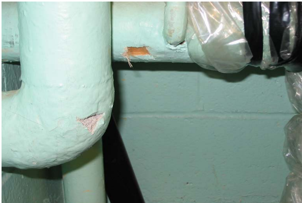
PHOTO 2: WW19 – Room 133 – A pipe elbow noted to be in good condition. The elbow contained between 50 and 75% chrysotile asbestos.
