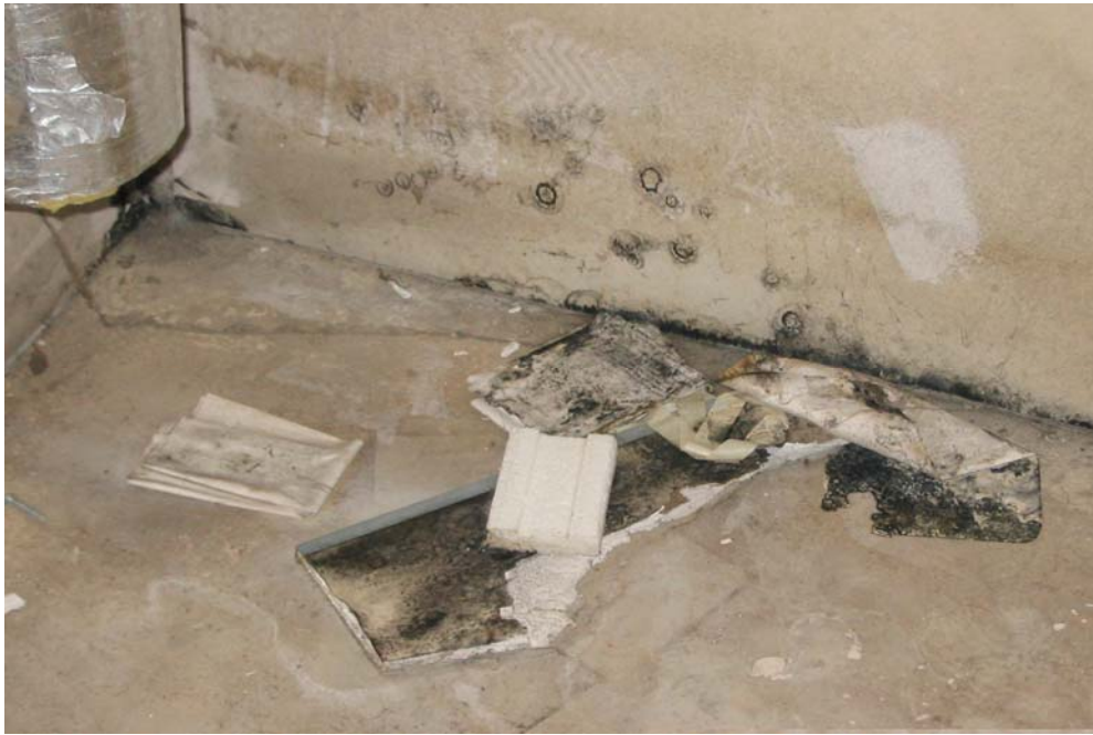
PHOTO 1: WW35– Room B01 – Water damage and mould growth observed in the basement of the building.
