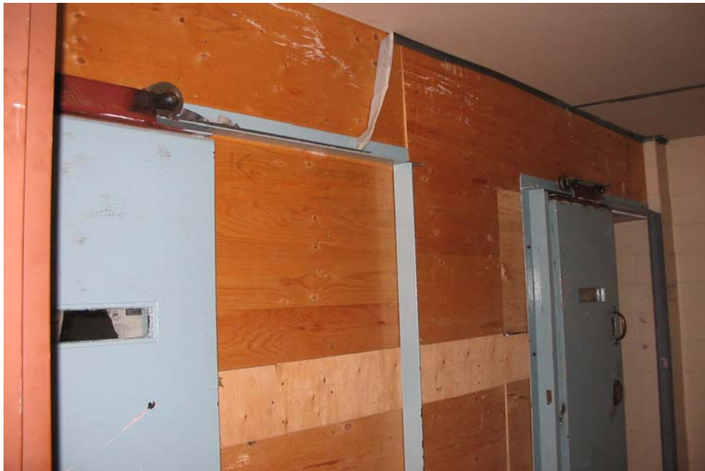
PHOTO 1: WA08 – Room 101 – The blue door paint on the mock cells were found to contain a lead concentration of 10,926 ppm.
