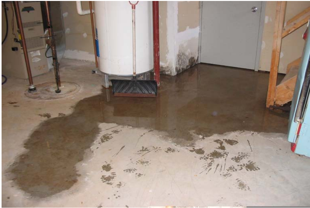
PHOTO 1: WW34 – Room B01 – Water leak and damage observed in the basement of the building. Also note mould growth on the wall to the right of the water boiler.
