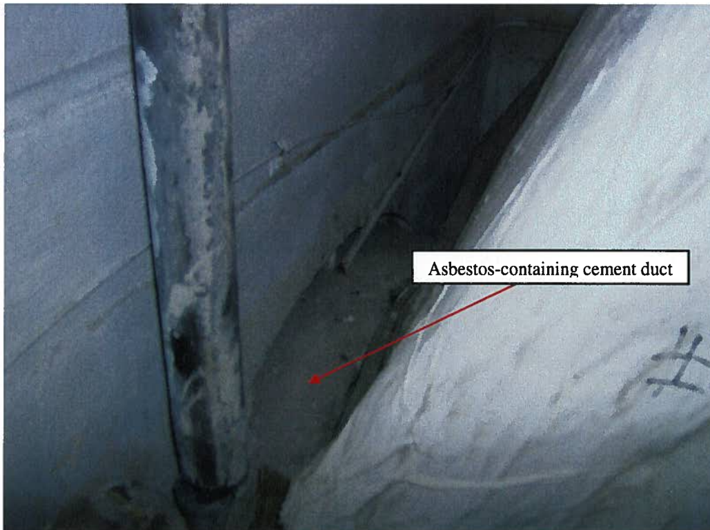
Photograph No. 1: Room 130 – Asbestos-containing cement duct penetrating north wall.
