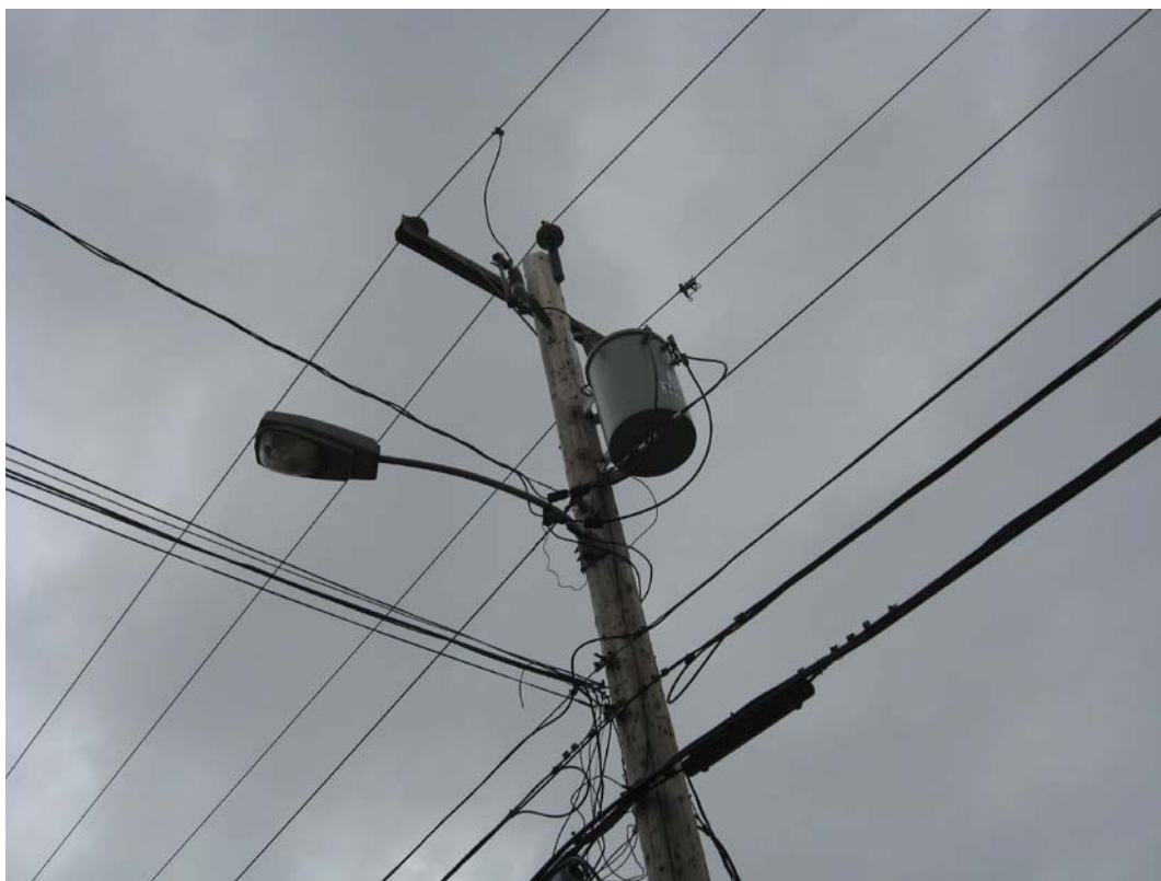
Photo 4: Pole-Mounted Transformer.
