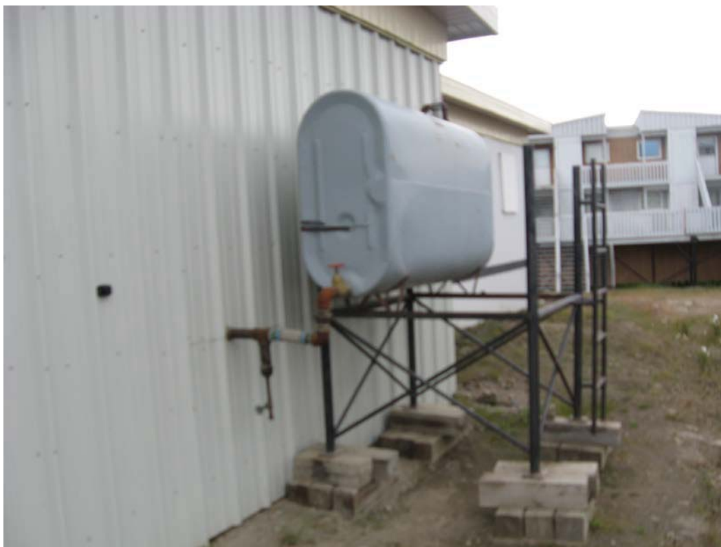
Photo 3: Furnace Oil AST.
