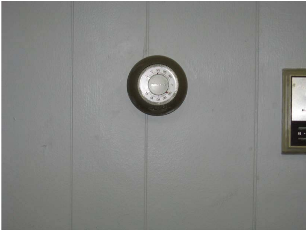
Photo 8: Mercury-Containing Thermostats.
