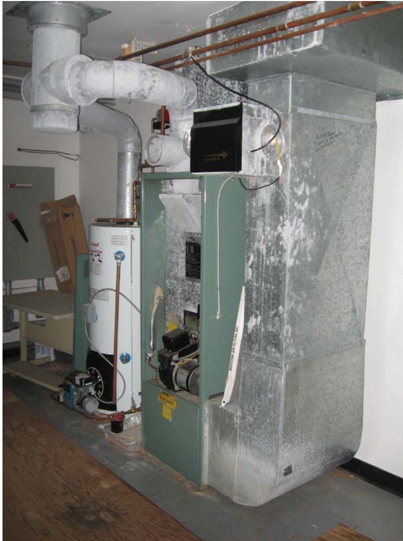
Photo 5: Furnace System.
