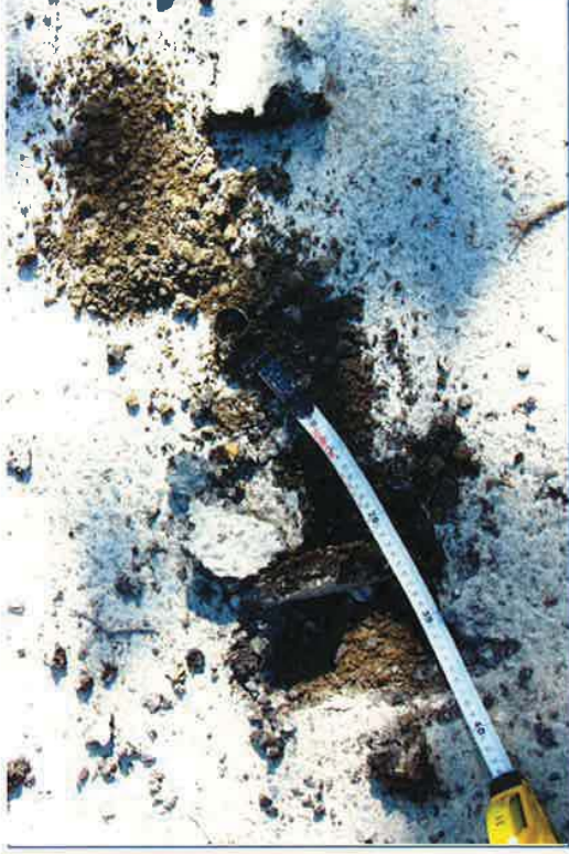
PHOTO 16 Close-up of pavement capping on old highway through campground - to be removed.
