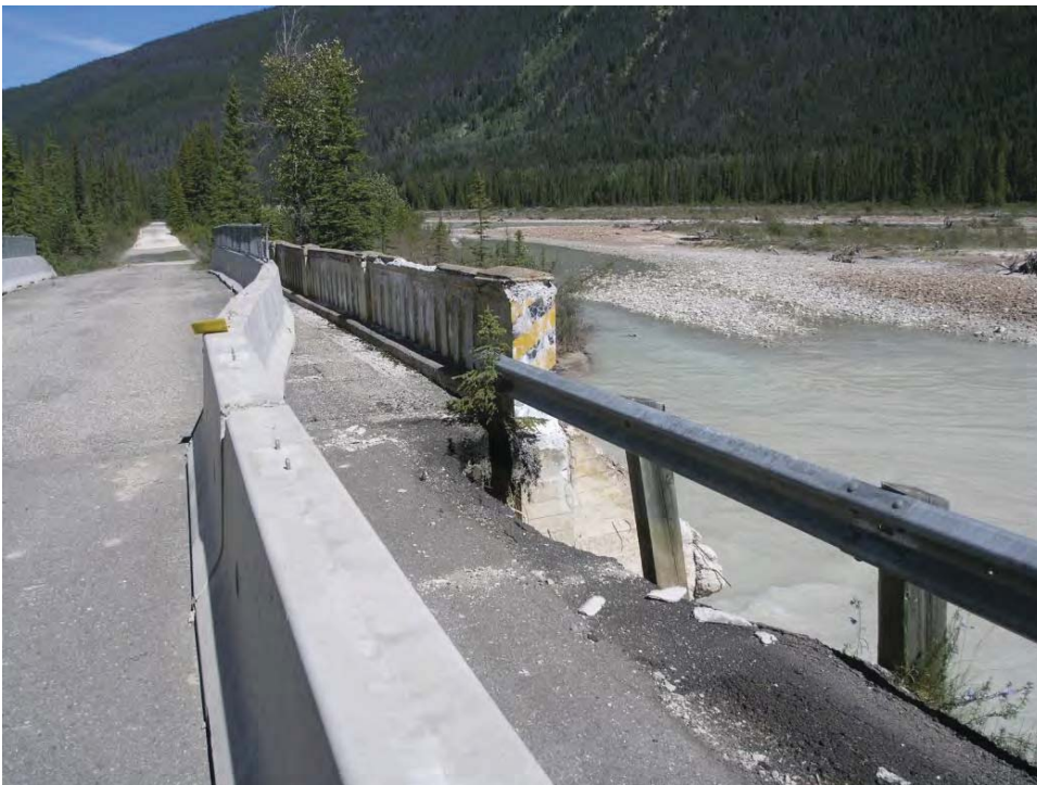
Figure 4 View of bridge top of Chancellor Peak bridge and erosion. View NE.
