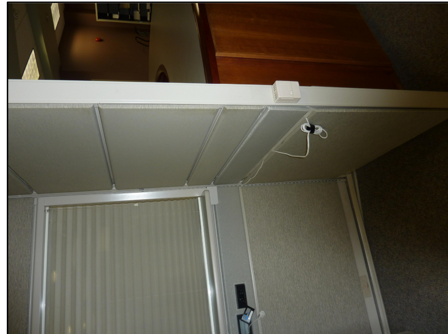
10 JET ZONE DIFFUSER THERMOSTATS TO BE DISMANTLED- WORK INCLUDES REMOVING ASSOCIATED DAMPERS AND CONTROLS.
