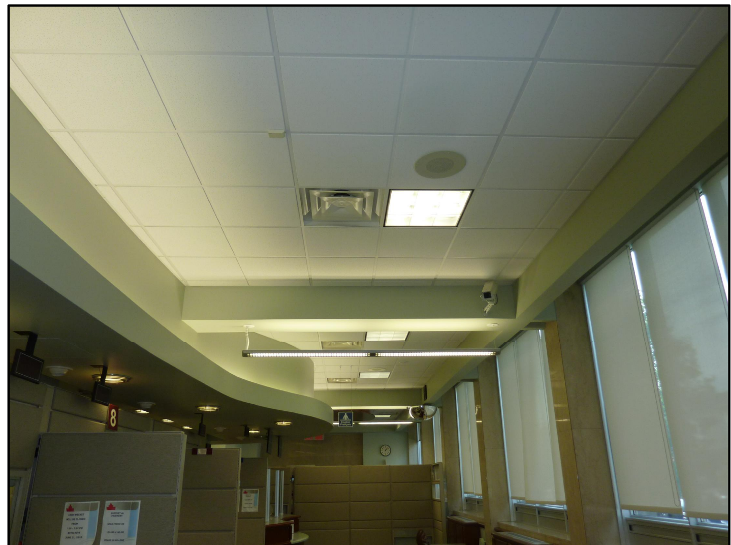
11 EXISTING DIFFUSERS ON GROUND FLOOR - NEW DIFFUSERS TO MATCH EXISTING
