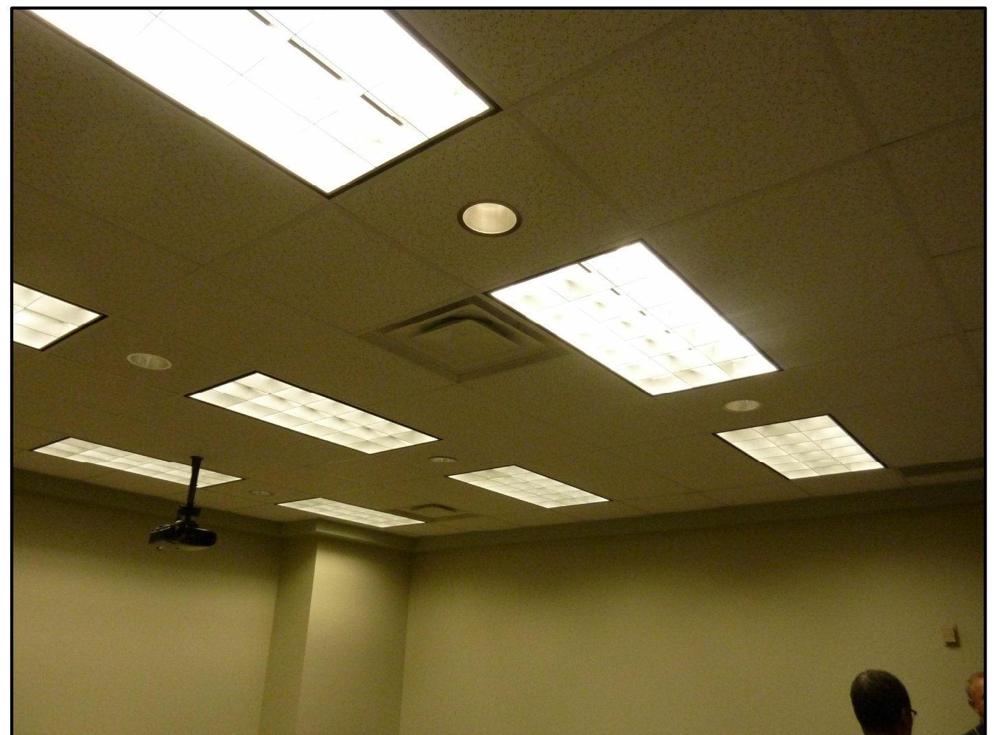
7 EXISTING SUPPLY AIR DIFFUSERS ON SECOND FLOOR - NEW DIFFUSERS TO MATCH EXISTING
