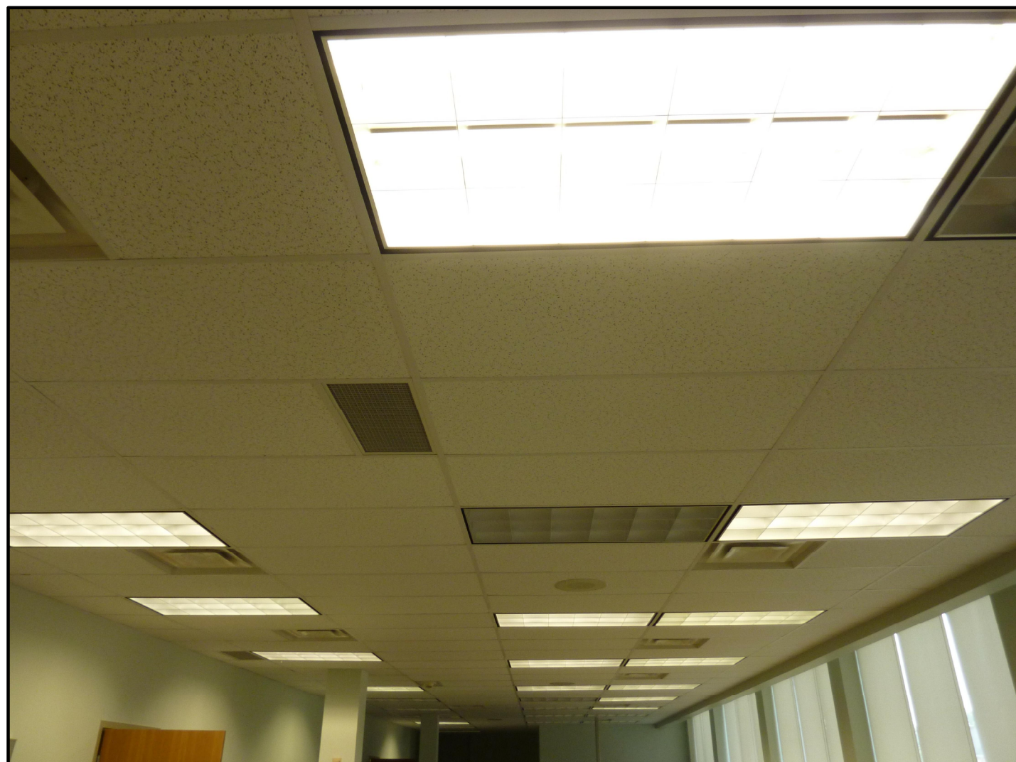
9 EXISTING EGG-GRADE RETURN : NEW EGG GRATES USED IN VICINITY OF EXISTING ONES TO MATCH
