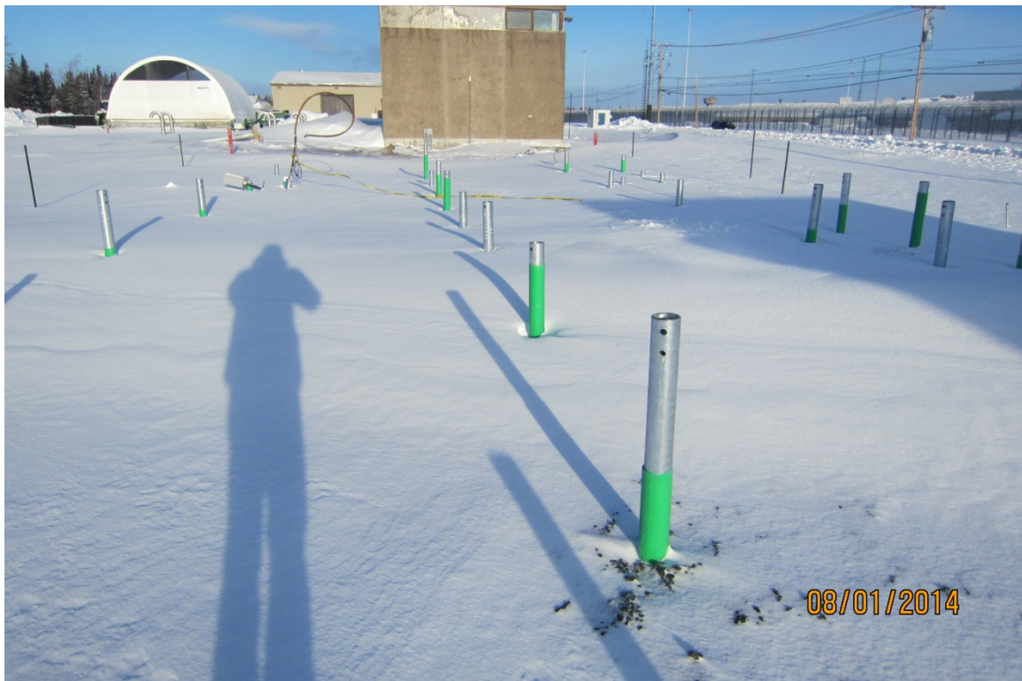
* The plates on the piles are being installed
