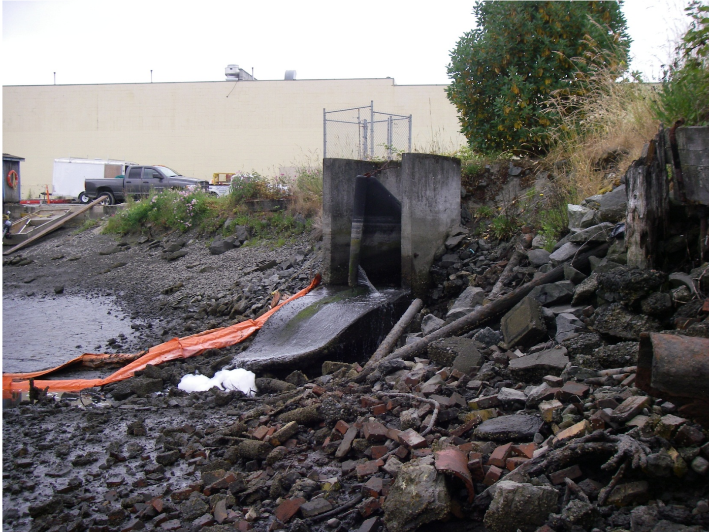
Photo 18: Close up of outfall 626 with headwall structure and check valve (tidegate).
