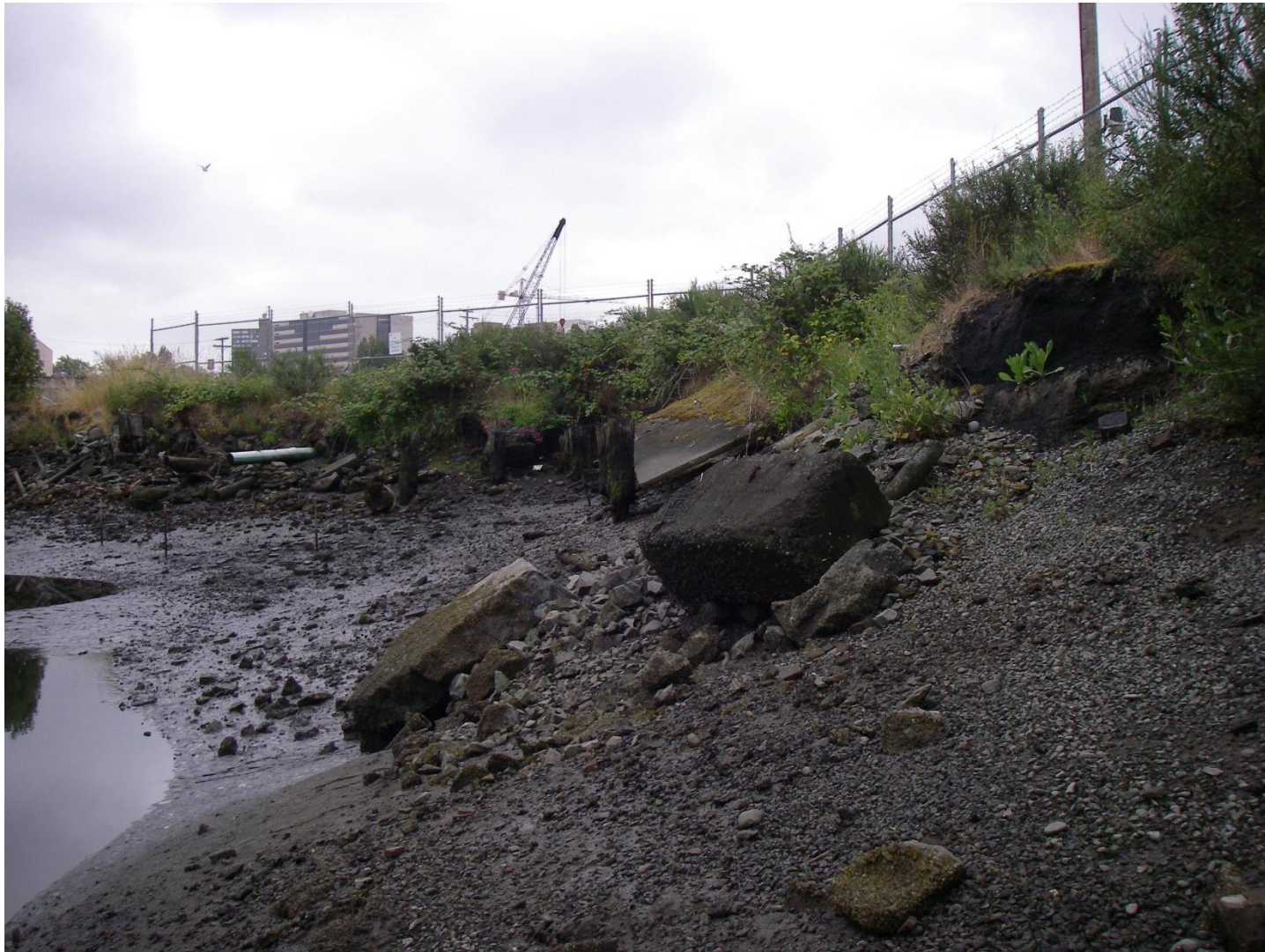
Photo 13: Looking east along the south shoreline of Rock Bay (West Excavation Area).
