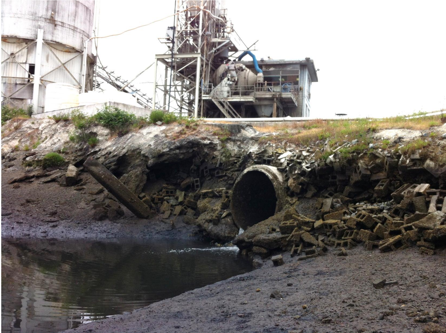
Photo 21: Looking northwest at outfall 627.
