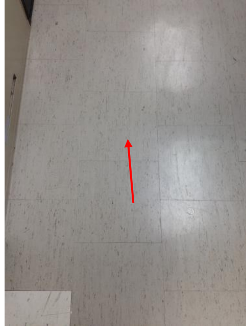
Photograph 2: [2 nd Floor Library] Asbestos-containing 12"x12" beige vinyl floor tiles with black streaks in the kitchen and office area of the library (Sample Set CCIW-10).
