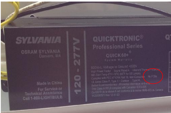
Photograph 7: [2 nd Floor Library] Fluorescent light ballast displaying “No PCBs” signage. Most ballasts in the subject areas were observed to be PCB-free, but it is possible that some ballasts contain PCBs.
