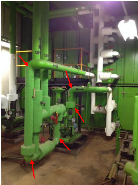
Photograph 3: [3 rd Floor Mechanical Room] View of asbestos-containing mechanical insulation on pipe elbows, flanges and valves (Sample Set CCIW-12).
