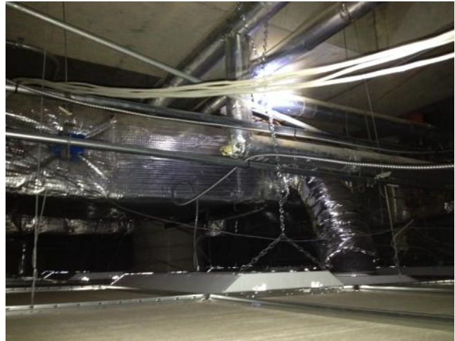
Photograph 6: [Ground Floor Office Area] Fibreglass insulation with foil wrap on ducts and pipes, observed throughout subject areas, which is non-asbestos-containing.
