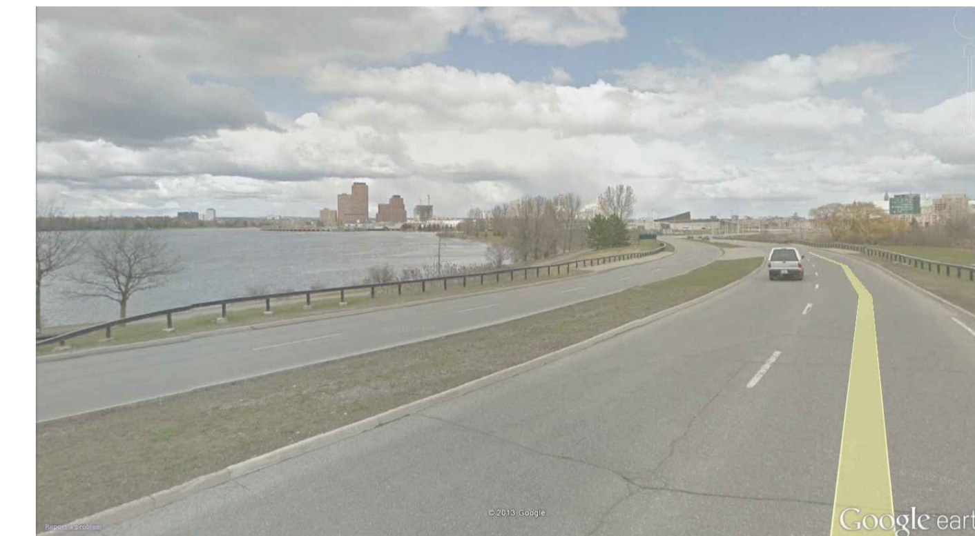
RAMP E STRUCTURE LOOKING TOWARDS EAST
