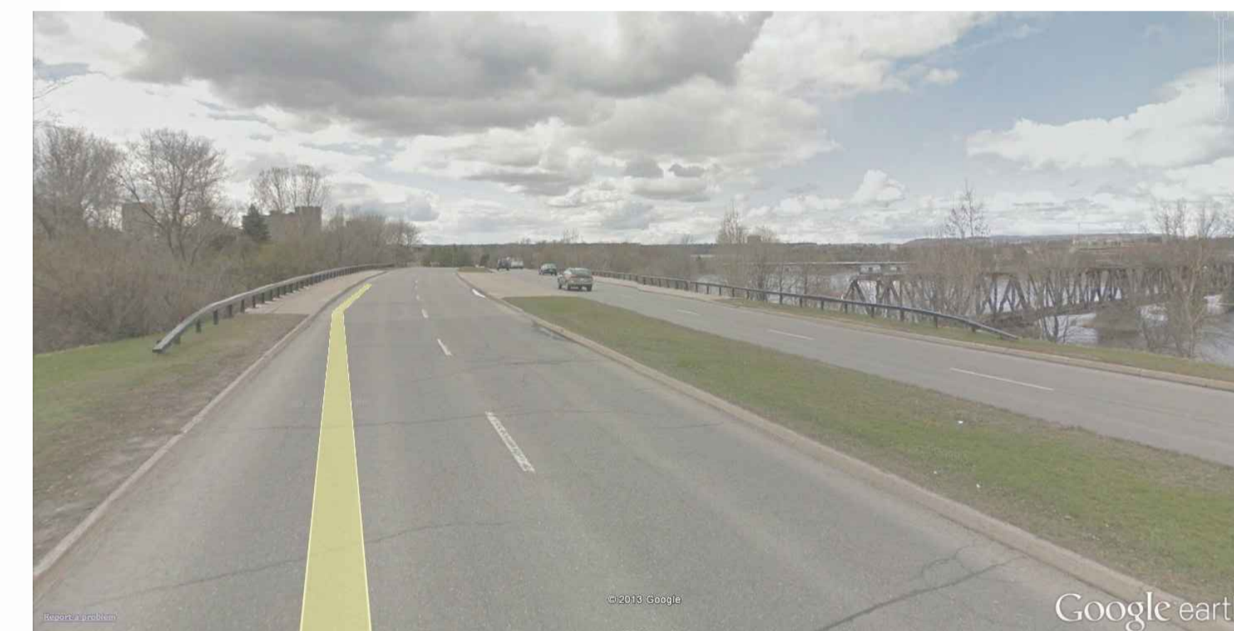
CPR STRUCTURE LOOKING TOWARDS WEST
