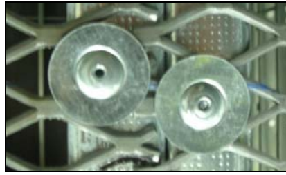
Figure 5: Example of mesh interlay seam, riveted
