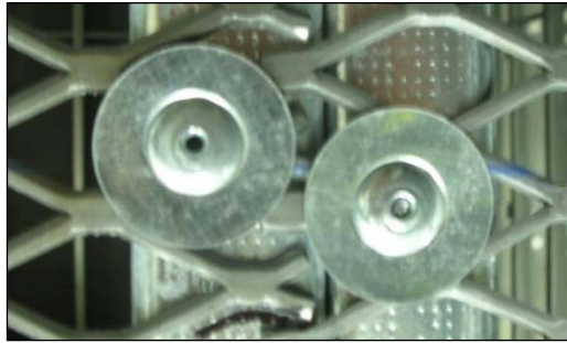
Figure 5: Example of Mesh Interlay Seam, Riveted
