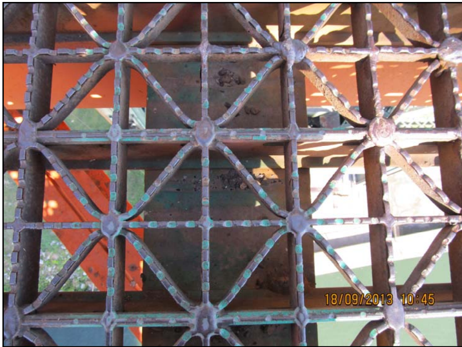
Photo 4: Close up view of the grating and supporting beam. Paint on the top of the beam is partially covered by dirt.
