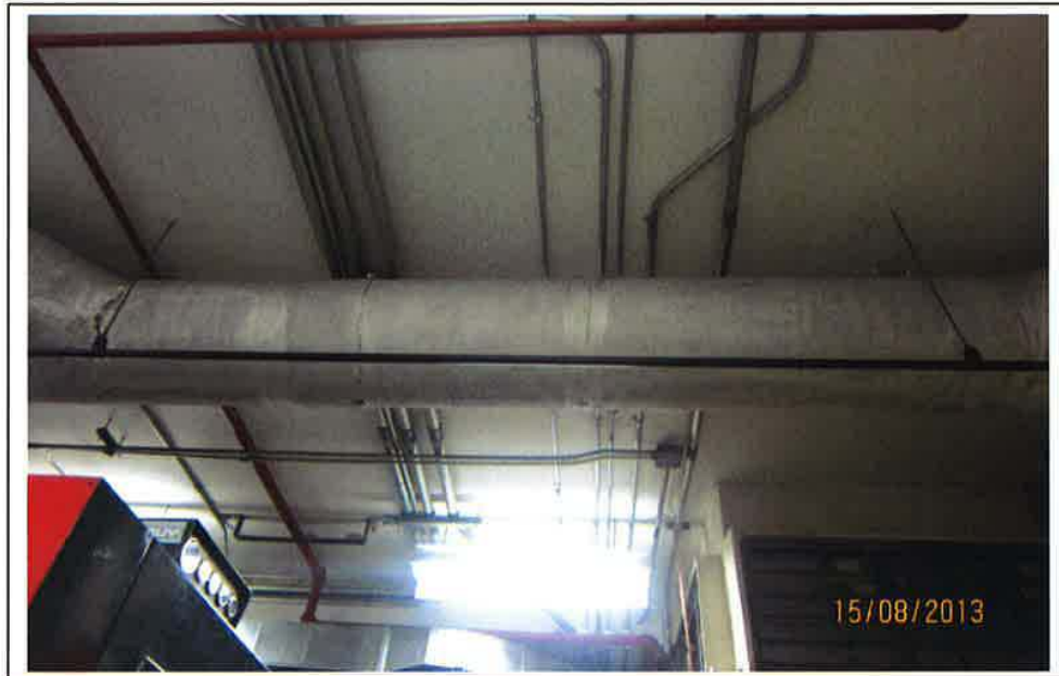
5 – CEILING VIEW (GENERATOR EXHAUST CONDUIT)
