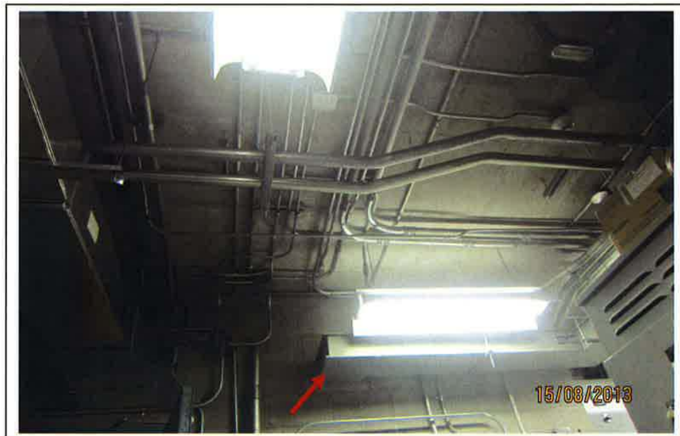
11 – NORMAL POWER BUS DUCT IN THE ELECTRICAL ROOM
