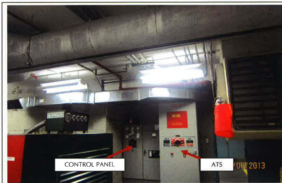
4 – GENERATOR CONTROL PANEL, EXISTING ATS VENTILATION AIR DUCT AND AIR INTAKE
