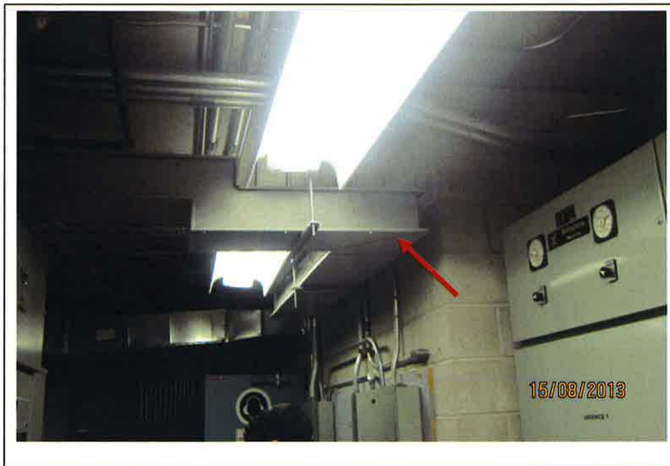
13 – NORMAL POWER BUS DUCT IN THE ELECTRICAL ROOM AND CDU
