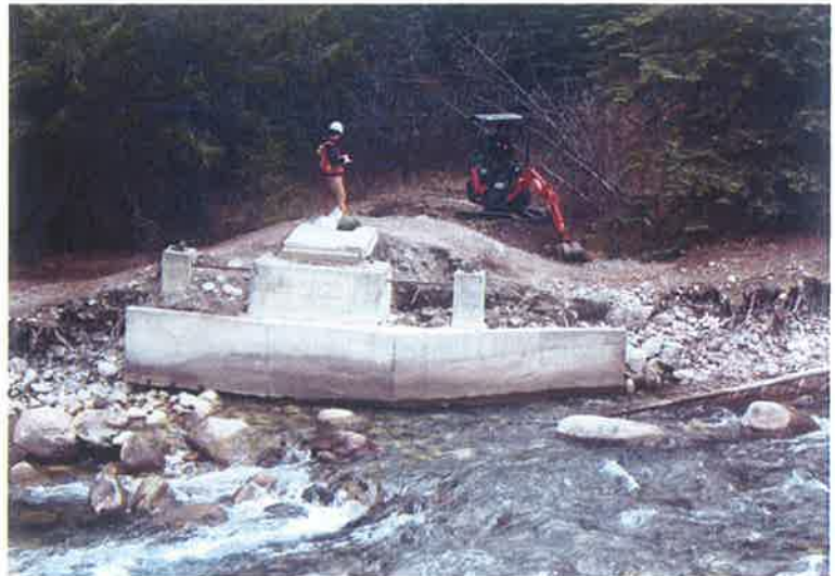
Photo 3. North bank of project
