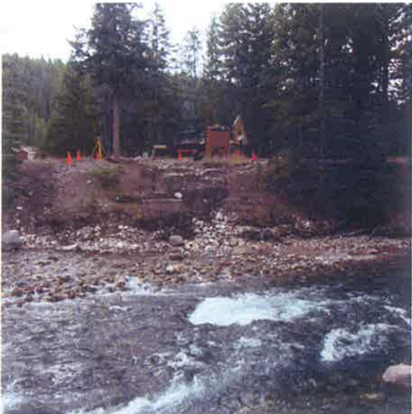
Photo 2. South bank of project
