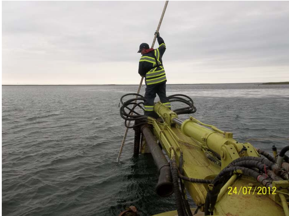
Photo 3 - Manual sounding undertaken at test pit locations.
