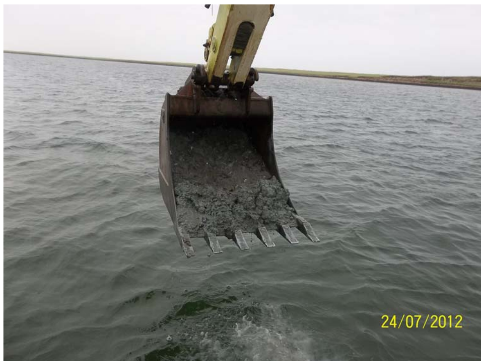
Photo 10 - Grey silty sand with some cobbles encountered at TP 6 - McEachern's Point (Elevation –1.86 to –2.36 CD).
