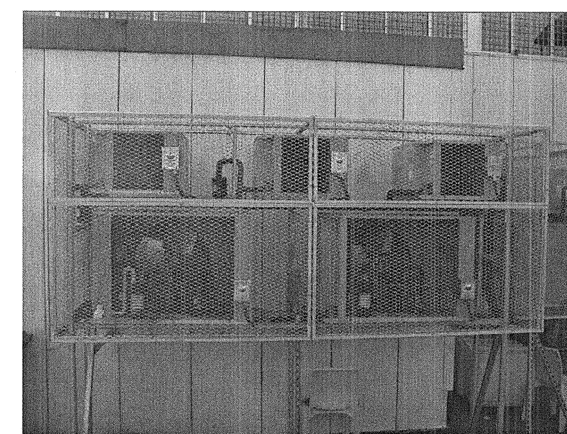
PICTURE #3 EXISTING COMPRESSOR LOCATED AT BOTTOM LEFT. USE EXISTING WIRING AND DISCONNECT SWITCH FOR NEW COMPRESSOR.
