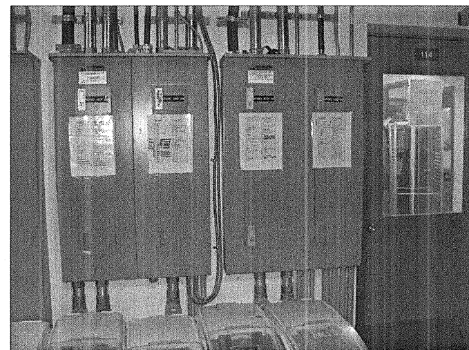
PICTURE #1 EXISTING PANEL 'AS2D' BY THE DOOR. PANEL FEEDS ALL EQUIPMENT RELATED TO EXISTING COOLER. USE TO FEED NEW FREEZER.
