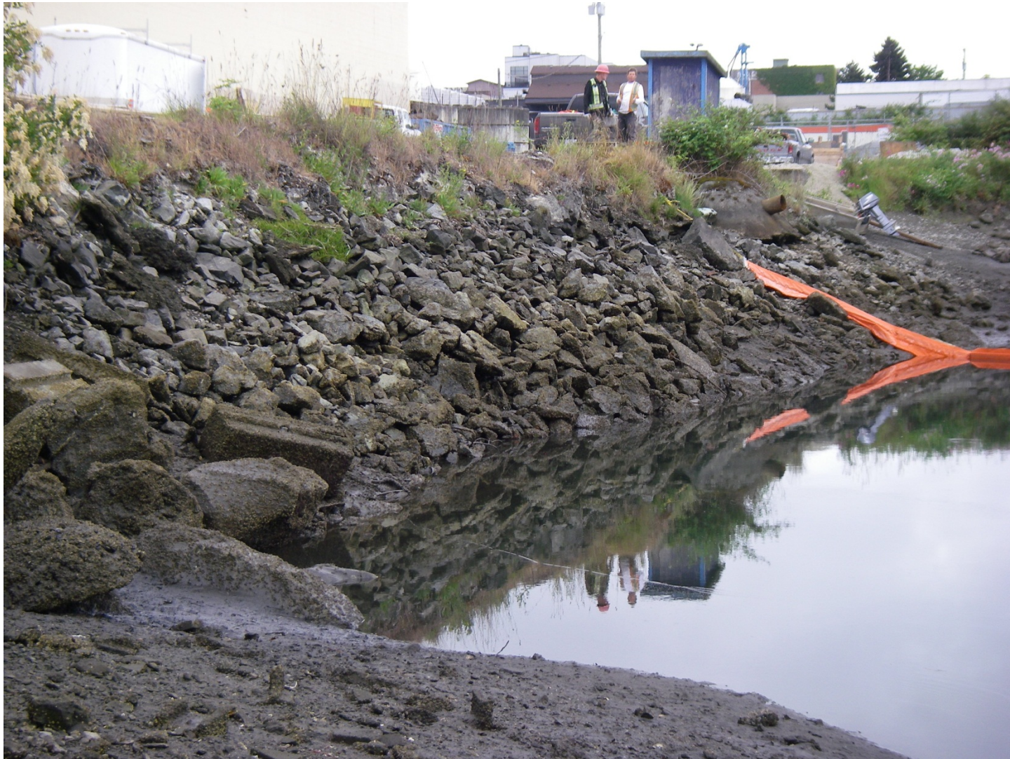
Photo 20: Looking south along the east shoreline of Rock Bay.
