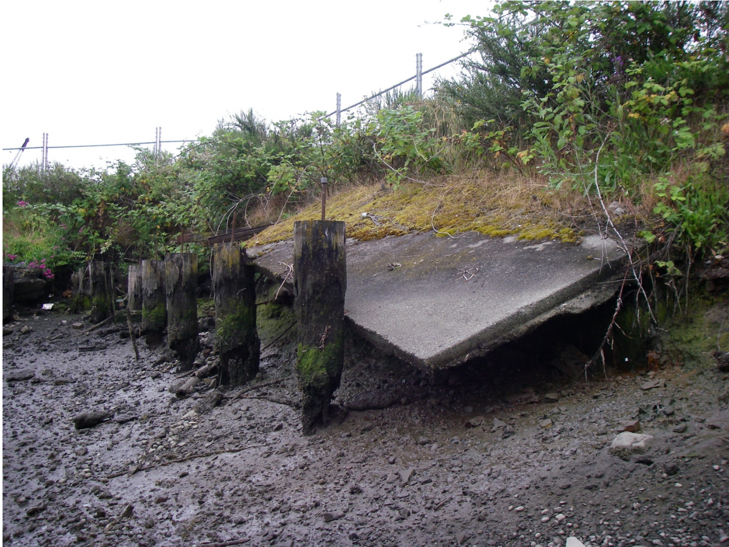
Photo 14: Old timber pilings and concrete dock on south shoreline of Rock Bay.
