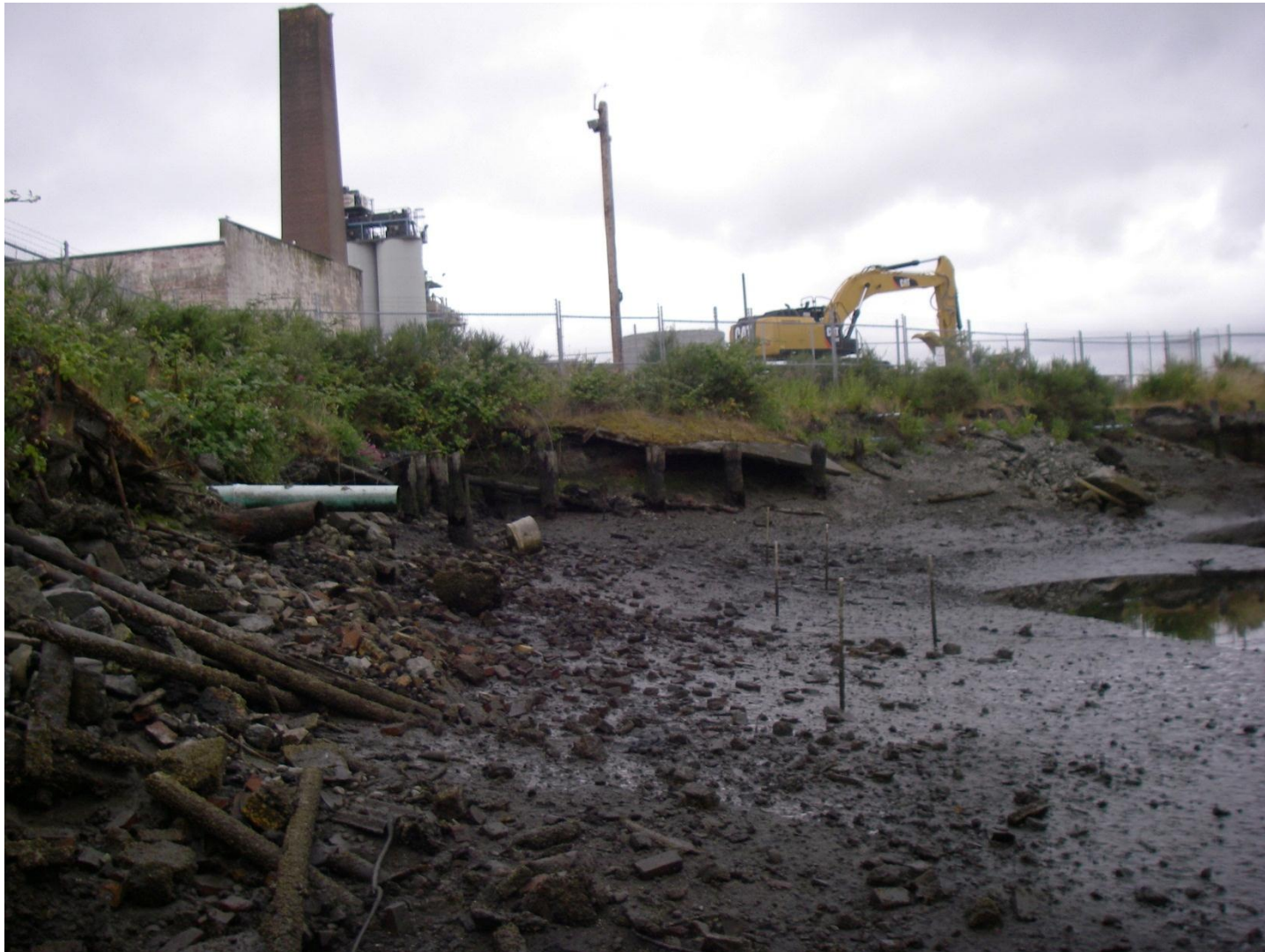
Photo 17: View looking west along the south shoreline of Rock Bay.
