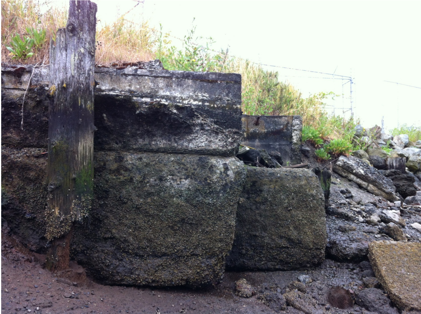
Photo 15: Old timber pilings and concrete dock on south shoreline of Rock Bay.
