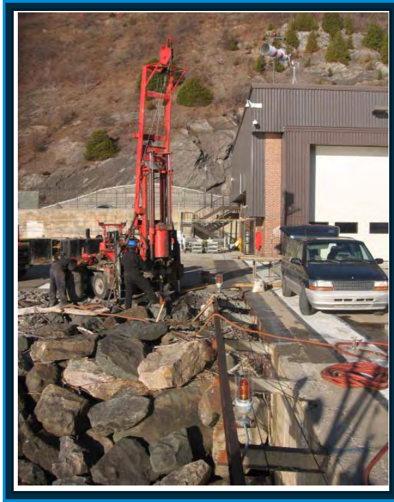
PHOTO #5: View of TF-08-09 rock drilling at the edge of the wharf.
