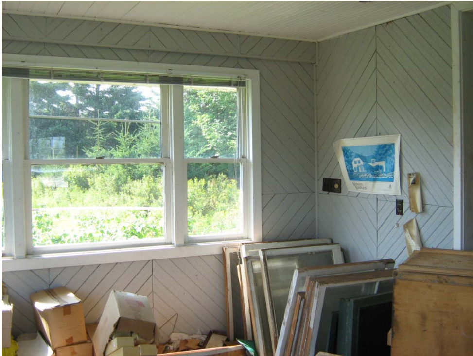
PHOTO No. 25: Asset No. 404 – Interior.
