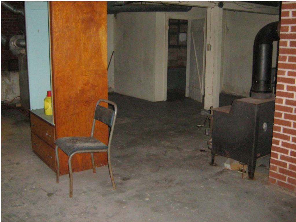
PHOTO No. 58: Asset No. 108 – Basement.
