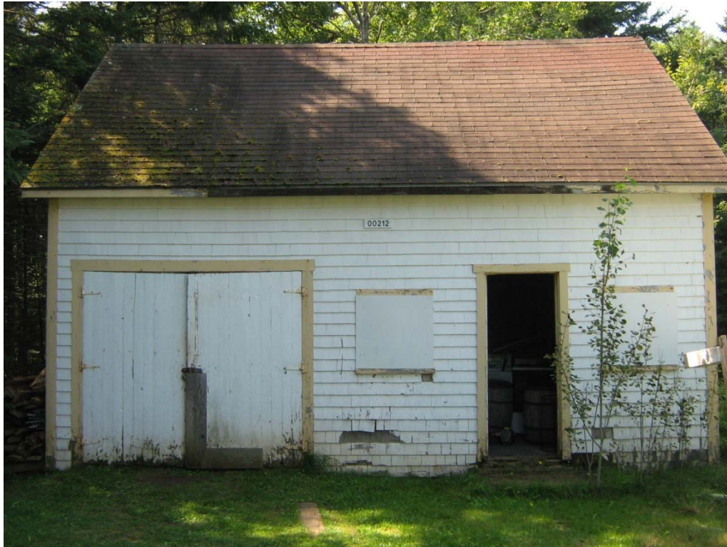
PHOTO No. 43: Asset No. 117 – Garage with Asset 106 – view from east.
