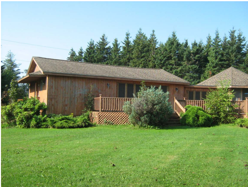
PHOTO No. 2: Cavendish Canteen – view from northeast.
