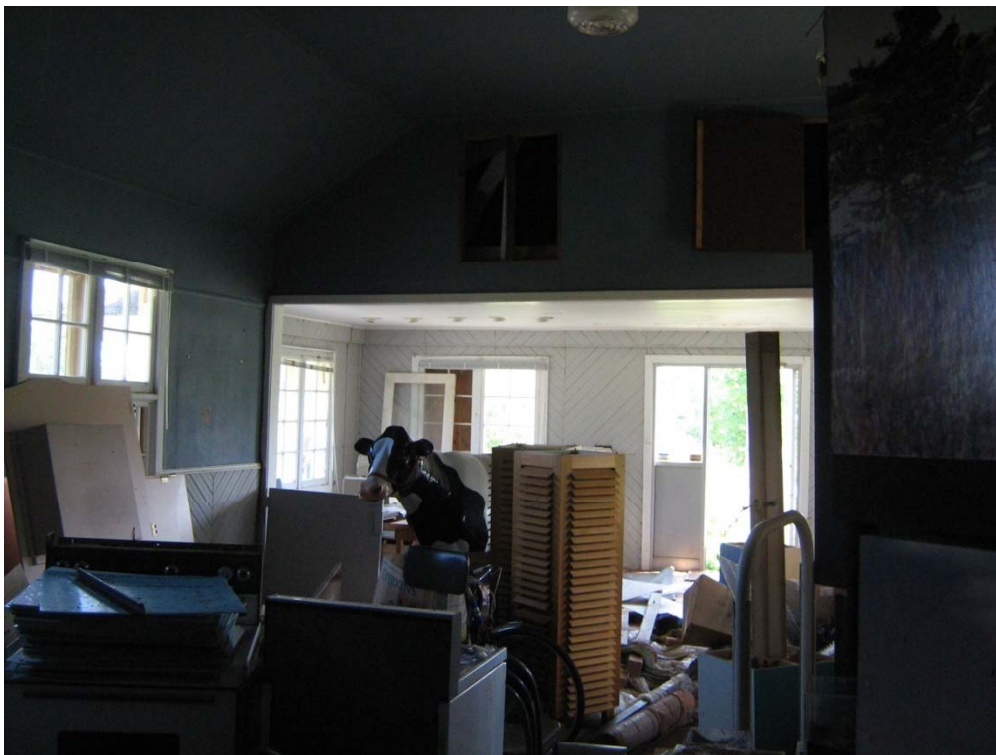
PHOTO No. 26: Asset No. 404 – Interior.
