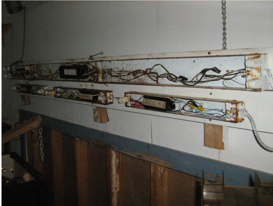
PHOTO No. 27: Asset No. 404 – Fluorescent light ballasts in projection room (potential PCB containing).
