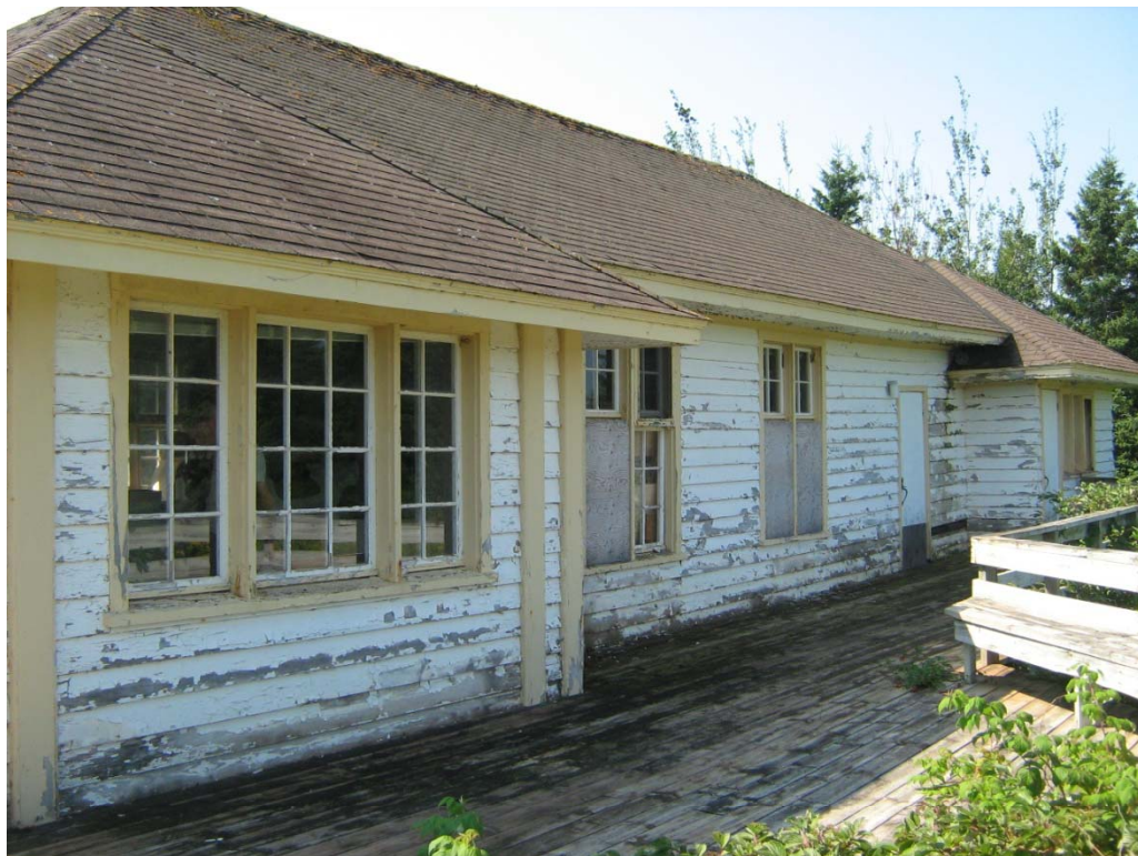
PHOTO No. 22: Asset No. 404 – north side of building - photo facing southwest
