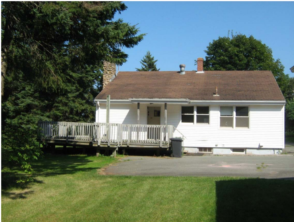
PHOTO No. 48: Asset No. 108 – view from west.
