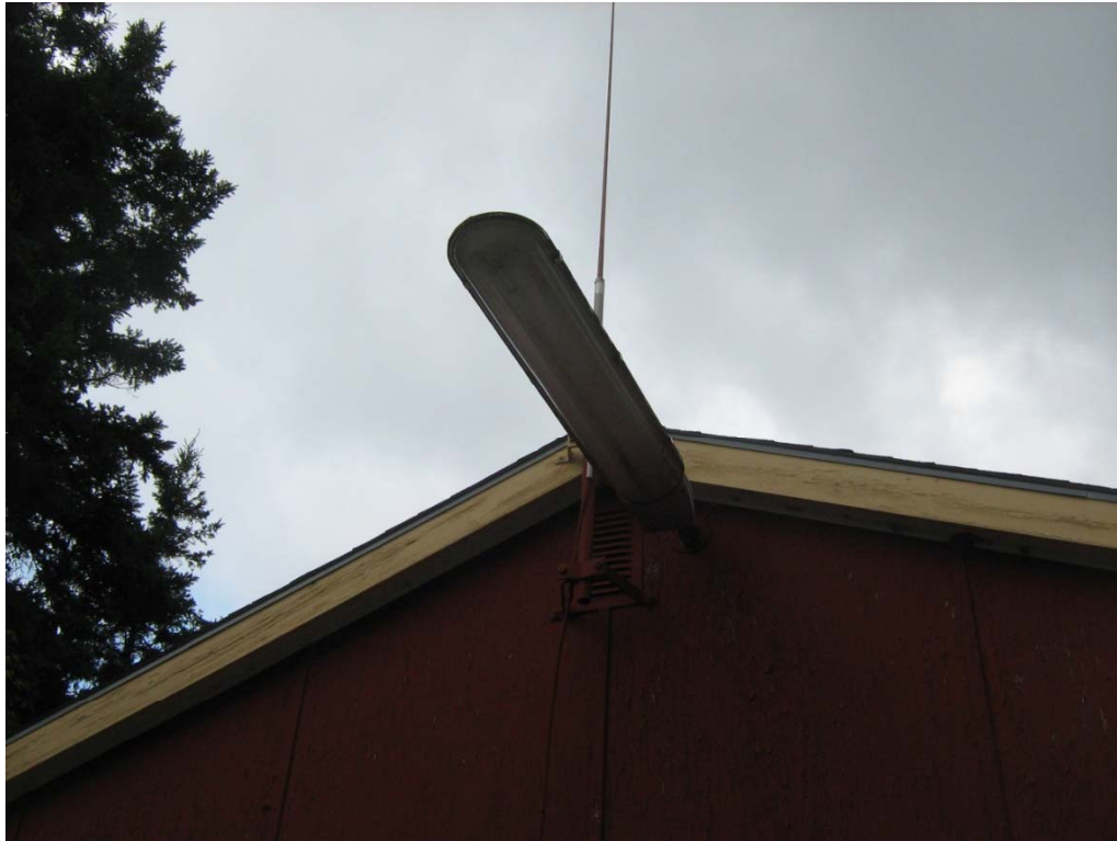
PHOTO No. 69: Asset No. 303 – Fluorescent Light (potential PCB/mercury containing).
