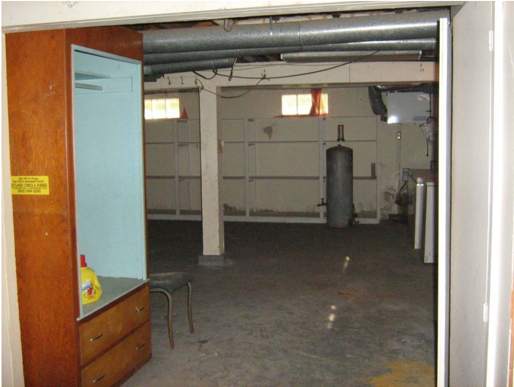
PHOTO No. 57: Asset No. 108 – Basement.
