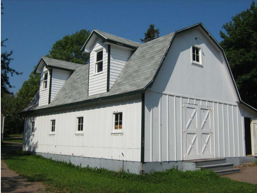
PHOTO No. 12: Cavendish Grove Art Barn – view from southeast.
