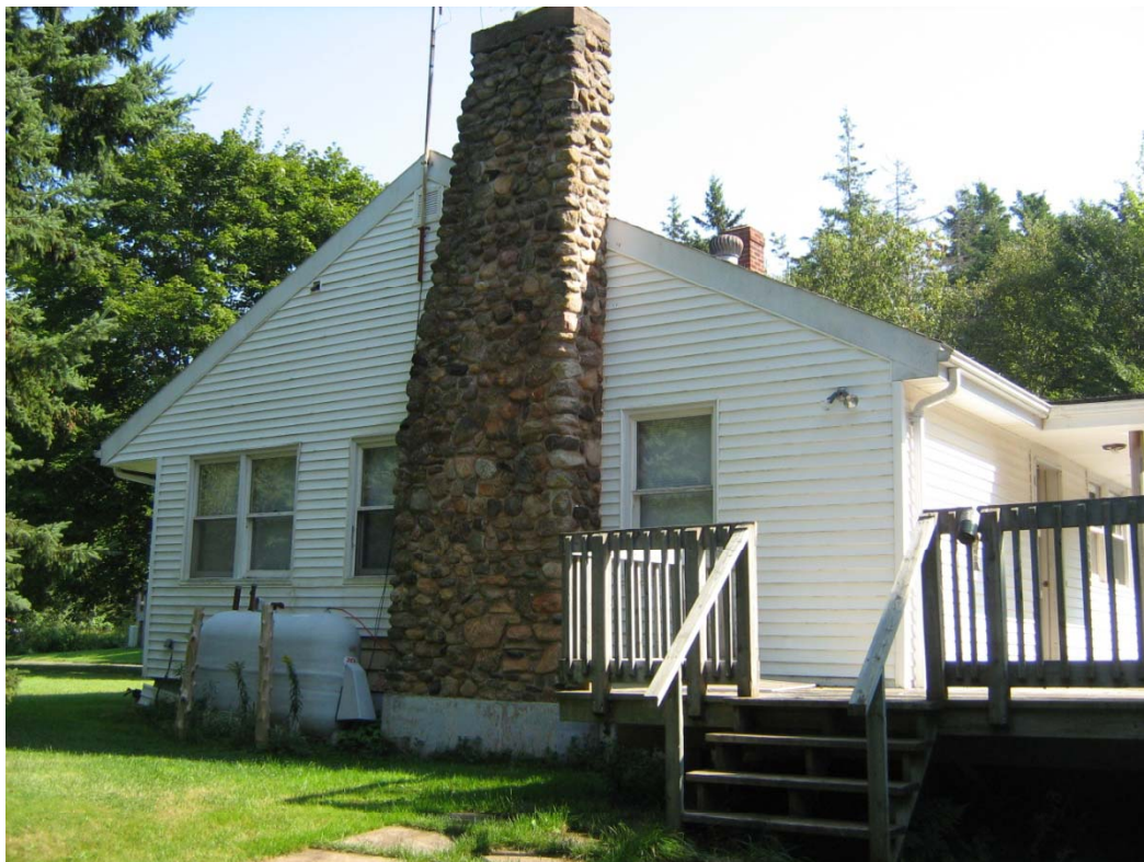
PHOTO No. 46: Asset No. 108 – view from north.
