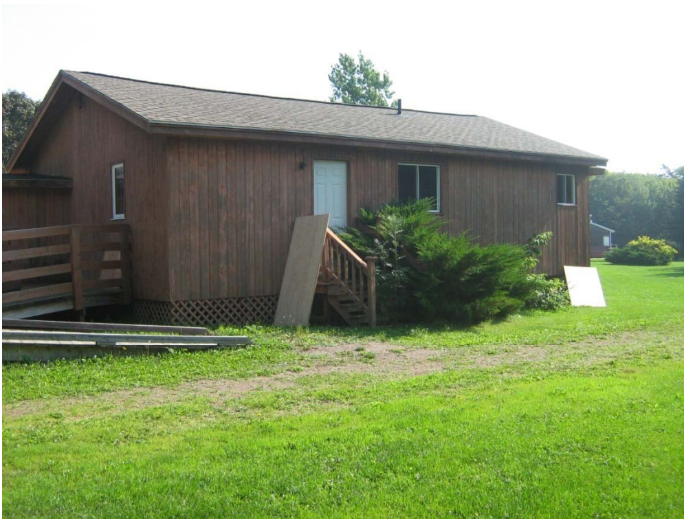
PHOTO No. 4: Cavendish Canteen – view from southwest.
