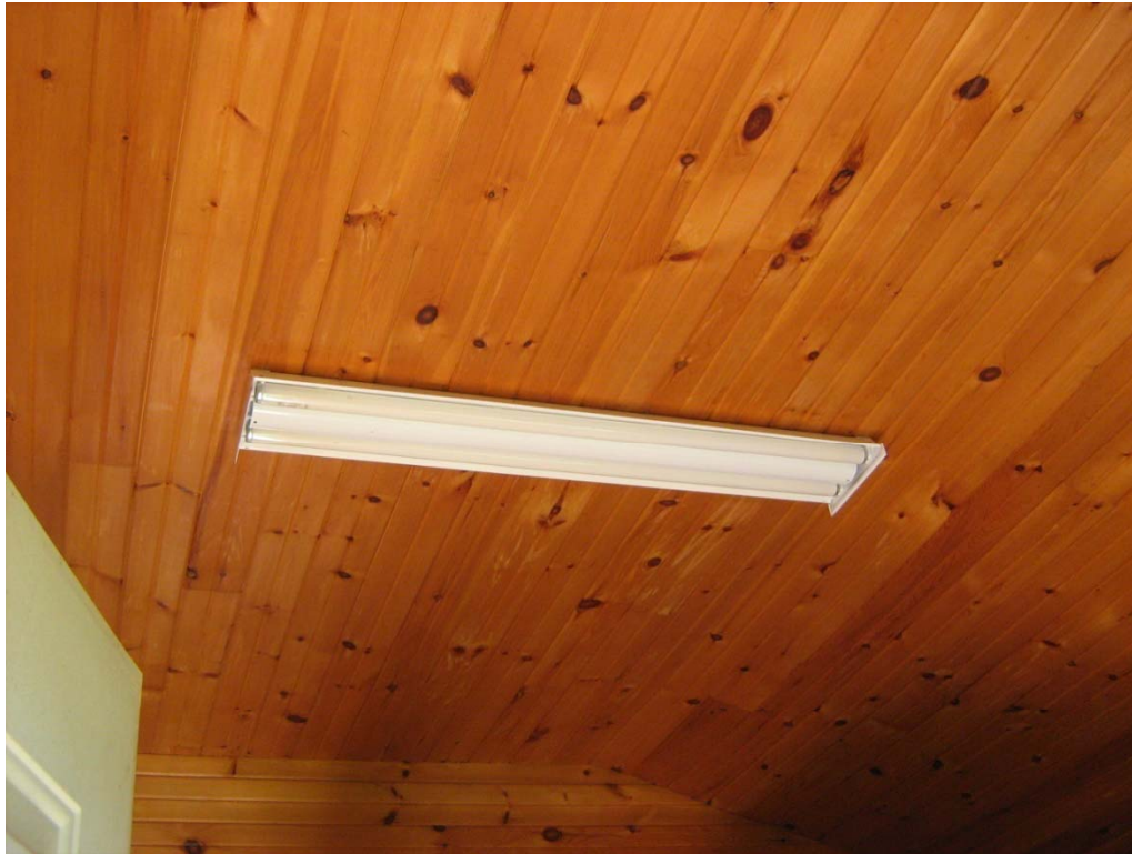
PHOTO No. 11: Cavendish Canteen – Fluorescent Light on washroom ceilings (potential PCB/mercury containing).
