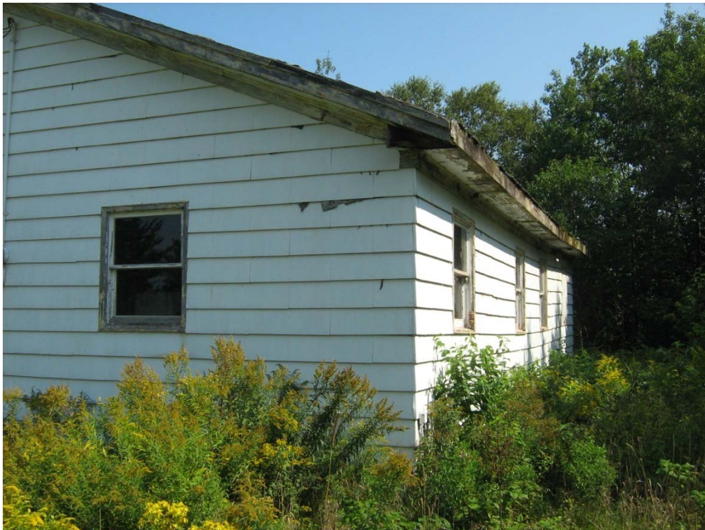
PHOTO No. 30: Asset No. 112 – view from west.
