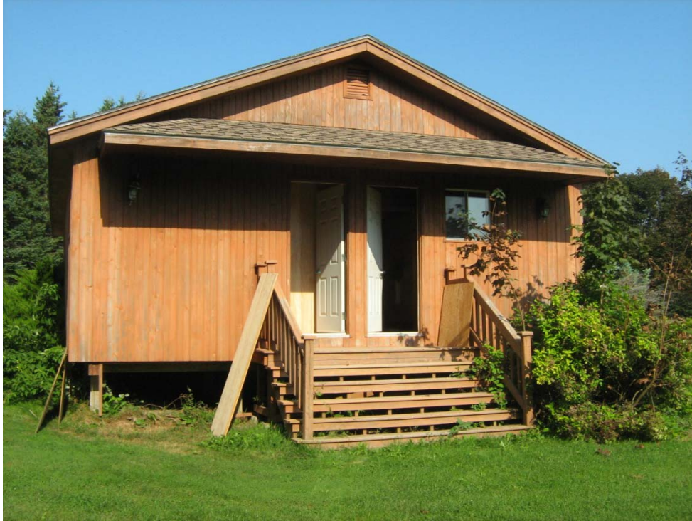
PHOTO No. 3: Cavendish Canteen – bathroom entrances – view east.
