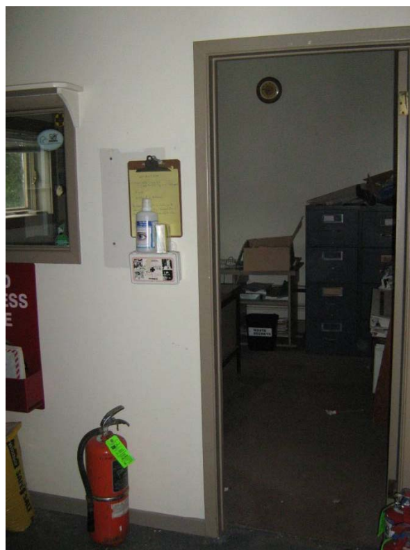
PHOTO No. 66: Asset No. 303 – Interior Office
