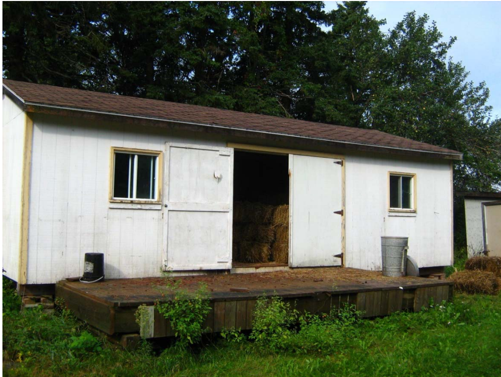
PHOTO No. 71: Asset No. 310 – Paint Grounds Building – view from east.
