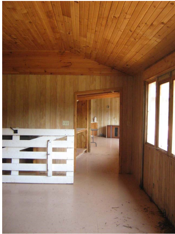
PHOTO No. 9: Cavendish Canteen – Multi Purpose Room and hall to Kitchen
