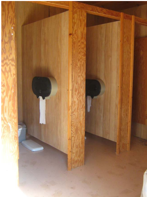
PHOTO No. 10: Cavendish Canteen – Interior Washrooms.
