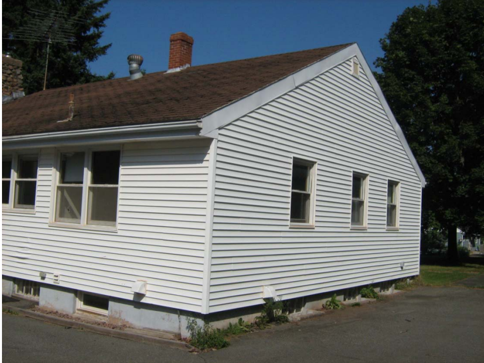
PHOTO No. 47: Asset No. 108 – view from southwest.
