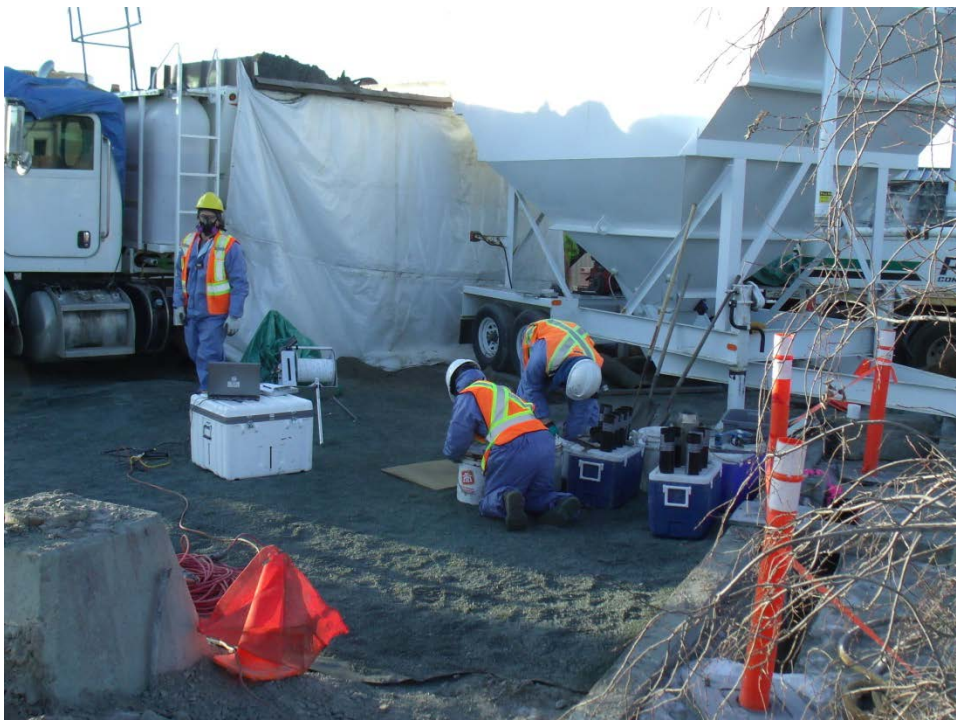
Figure 3: Cylinders Being Prepared in the Field
