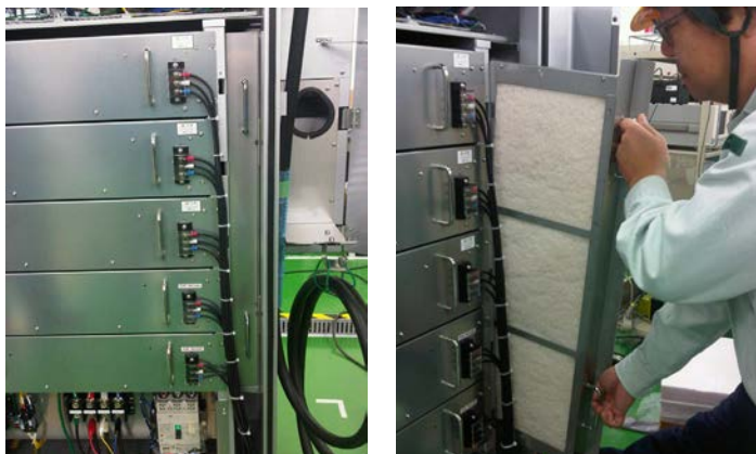
Figure 23. Filter Cleaning Procedure.
