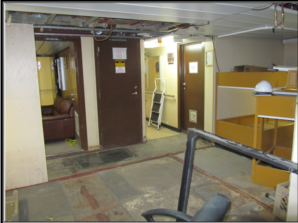
Main Deck Cabins above Fresh Water Tank - Bulkheads/Flooring Removed for Inspection
