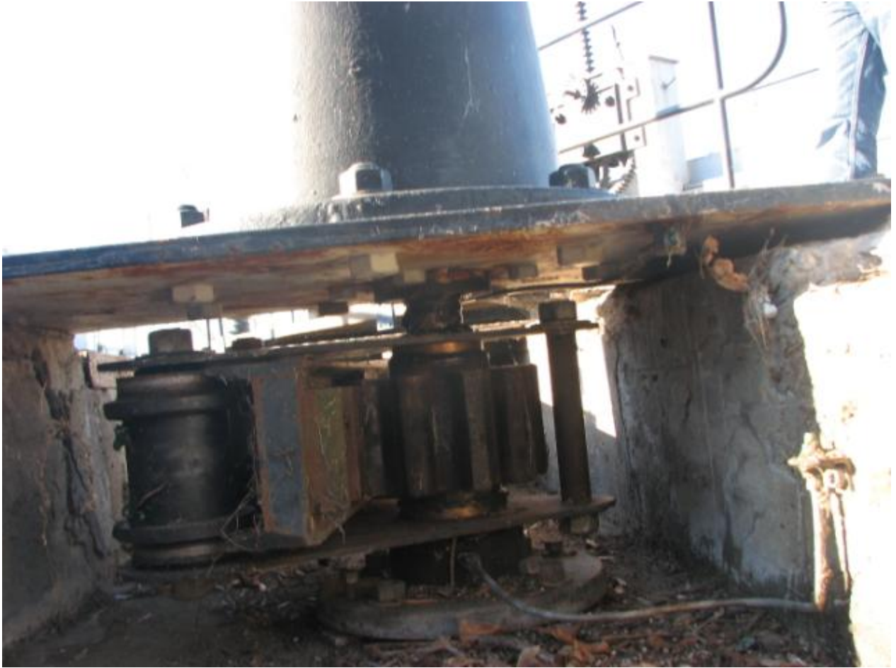
A15 –Rack and pinion, view toward canal
