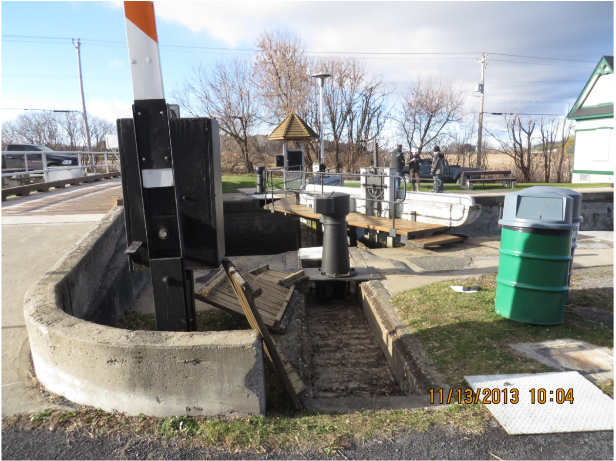
A14 – Right bank rack and pinion pit
