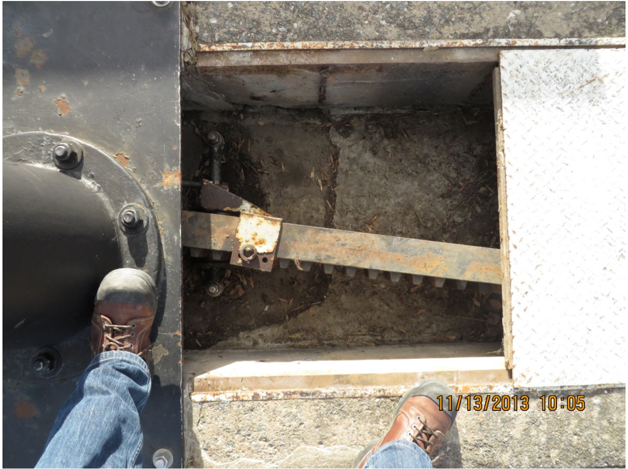
A17 – Right bank rack and pinion pit
