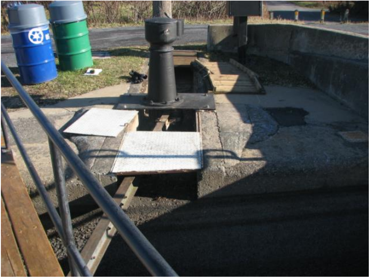
A13 – Right bank rack and pinion pit
