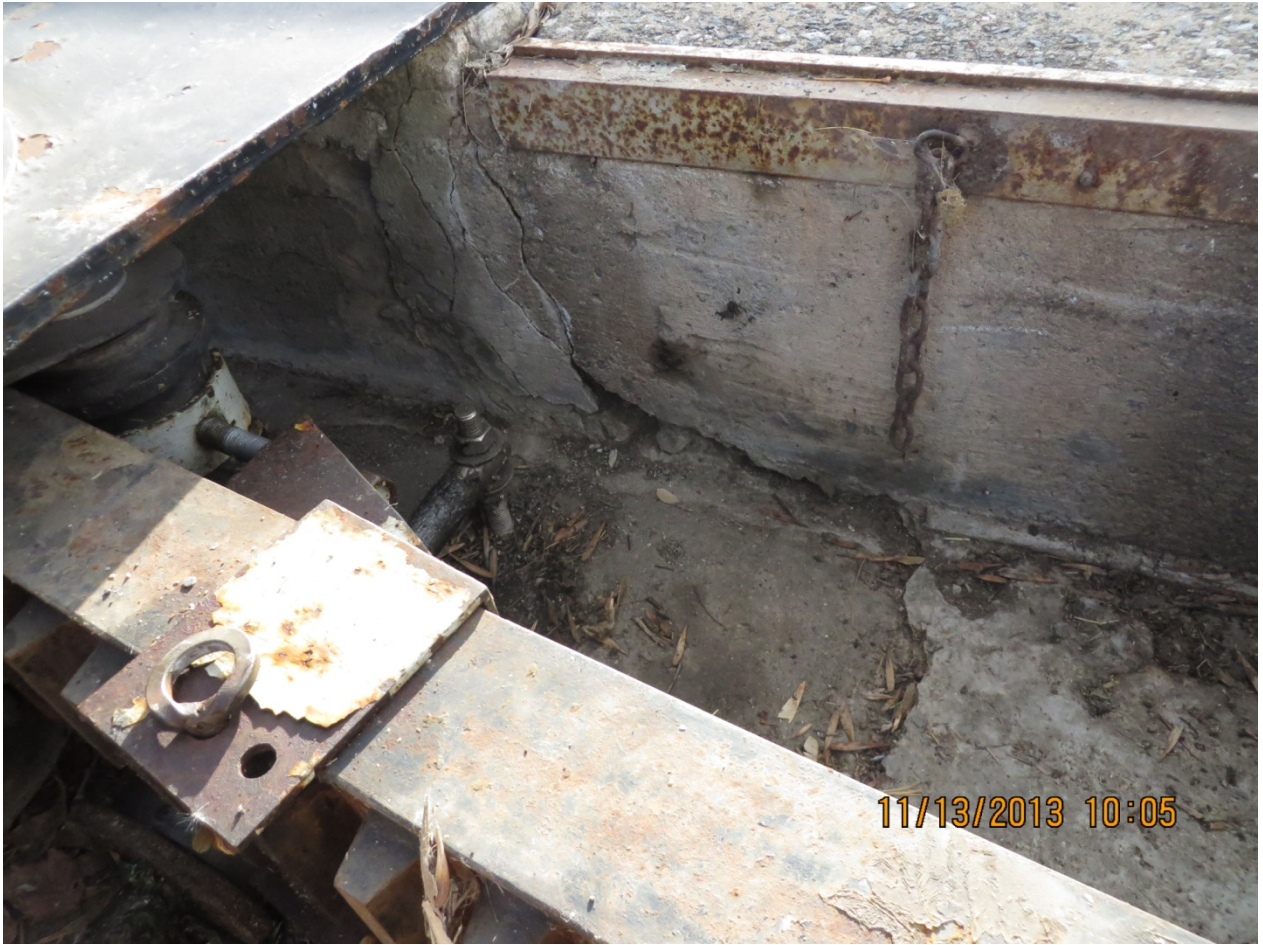
A16 – Right bank rack and pinion pit
