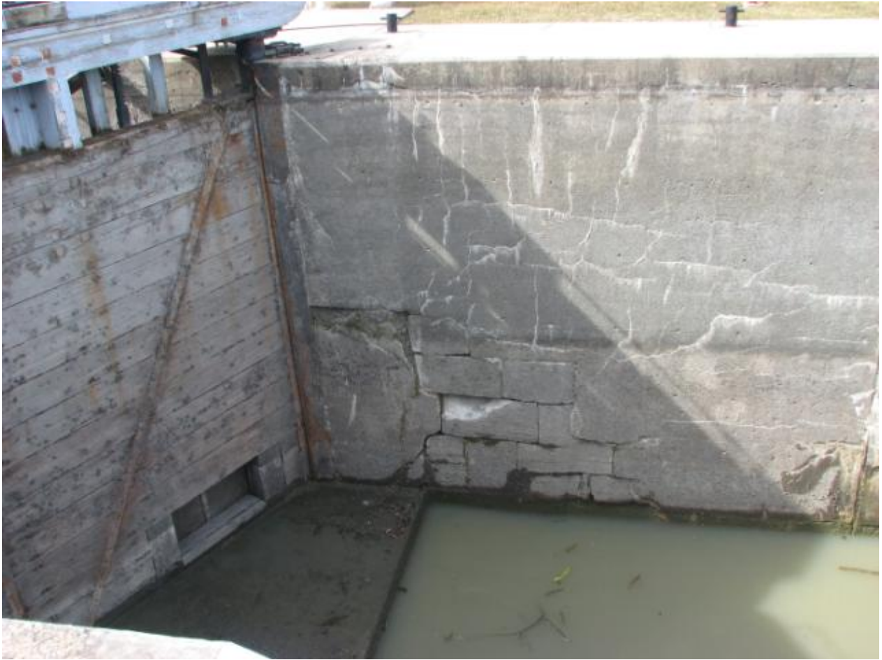
A1 – Downstream face of left gate
