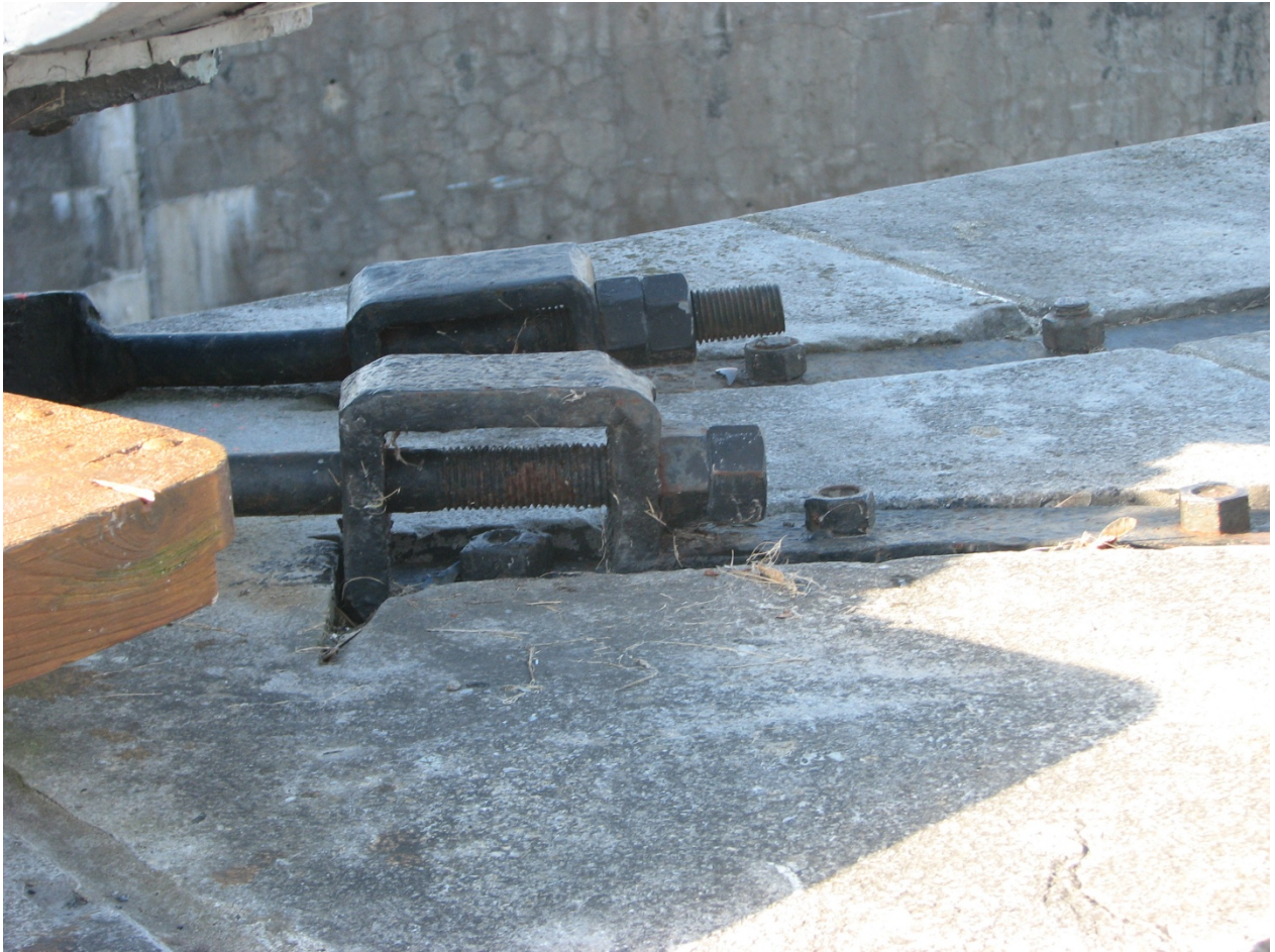
B8 – Straps' threaded rods
