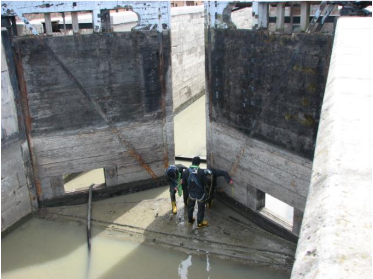
B2 – Downstream face of the gates
