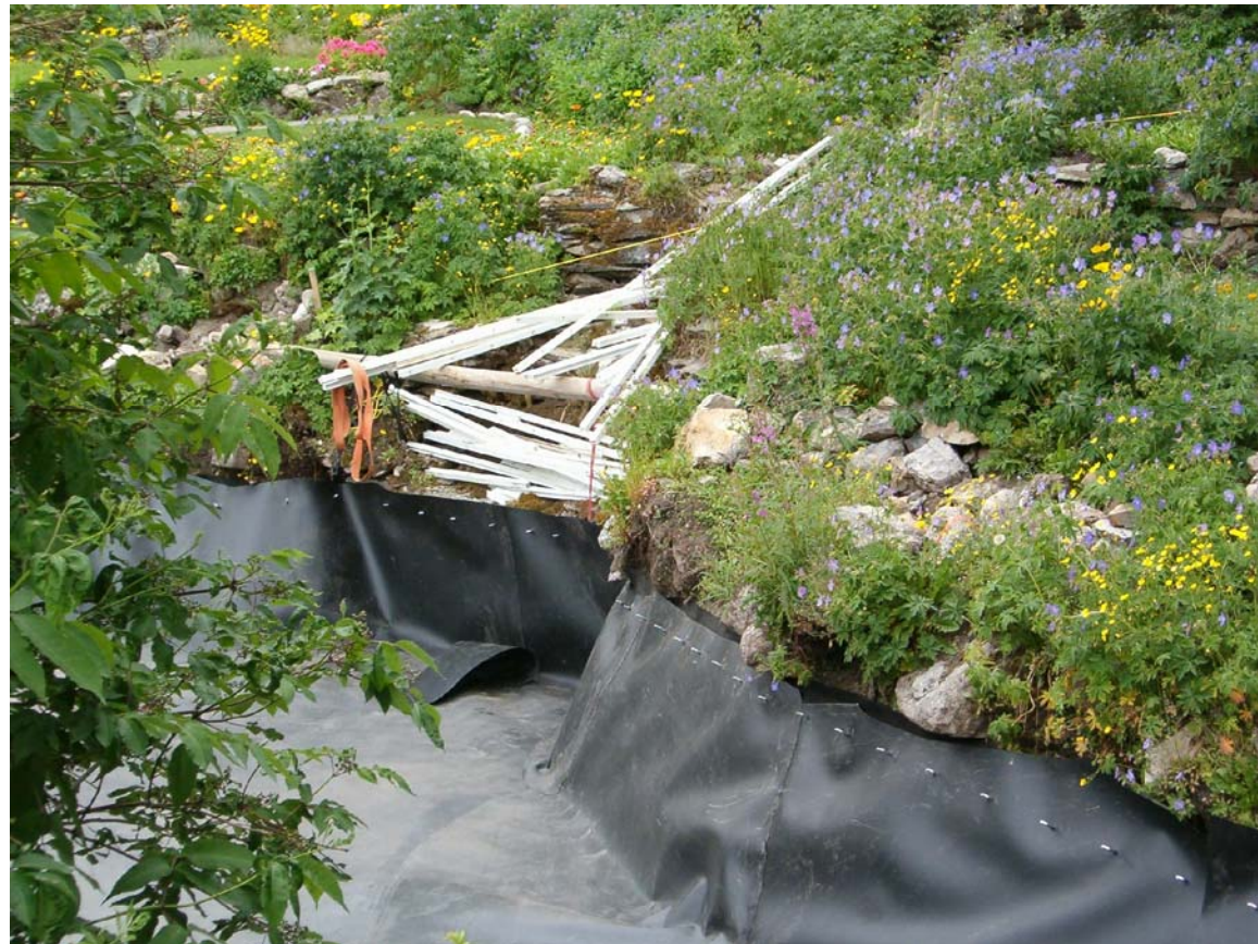
PHOTO #E24 INSTALLATION OF LINER MEMBRANE
