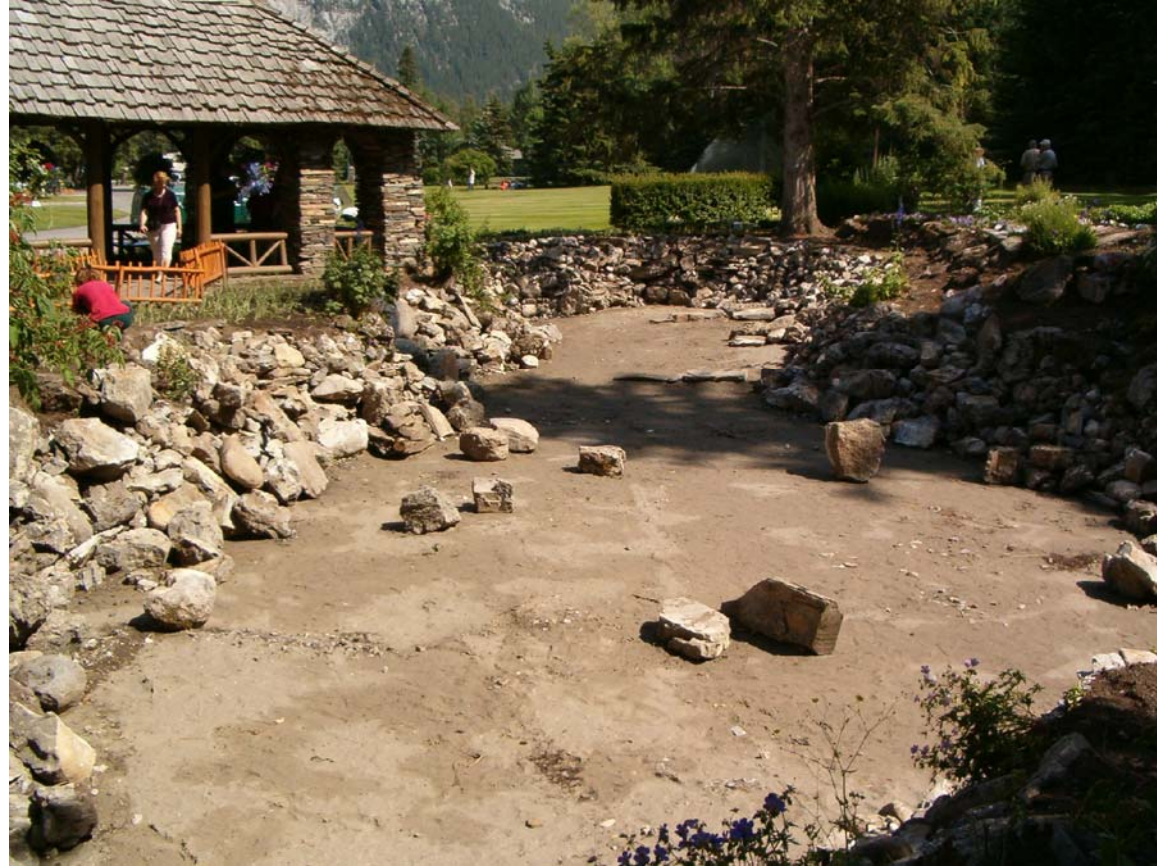
PHOTO #E30 STONES REPLACED IN POOL
