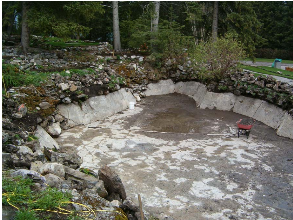
PHOTO #E12 ORIGINAL CONCRETE WALLS AND SLAB EXPOSED
