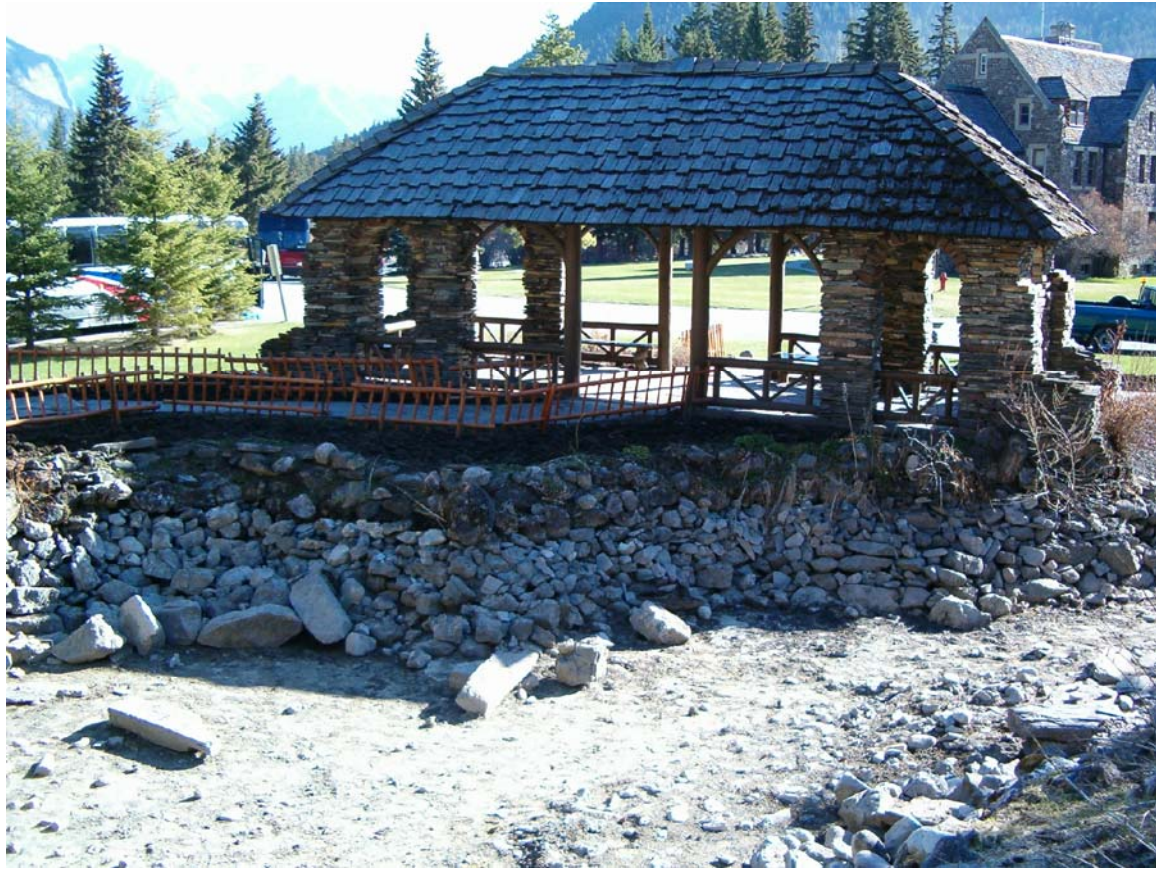
PHOTO #E1 RECORDING PRIOR TO REPAIRS
