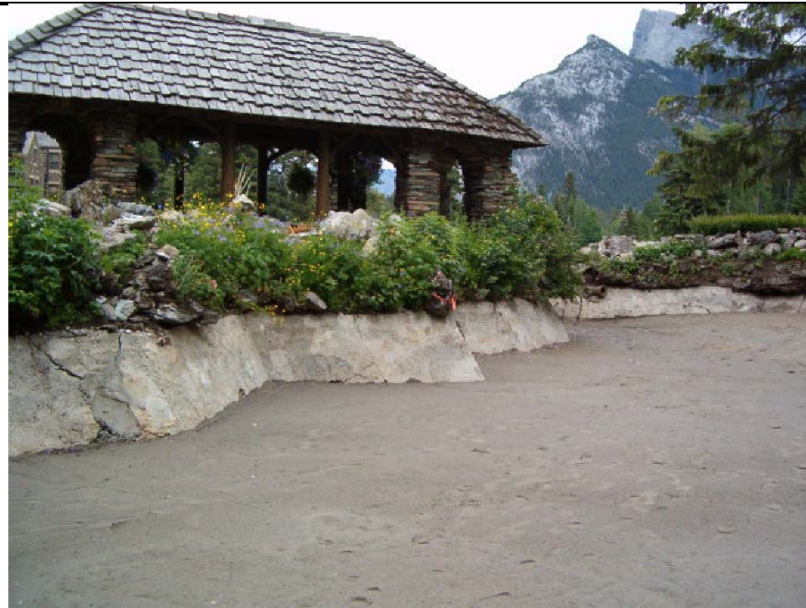
PHOTO #E14 CONC. WALLS REPAIRED & SAND BASE INSTALLED OVER SLAB
