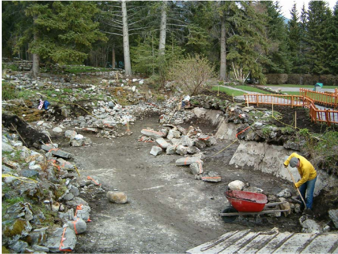
PHOTO #E5 REMOVAL OF STONES IN PROGRESS
