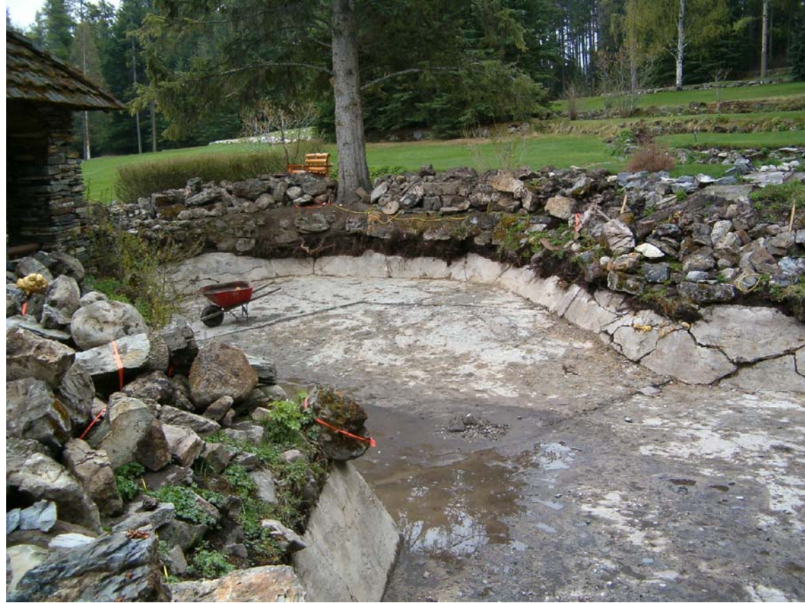
PHOTO #E10 ORIGINAL CONCRETE WALLS AND SLAB EXPOSED
