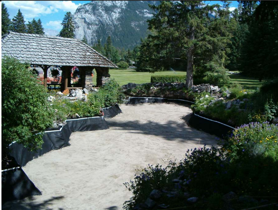
PHOTO #E25 INSTALLATION OF SAND BALLAST, FILTER FABRIC & PLASTIC CLAMPING CHANNEL
