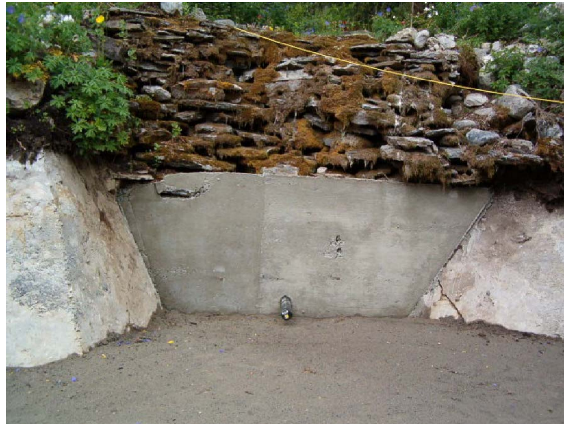
PHOTO #E16 NEW CONCRETE WALL & DRAIN PIPE AT CASCADE #2
