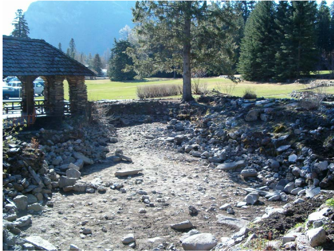
PHOTO #E2 RECORDING PRIOR TO REPAIRS
