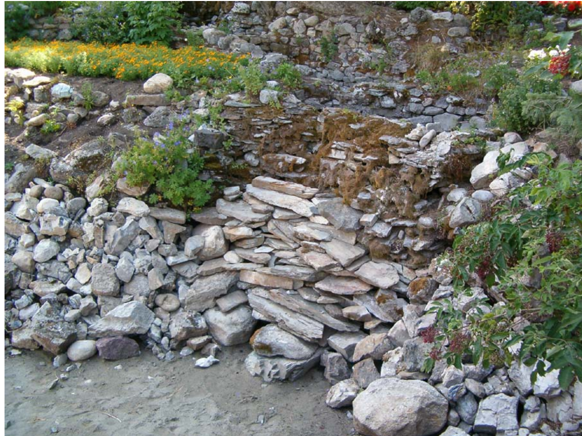
PHOTO #E32 STONES REPLACED AT CASCADE #2
