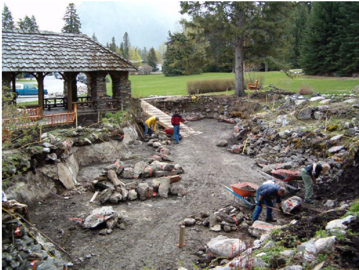
PHOTO #E7 REMOVAL OF STONES IN PROGRESS
