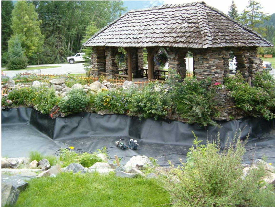
PHOTO #E21 INSTALLATION OF LINER MEMBRANE
