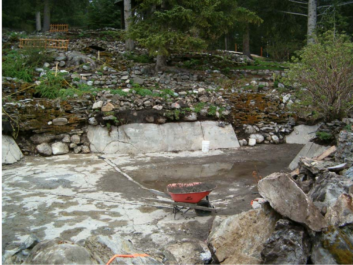
PHOTO #E9 ORIGINAL CONCRETE WALLS AND SLAB EXPOSED
