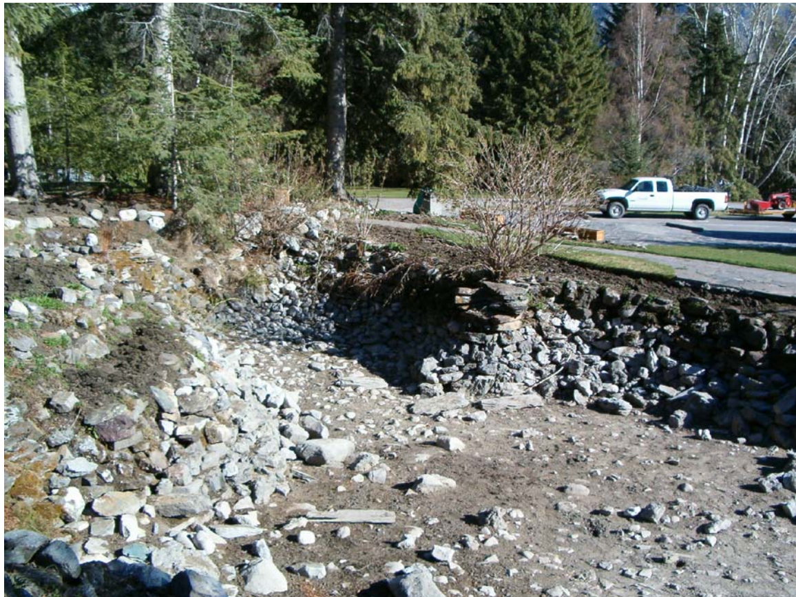
PHOTO #E3 RECORDING PRIOR TO REPAIRS
