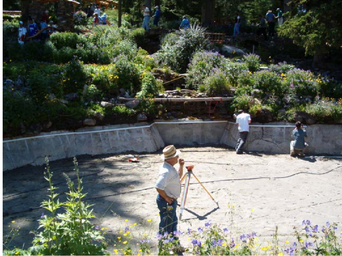
PHOTO #E18 INSTALLATION OF ANCHORS & DRY-FIT OF PLASTIC CLAMPING CHANNEL
