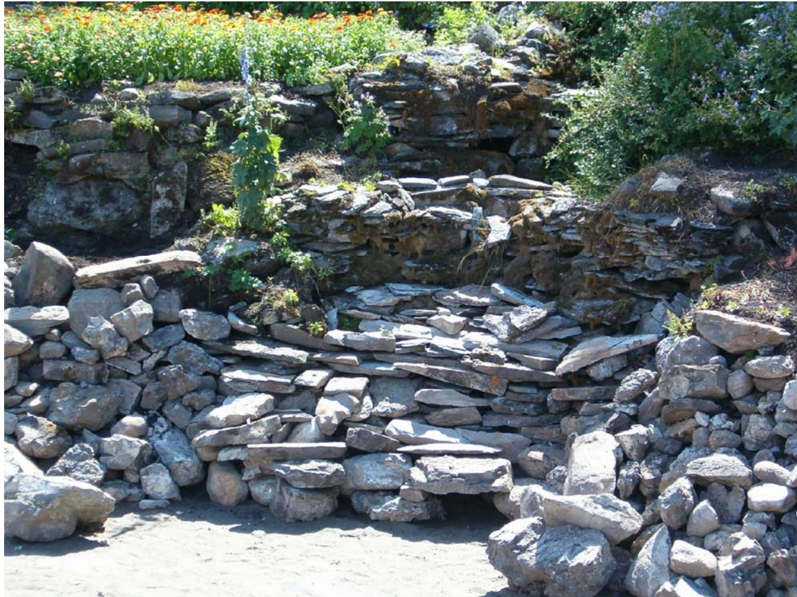
PHOTO #E31 STONES REPLACED AT CASCADE #1
