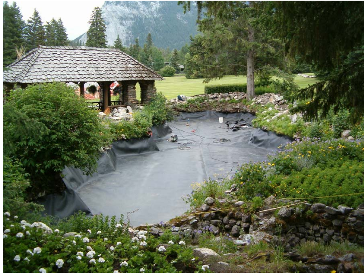
PHOTO #E22 INSTALLATION OF LINER MEMBRANE
