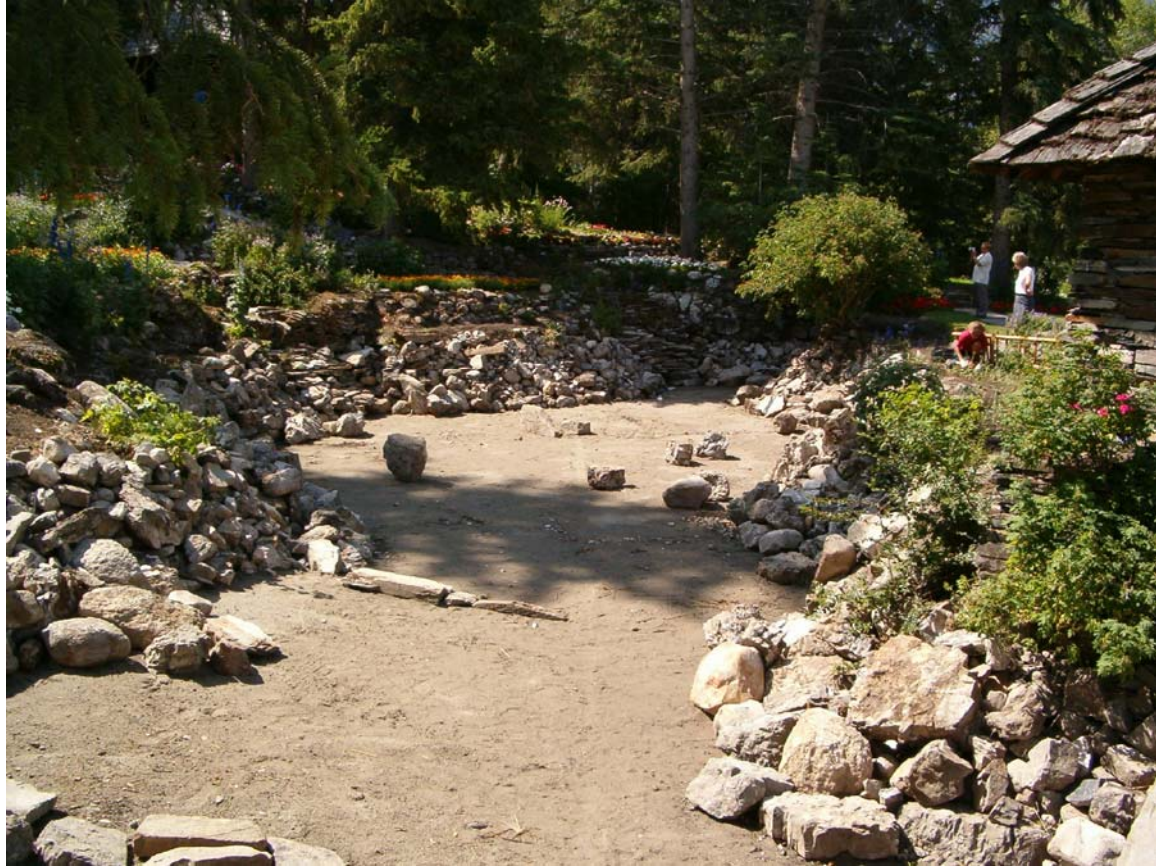
PHOTO #E29 STONES REPLACED IN POOL
