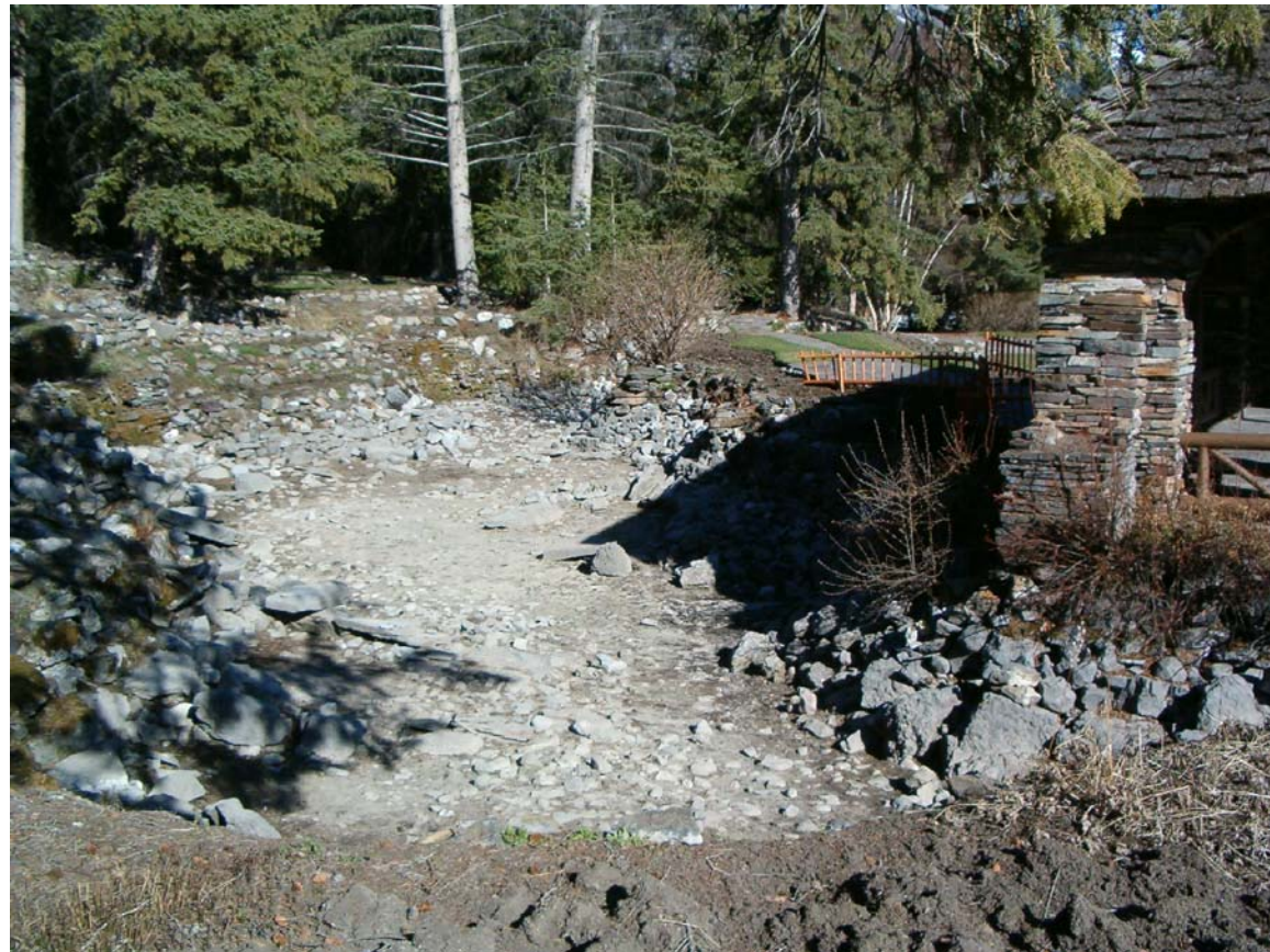
PHOTO #E4 RECORDING PRIOR TO REPAIRS
