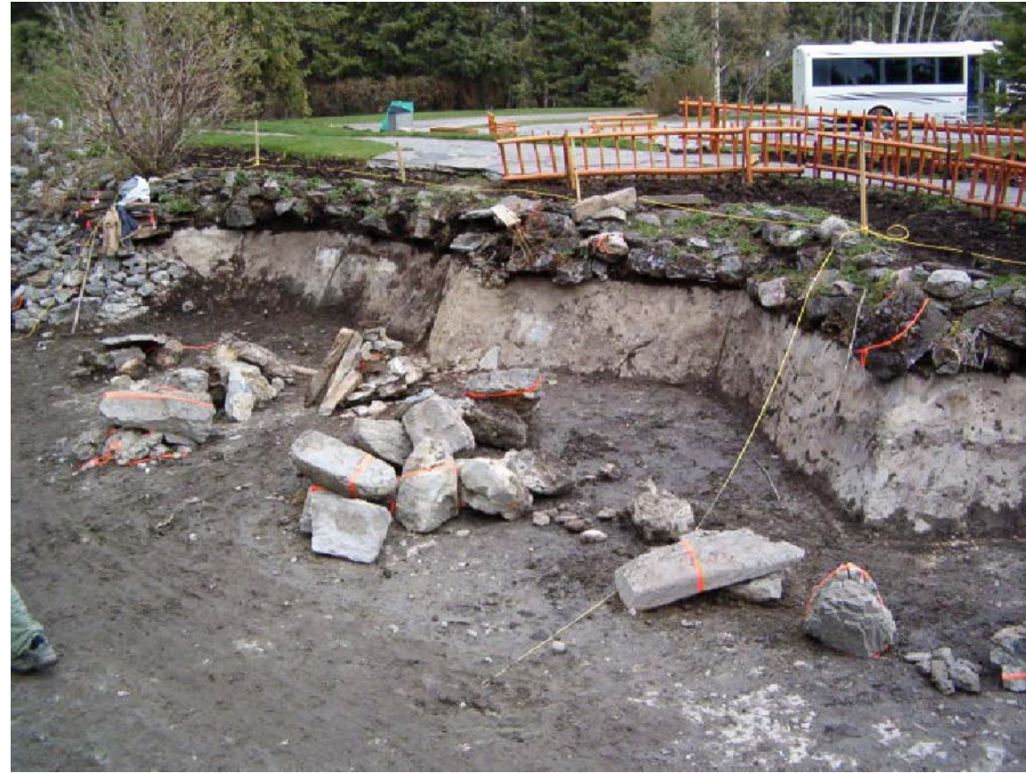
PHOTO #E6 REMOVAL OF STONES IN PROGRESS
