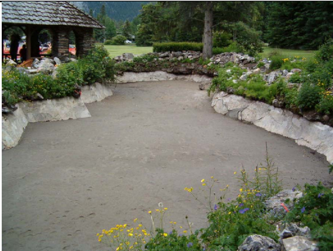
PHOTO #E13 CONC. WALLS REPAIRED & SAND BASE INSTALLED OVER SLAB
