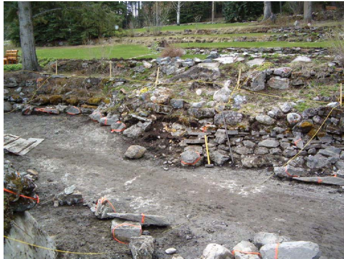
PHOTO #E8 REMOVAL OF STONES IN PROGRESS
