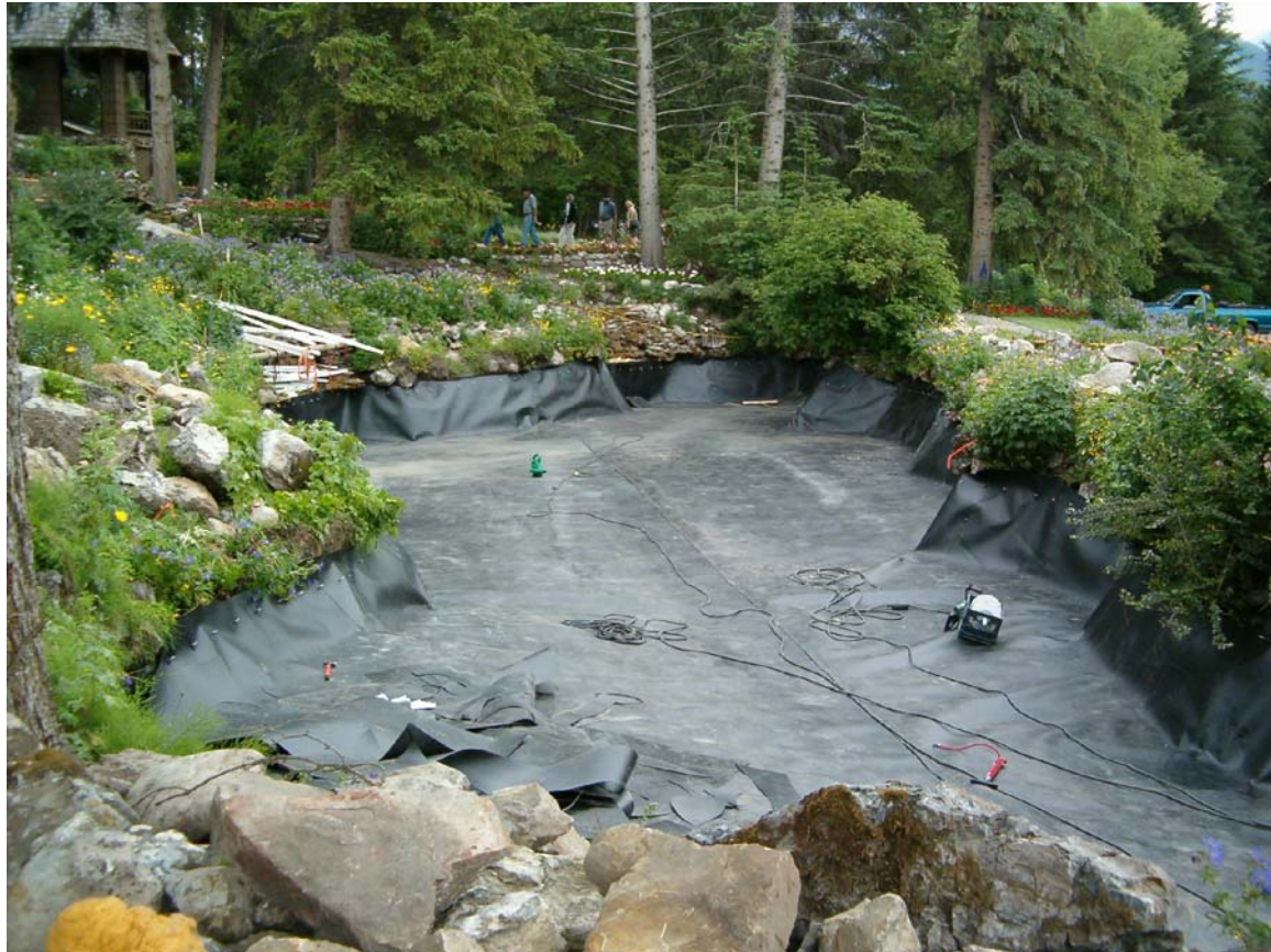
PHOTO #E19 INSTALLATION OF LINER MEMBRANE
