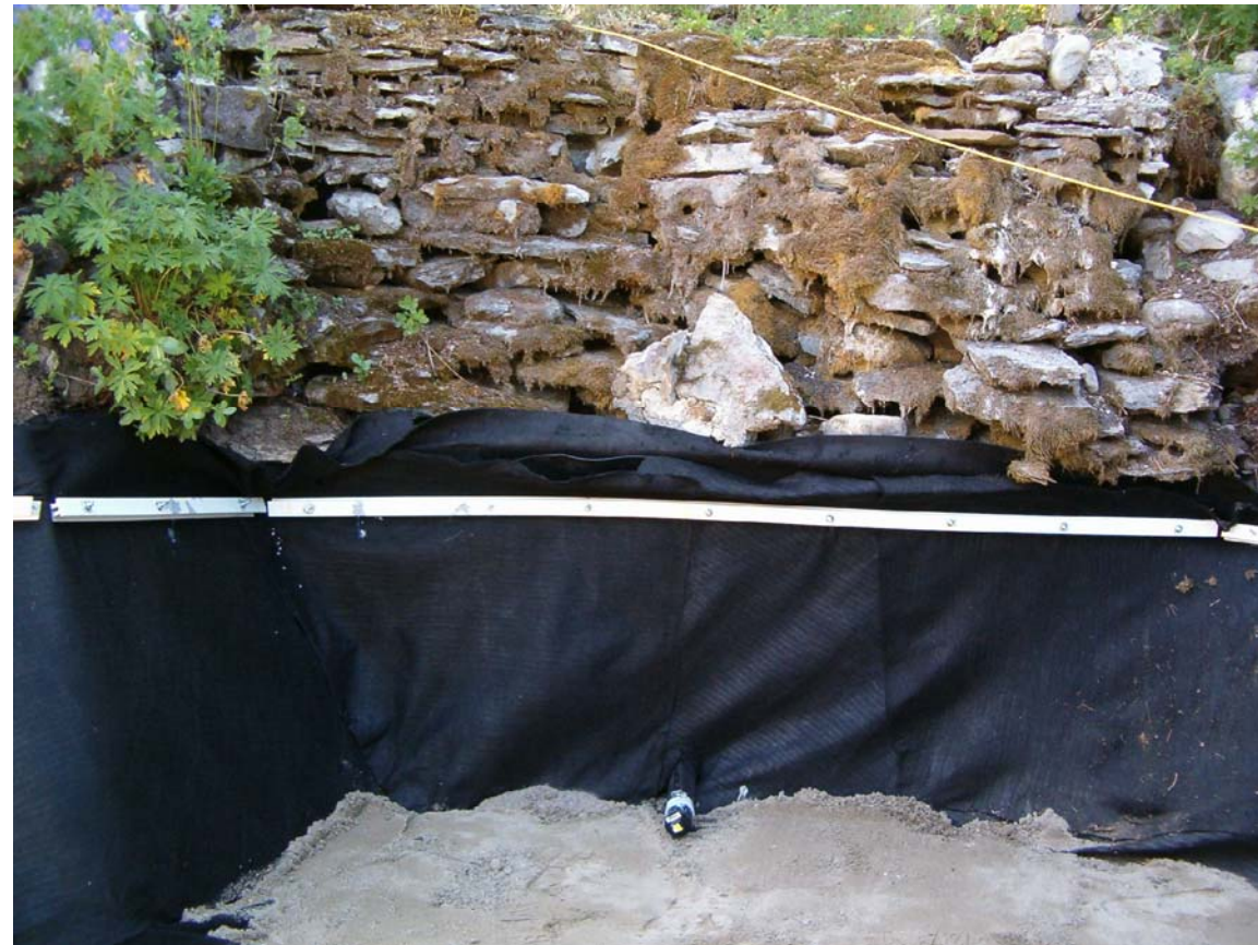
PHOTO #E28 INSTALLATION OF LINER AT CASCADE #2
