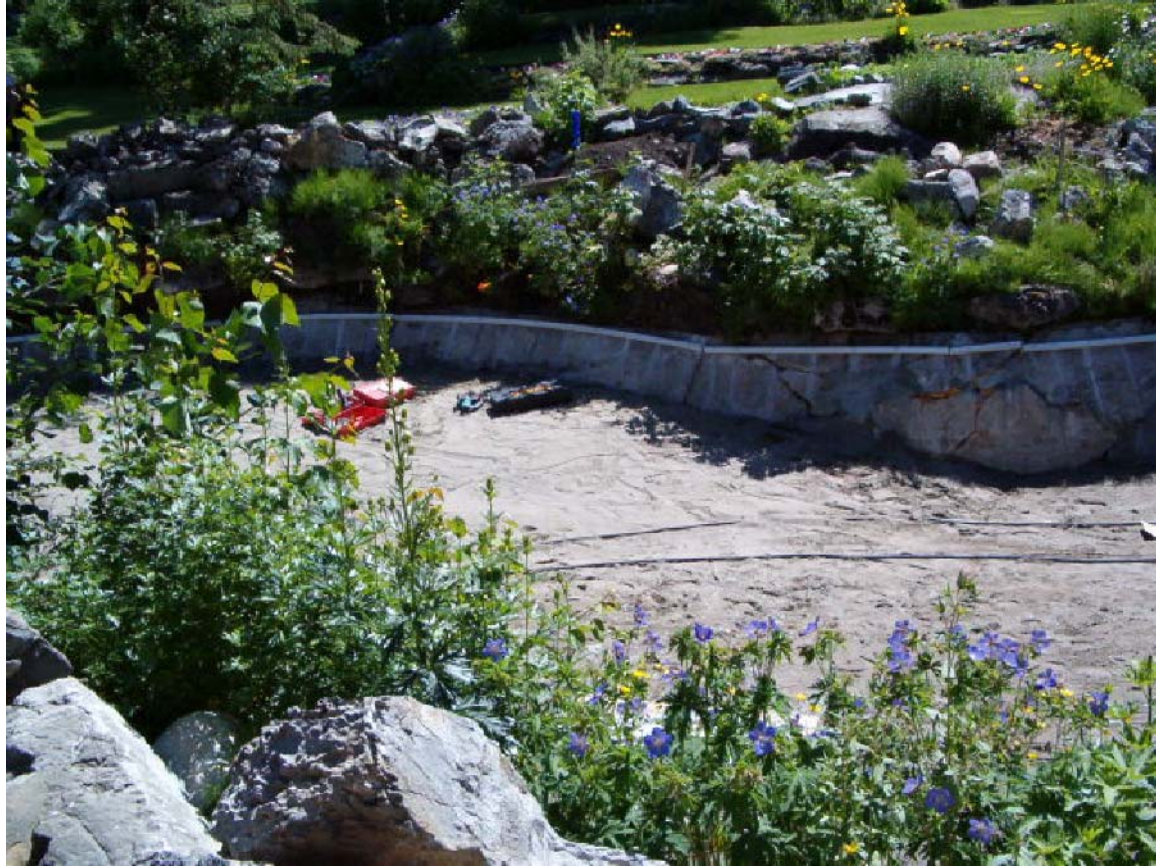
PHOTO #E17 INSTALLATION OF ANCHORS & DRY-FIT OF PLASTIC CLAMPING CHANNEL
