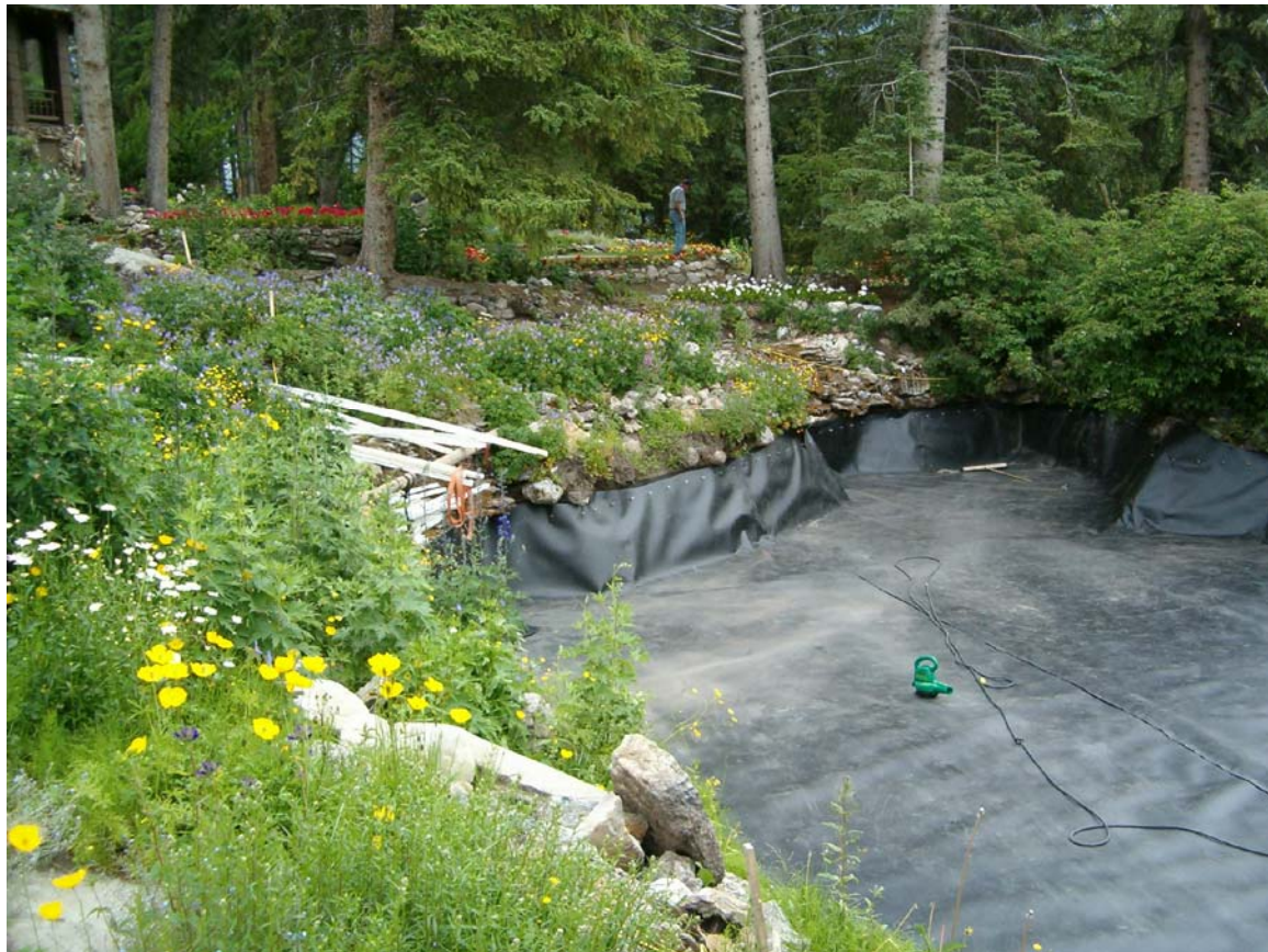
PHOTO #E23 INSTALLATION OF LINER MEMBRANE
