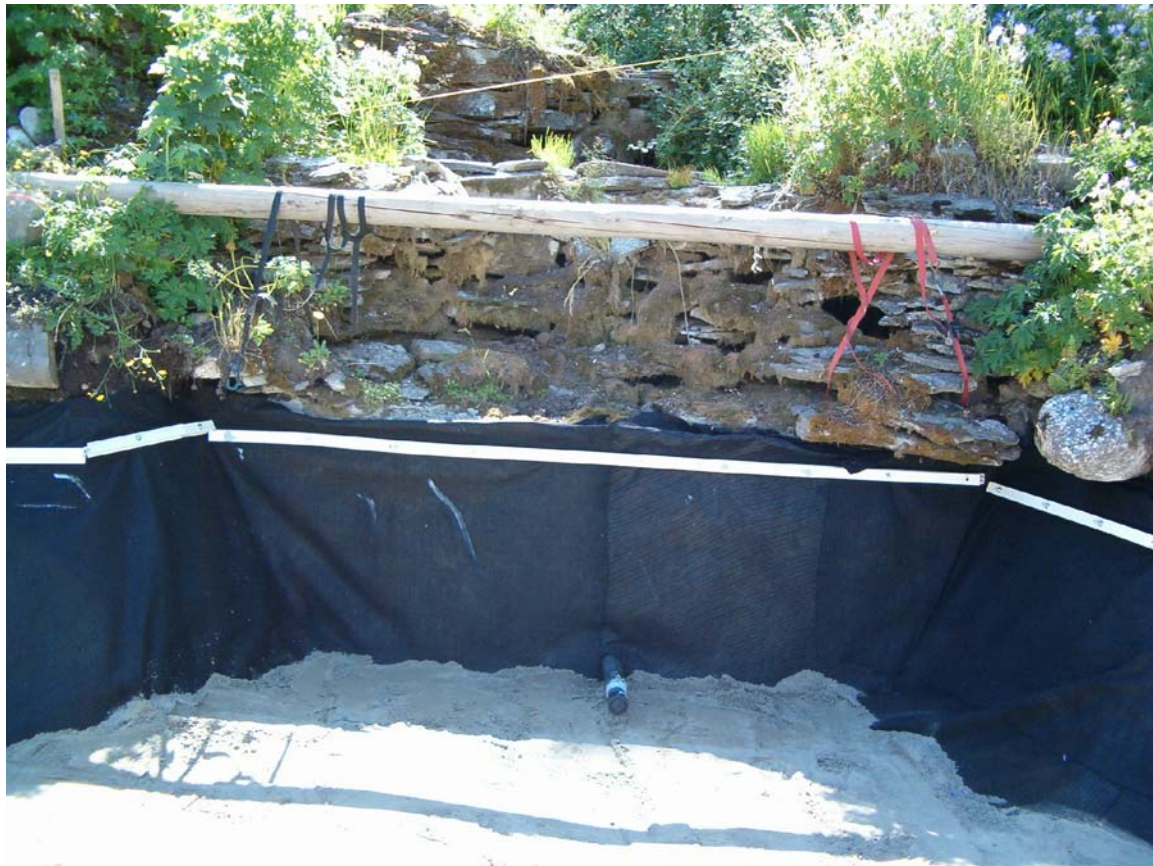
PHOTO #E27 INSTALLATION OF LINER AT CASCADE #1
