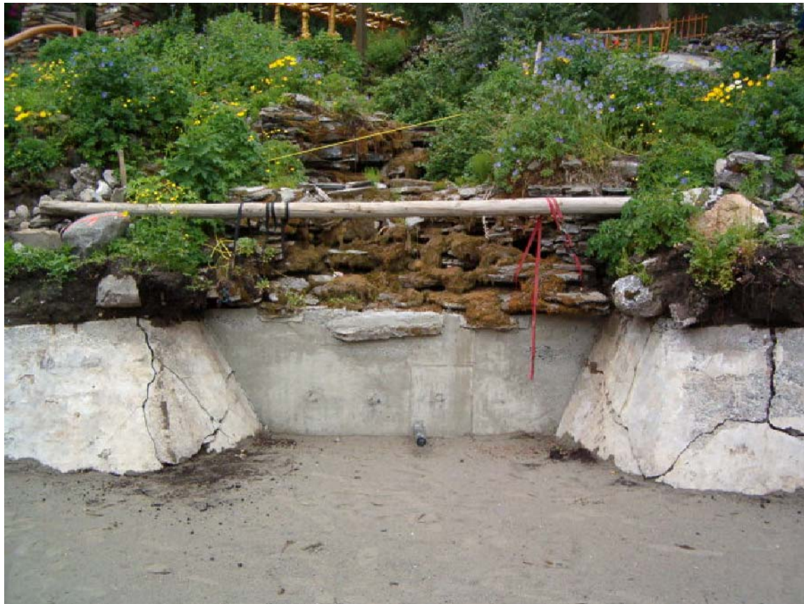
PHOTO #E15 NEW CONCRETE WALL & DRAIN PIPE AT CASCADE#1
