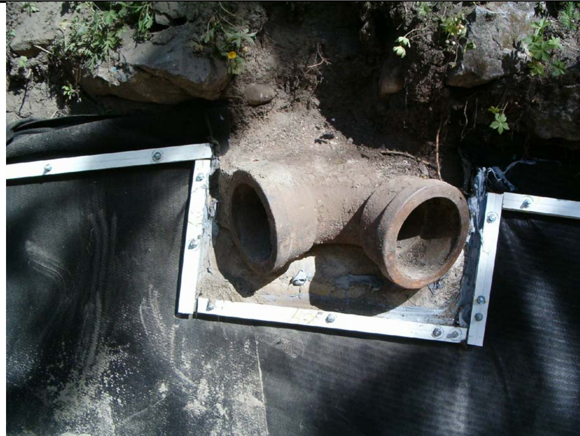
PHOTO #E26 INSTALLATION OF LINER AT OVERFLOW PIPE
