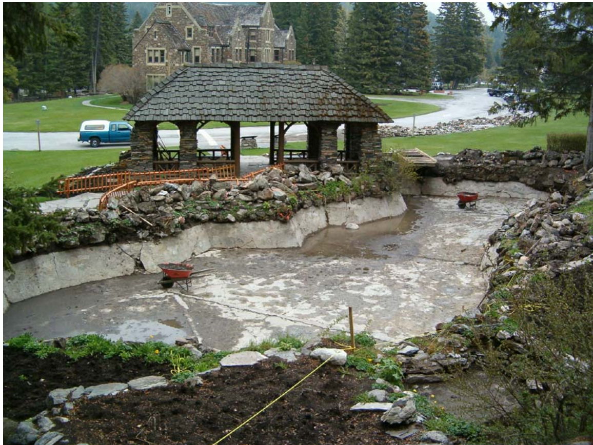
PHOTO #E11 ORIGINAL CONCRETE WALLS AND SLAB EXPOSED
