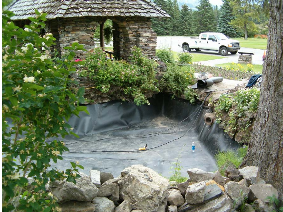
PHOTO #E20 INSTALLATION OF LINER MEMBRANE
