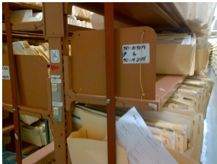
*Figure 1: Vertical bracing bars (A) and metal plates (B).
