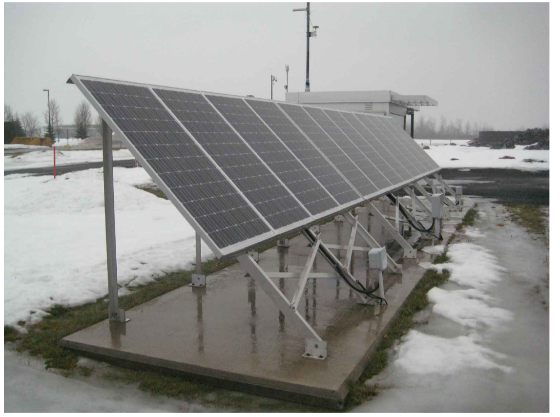
B PANNEAUX PHOTOVOLTAÏQUES PHOTOVOLTAIC CELLS PANELS
