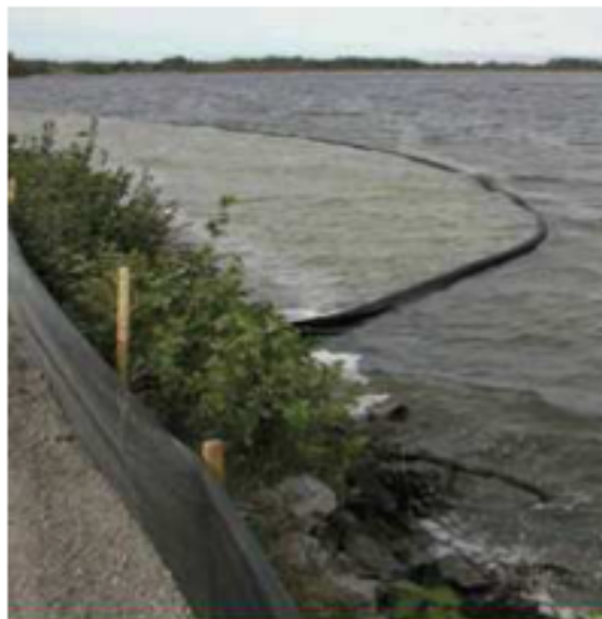
FIGURE 2 An exemple of a turbidity curtain installed in a river.
