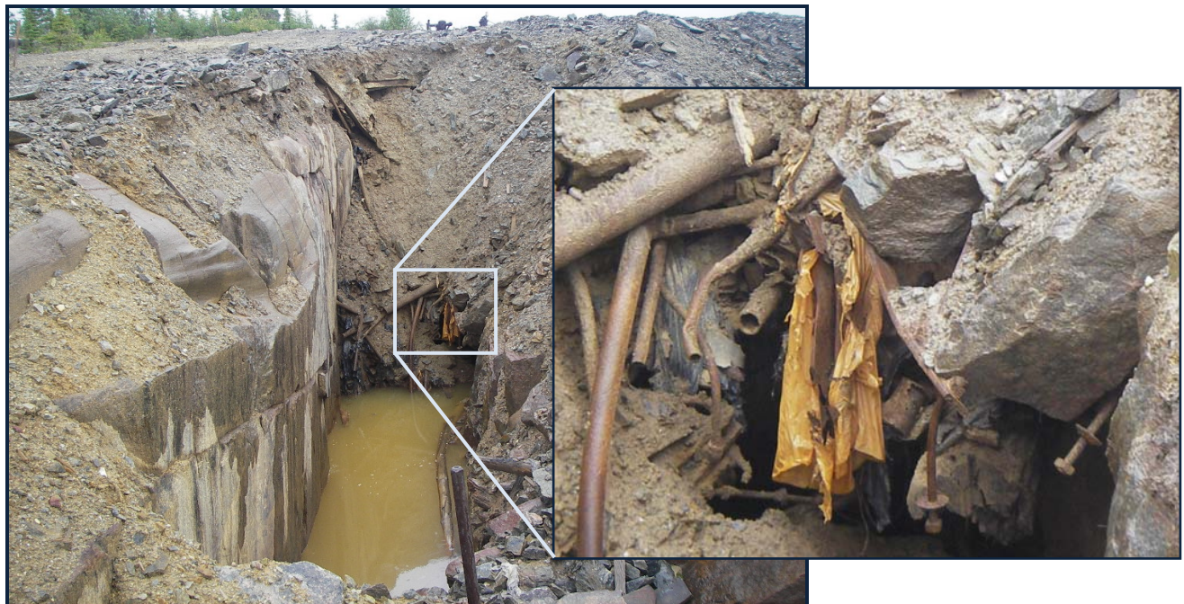
Figure 5. Detail of the rockfilled end of the Open Cut could be evidence of a service tunnel.
