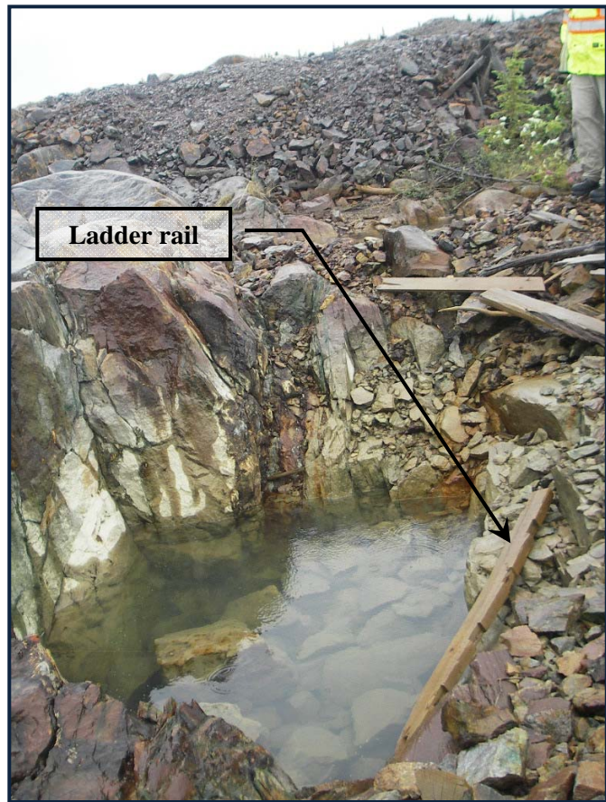
Figure 9. Possible surface breakthrough location of the Stope Raise.
