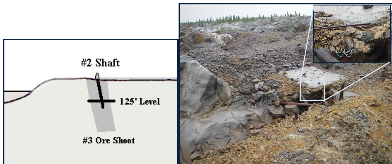
Figure 2. No.2 Shaft Longitudinal View (left); concrete slab over shaft (right).
