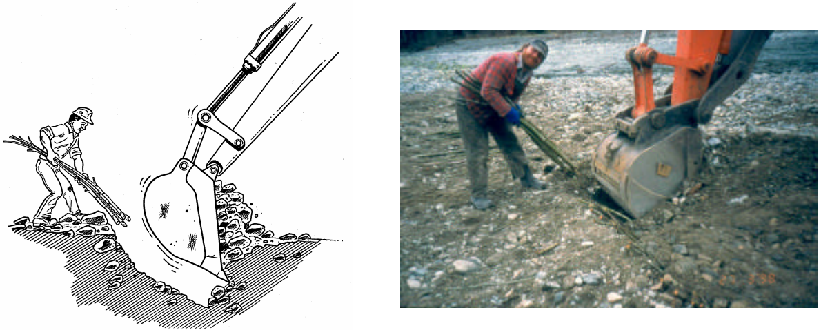
Figure 3.1.7-1(left) & Photograph 3.1.7-1 (right). An excavator can be used for live gravel bar staking. This is a simple method of establishing pioneering woody vegetation on the tops of gravel bars where excess gravel is causing stream instability. It can be effectively used in these cases to establish riparian vegetation along streams and initiate successional advancement. Live gravel bar staking changes the water flow across the bar during high flows, allowing deposition of fine sediment and thus encouraging invasion by other species. The stakes should be inserted at an angle with the tip pointing downstream. This will allow the cutting to offer little resistance during the early years with the new shoots developing to slow the flow (from Polster, 2001).
