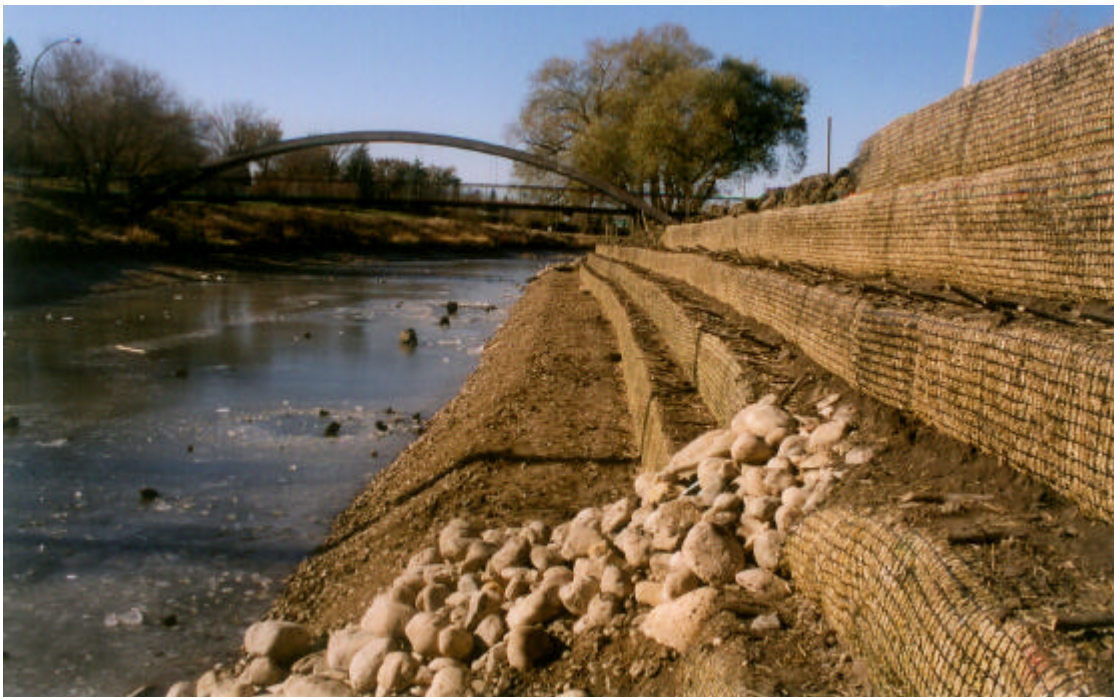
Photograph 3.1.5-1. Brush layers are installed between the layers of plastic soil reinforcement to provide a suitable riparian cover. Cattails and bulrushes were planted on the granular material bench to protect the slope from wave erosion. The riprap is used to armour the slope where a culvert outfall occurs. The normal water level is at the base of the first wrapped lift. This site is on Wascana Creek in Regina, Saskatchewan.
