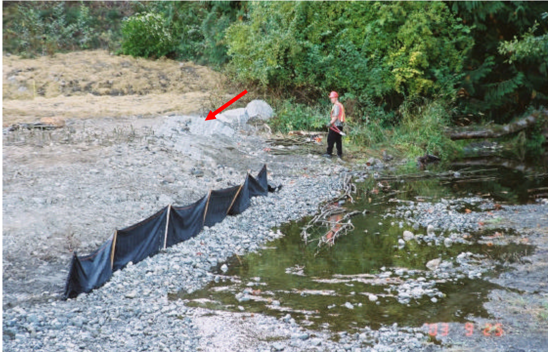
Photograph 2.2-1. Articulating concrete mats (red arrow) are used here to protect the underlying pipeline against erosion. Live cuttings (soaking in stream) are being installed in the holes in the mats.
