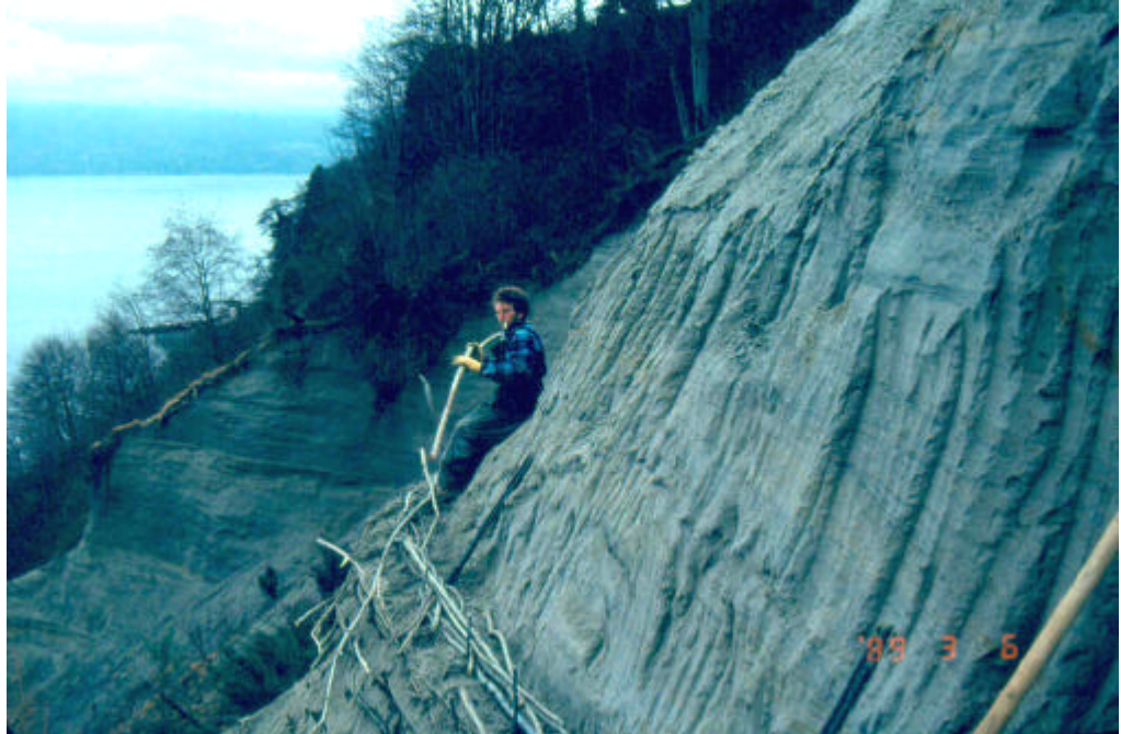
Photograph 3.2.1-1. Wattle fences can be used to treat some steep (70 degree) slopes. These sand cliffs at the University of British Columbia were treated in the late 1980's and are now supporting invading Douglas fir and other forest species. (from Polster, 2001)
