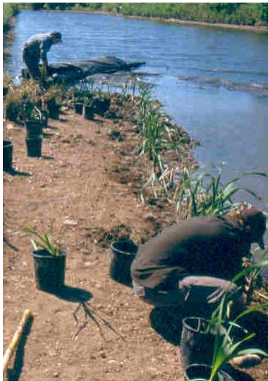
Photographs 3.3.5-1 & 2. Sprigs of emergent aquatic vegetation such as Cattails ( Typha latifolia ) and bulrushes ( Schoenoplectus spp.) can be used to provide erosion protection from relatively slow moving prairie streams and from waves. Planting undertaken in the spring has grown over the summer to fully protect the shore from wave and streambank erosion. Photos taken on Wascana Creek in Regina, Saskatchewan.
