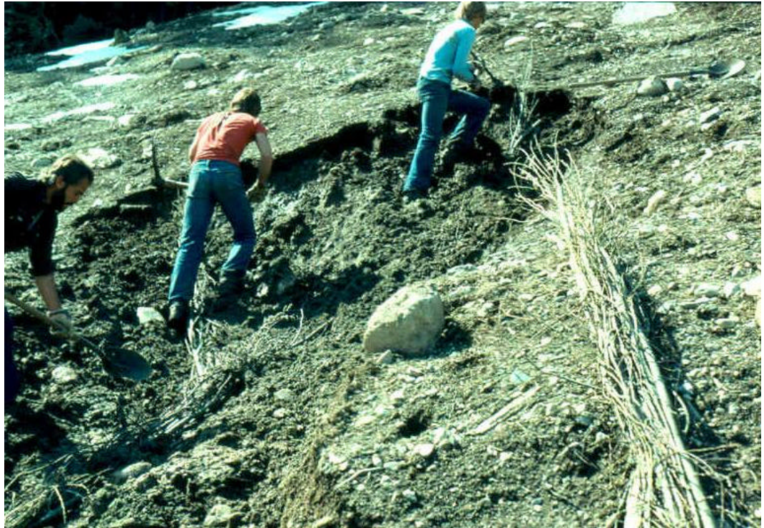
Photograph 3.3.1-3. Live pole drains provide immediate drainage of “soupy” soils. Bundles of willow are inserted and act as a preferred flow path for subsurface flows, moving the water through sensitive soils.
