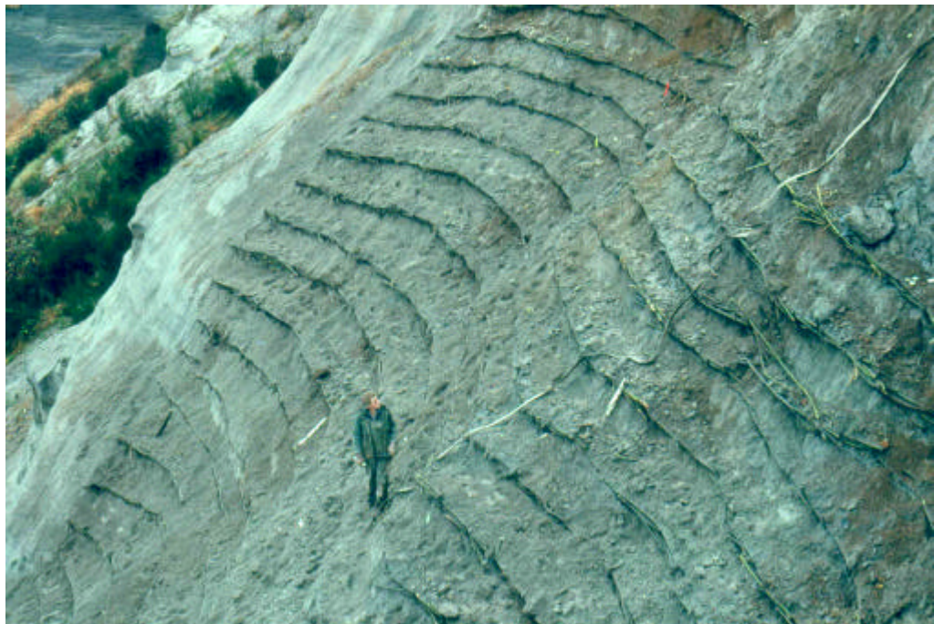
Photograph 3.2.1-2. The wattle fences do not change the actual slope (see background), but change the characteristics of the slope surface relative to plant growth. By preventing material movement on the slope, the wattle fences allow vegetation to be established (from Polster, 2001).
