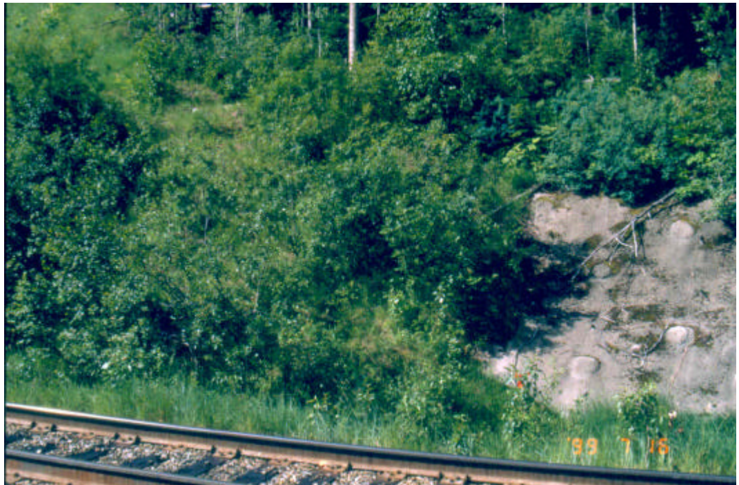
Photograph 3.3.1-2. A dense copse of willows has established after about 12 years. The hard engineering solution, to extend the tied back shotcrete wall (right) would have cost several orders of magnitude more than the bioengineering.
