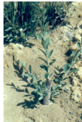
Figure 3.1.6-1 (left) & Photograph 3.1.6-1 (right). Live staking is a simple method of establishing pioneering woody vegetation. It can be effectively used on "flowing" silts and to establish riparian vegetation along streams. Most (3/4 to 7/8) of the cutting should be underground to establish a balance between root and shoot growth (from Polster, 2001).
