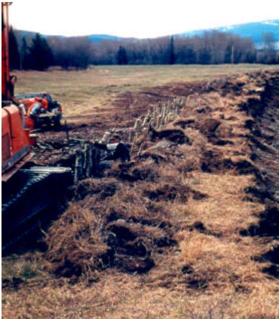
Figures 3.2.5-1 & 2 and Photographs 3.2.5-1 & 2. Live palisades can be used to provide a row of dense root systems to hold eroding banks in place. Cross section of live palisades (right). Note that the large posts must extend to the water level. Photographs (below) of live palisades installed along the Bulkley River (photos by Greg Tamblyn) (modified from Polster, 2001)
