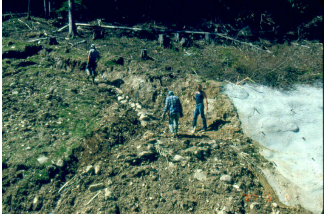
Photograph 3.3.1-1. Live pole drains were installed in the scarp to control movement of the large block of soil (on left). The soil was so wet rocks were needed to hold down the drain.
