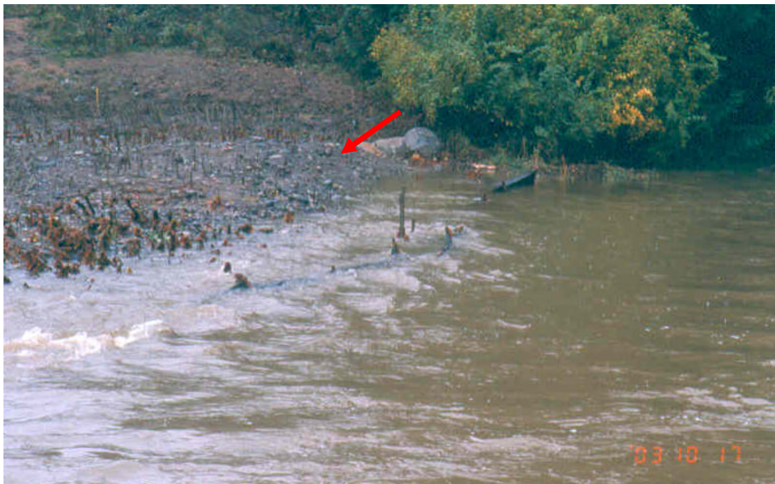
Photograph 2.2-2. The same site shown in Photograph 2.2-1 is seen here during high flows. The concrete mat (as well as the live gravel bar staking) was effective in holding the bank in place and protecting the newly planted cuttings from erosion.
