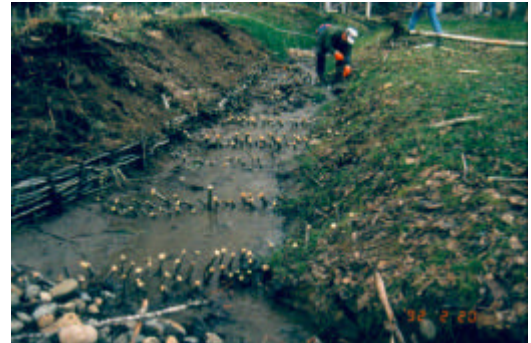
Figure 3.3.4-1 and Photograph 3.3.4-1. Live silt fences can be used to provide a willow coppice in smaller, slow moving streams and ditches. They act by slowing the velocity of the water and allowing sediments to settle out. The cuttings can be either in single rows (as shown) or multiple rows in each band (as shown in the photo above). Note the use of live bank protection on the right bank (from Polster, 2001).
