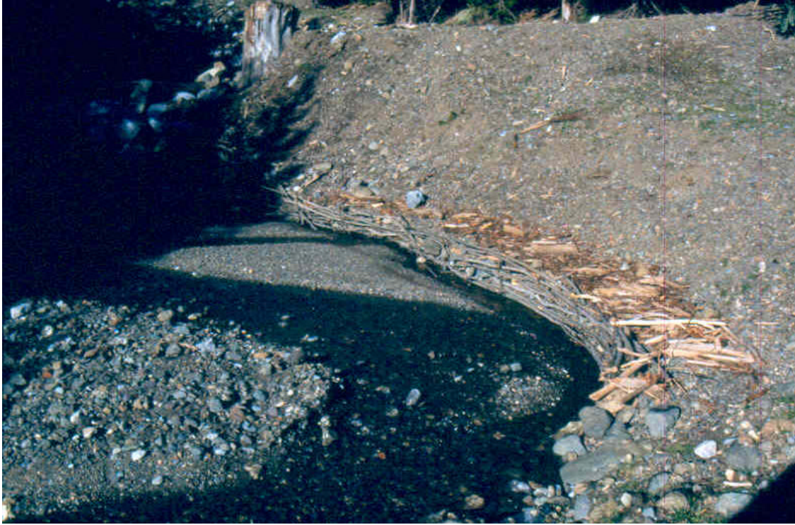
Photograph 5.3.2-1. Live bank protection is used to prevent erosion of bank sediments. The small woody debris collected on the top of the bench formed by the live bank protection after high winter flows. No stream velocity information is given (from Polster, 2001).
