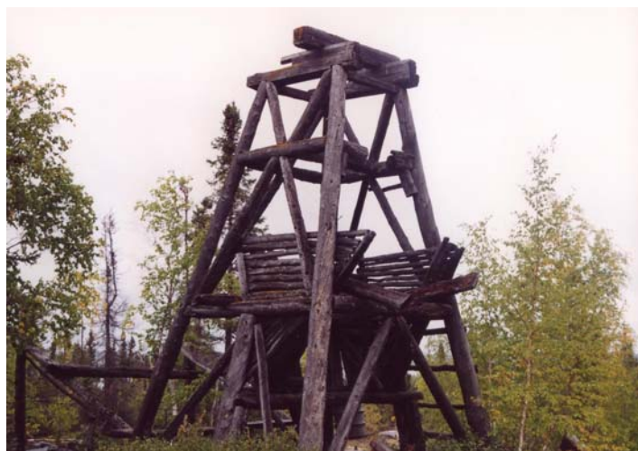
Figure 1. Burnt Island Mine old headframe, 2001.
