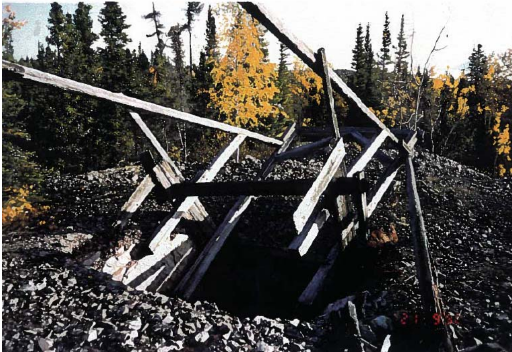
Collapsed headframe at shaft
