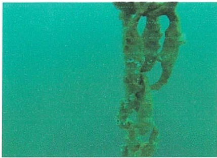
West buoy anchor chain at Shuttle Island. Shows totally unserviceable chain
