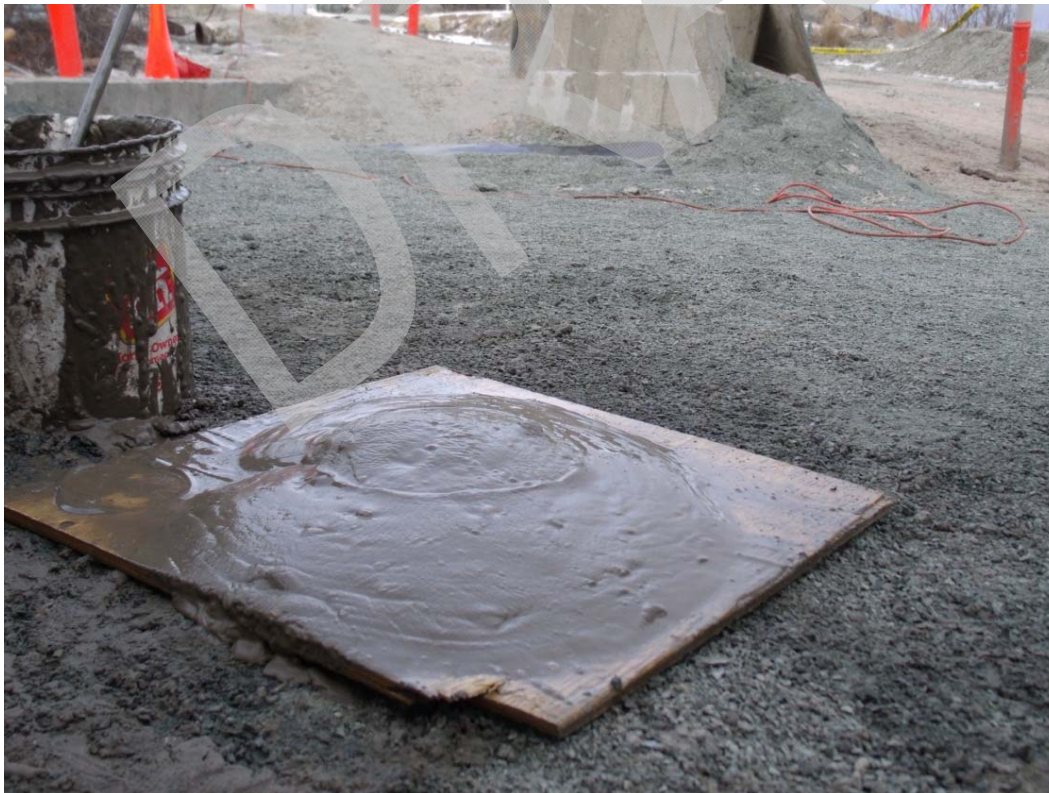
Photograph 9: 250 mm (10") slump paste with 2% (by weight) Normal Portland Cement binder
