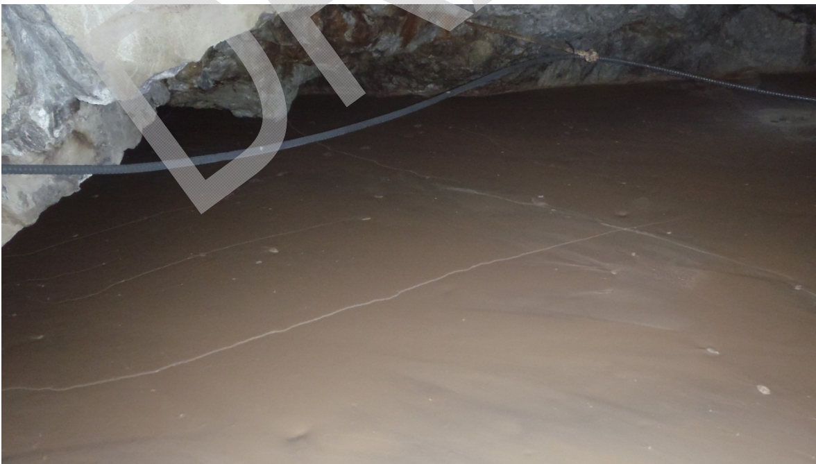
Photograph 12: Flat paste profile in B1-18 EB void below B1 pit sinkhole
