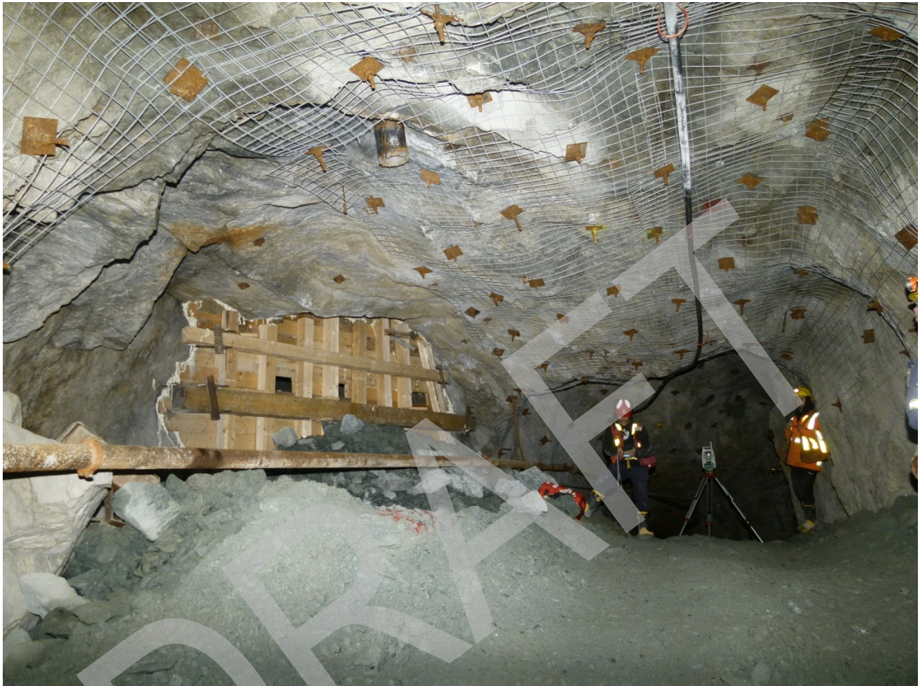
Photograph 3: Constructed fill fence (barricade 1) showing ports for paste spillage prior to backfilling
