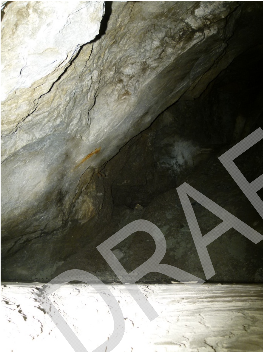
Photograph 5: Paste behind barricade 2 (taken through ports) showing flat paste profile
