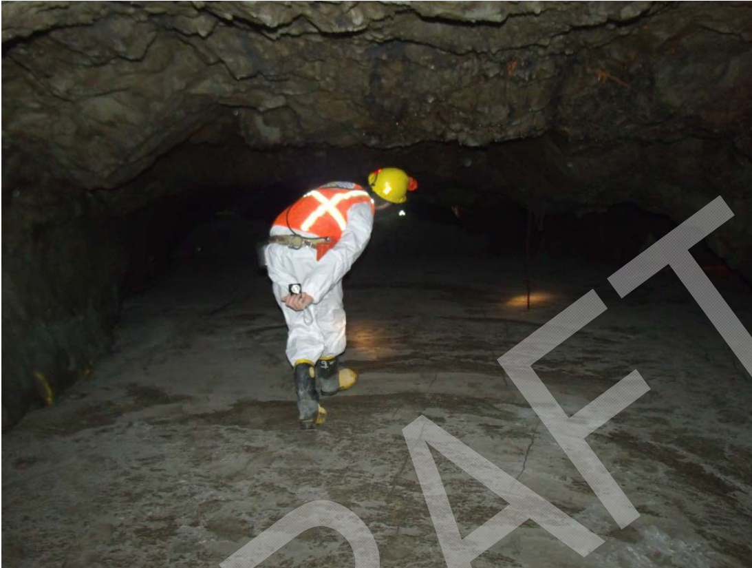
Photograph 11: Flat paste profile in the North extension of the B1-18 Upper North stope
