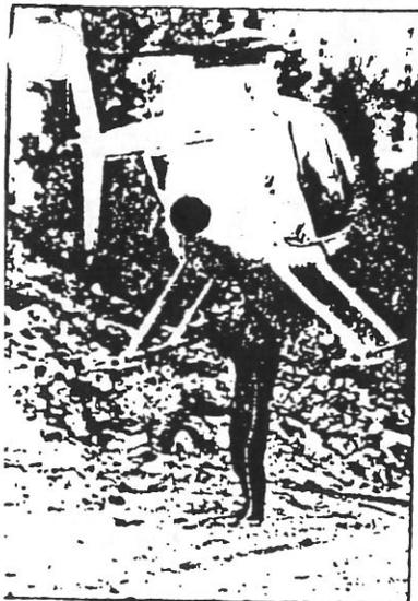
Cable is attached to the bottom of a helicopter to lift drums out of mine site.
