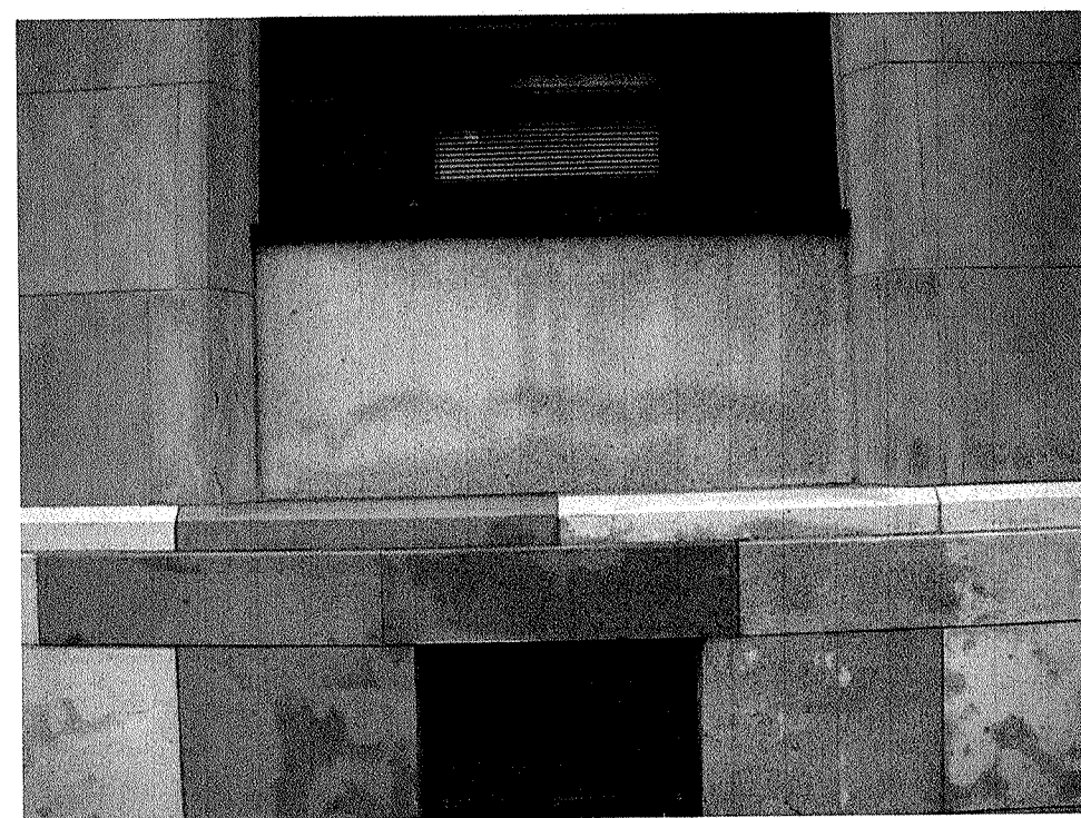
1 STONE UNITS TO BE REMOVED FOR TEST OPENING
