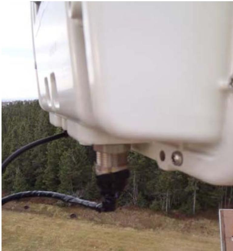
Photo 9 – Poor Tx-line connector weather-proofing
