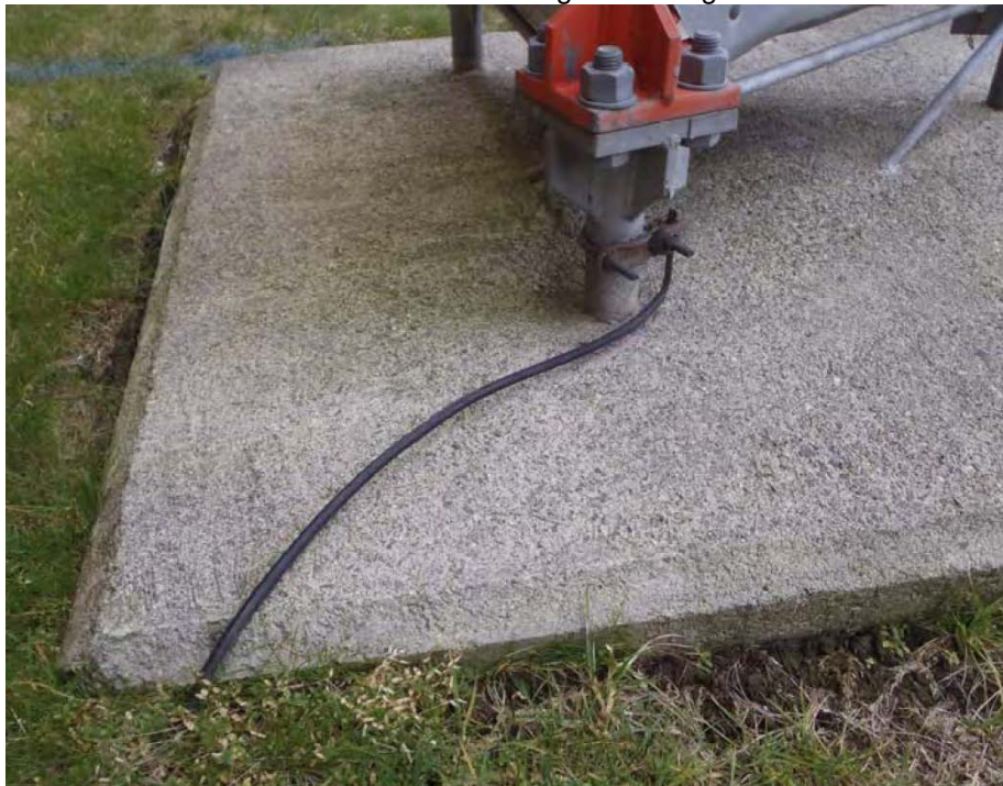
Photo 3 – Tower Leg Grounding
