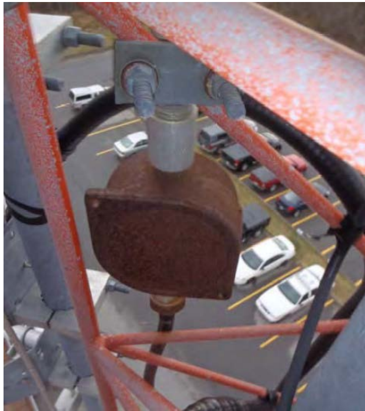
Photo 11 – Tx-line crossing ladder face
