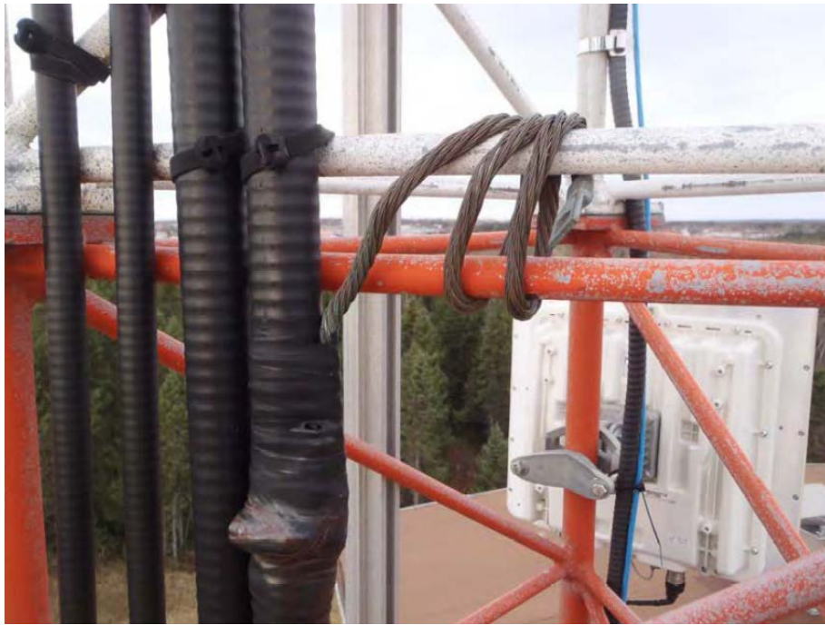
Photo 9 – Poor Tx-line connector weather-proofing
