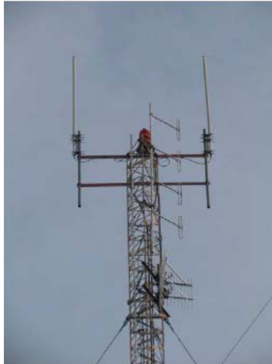
8 Antenna Configuration taken from anchor 3
