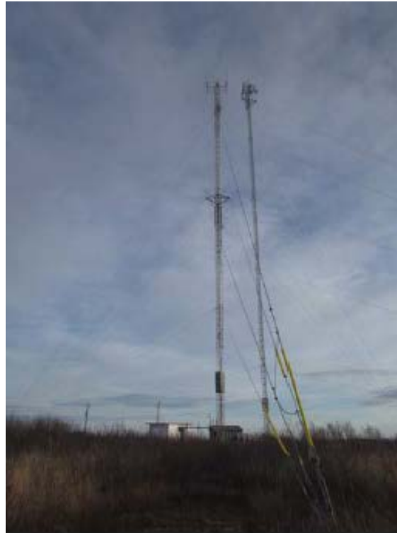
7 Tower Profile as seen from anchor 3
