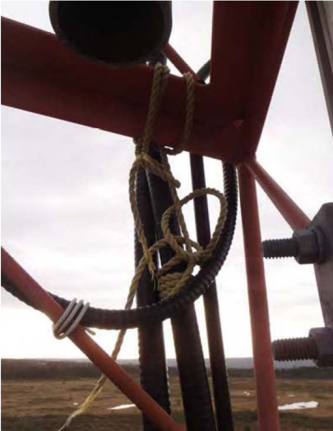
Photo 7 – Rope used for hoisting grips
